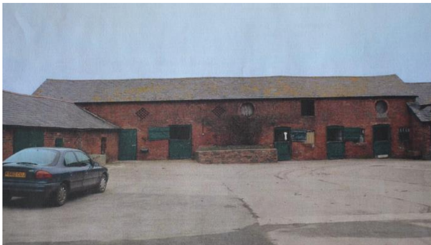
Pl.5: Late-20 th century view of the North Range or Stables, with the West Range to the left.
