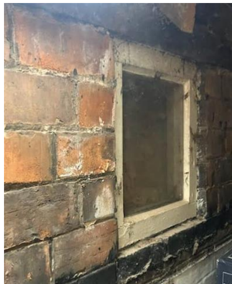
Pls.2-5: The three windows beneath the eaves of the 'stem' of the 'T' facing towards the farmyard.
