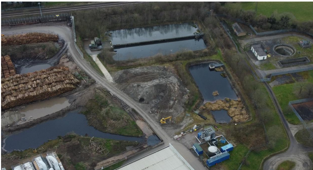
16.03.2022 – Pile spoil stored on site
