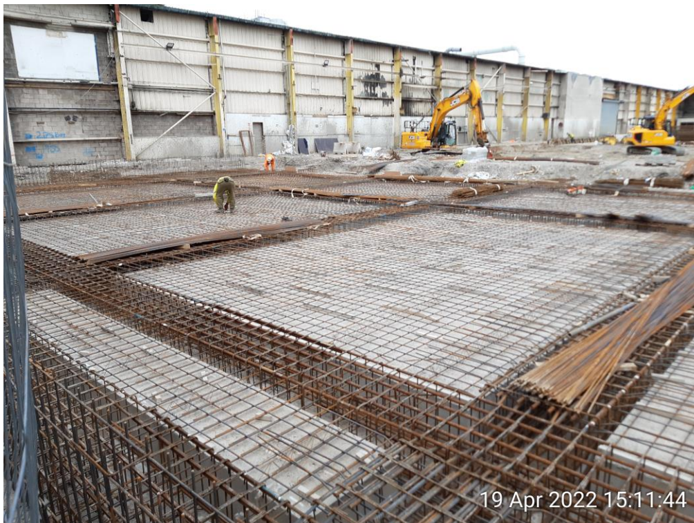
19.04.2022 – Ground beam and slab rebar
