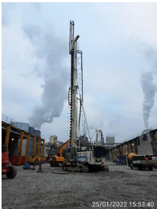
25.01.2022 – Piling rig set up
