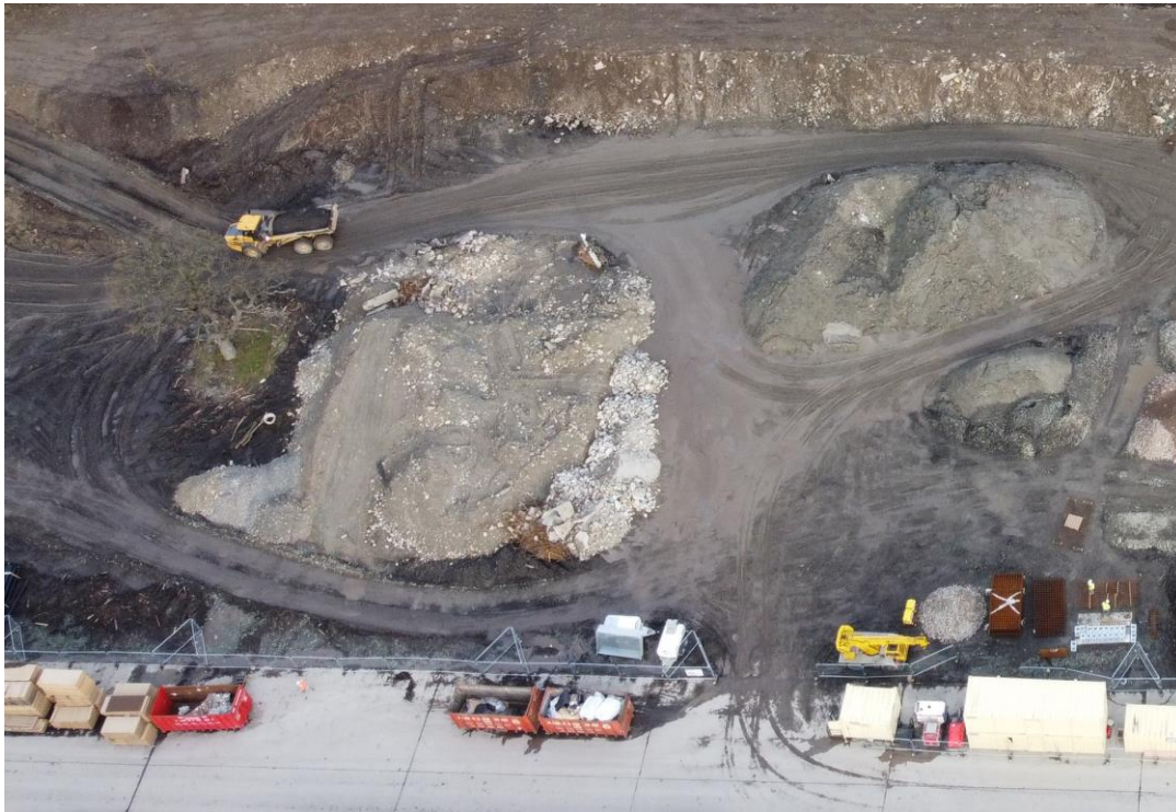
25.03.2022 – Broken out concrete slab and piling mat stored on site
