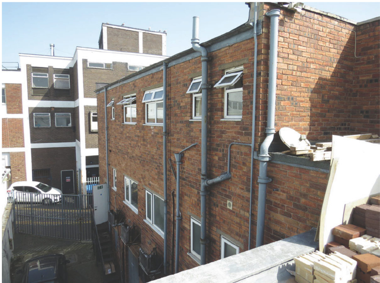
2 – The rear of the building and yard from the roof.
