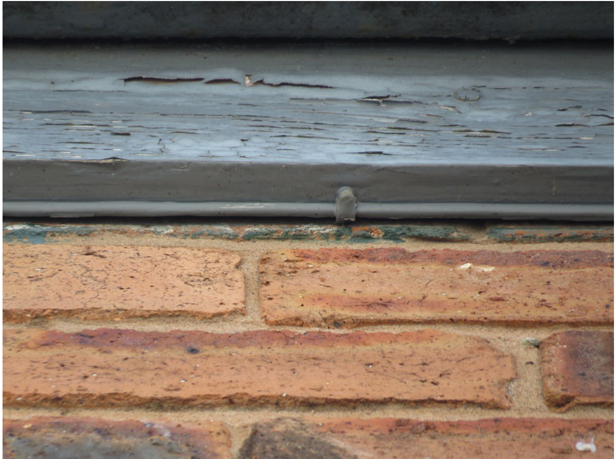
3 – Fascia boards at the rear are in good condition with no suitable gaps.
