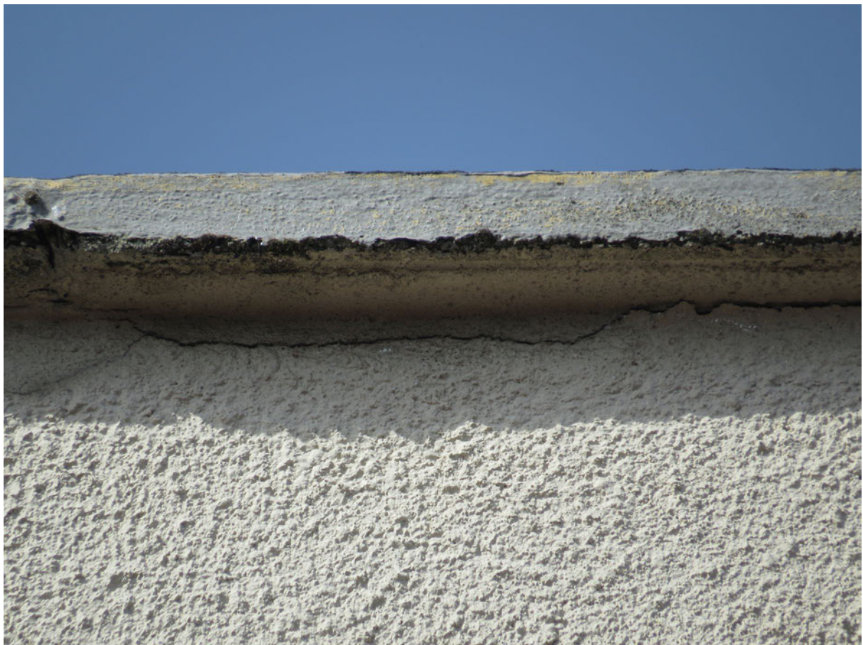
4 – Parapet walls are sealed with coping stones with no gaps between materials.
