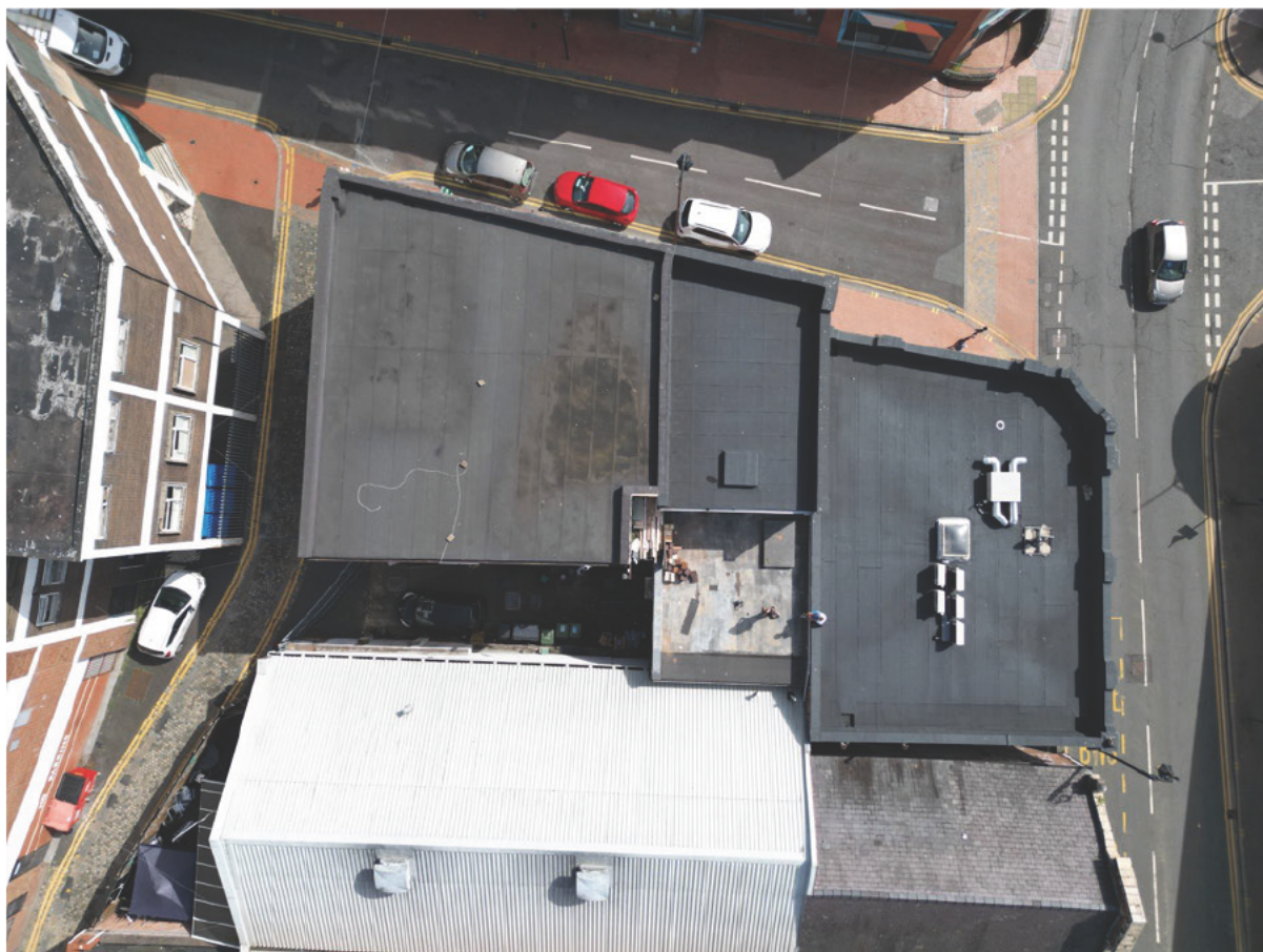
10 – The roof is in good condition with no gaps between materials.
