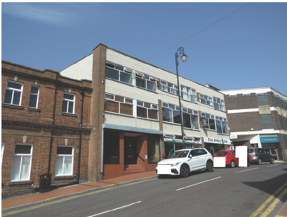
9 – The building is in a busy town centre location.
