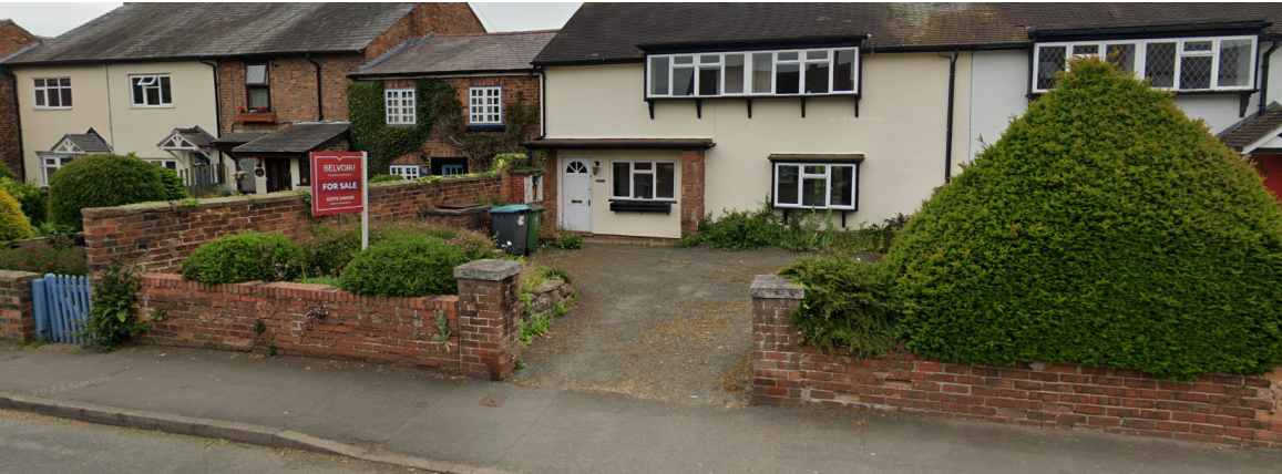
Image of Demolished Front Boundary Wall
