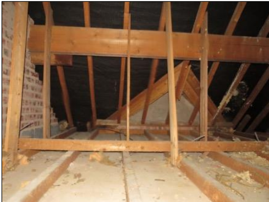
Photograph 2: An internal view of the main roof space.
