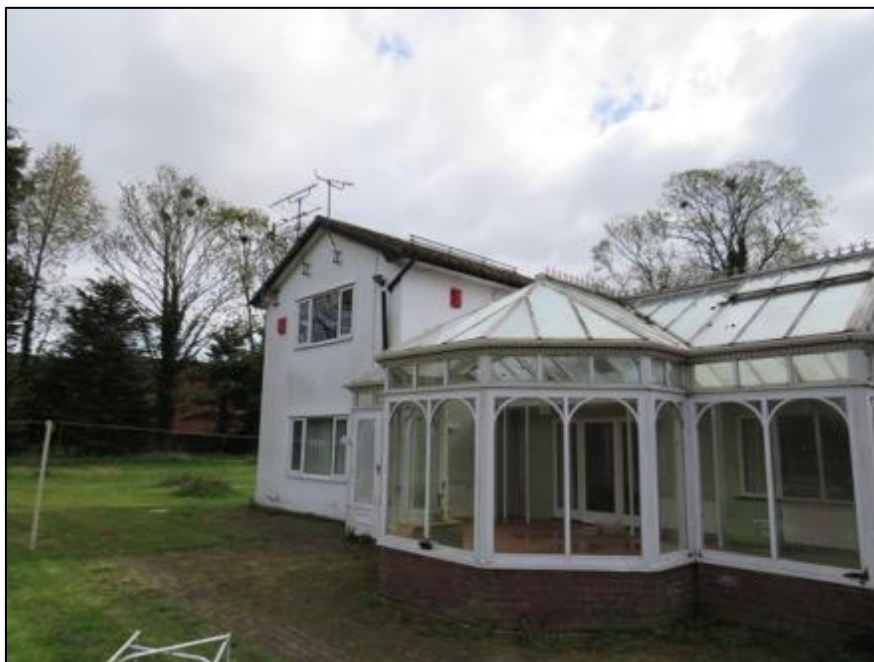
Photograph 4: The rear view of the dwelling showing the conservatory.
