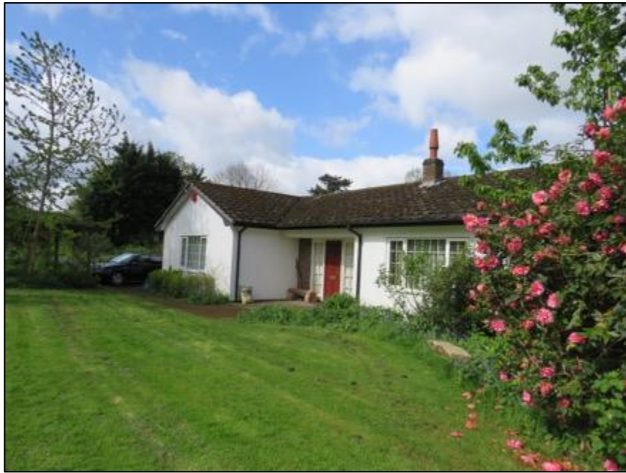
Photograph 1: A front view of the building.
