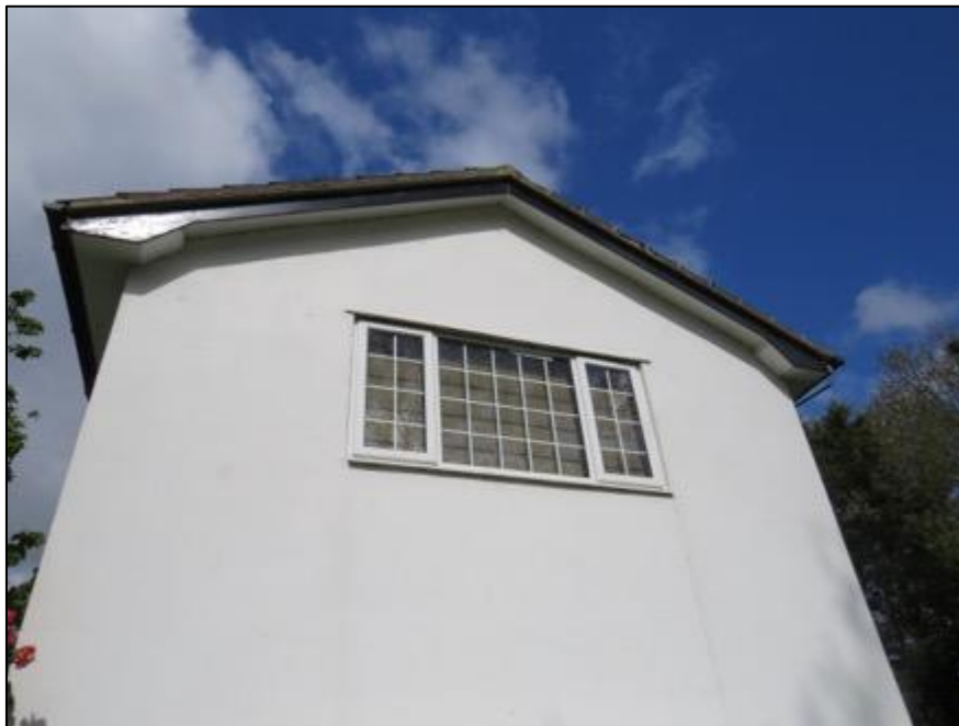
Photograph 3: An external view of the main house the facias are all well sealed.
