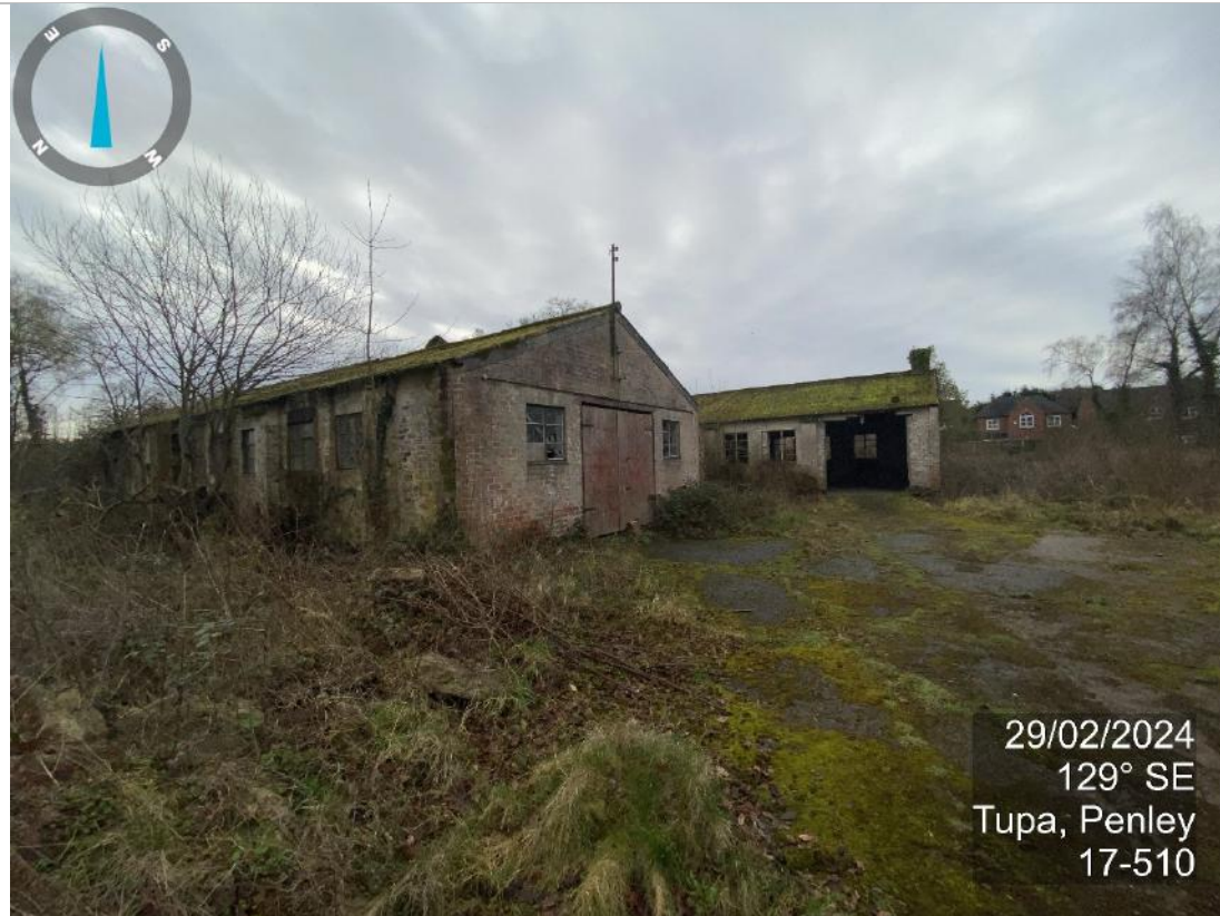
PLATE 1 VIEW OF FORMER HOSPITA BUILDING FACING SOUTH-EAST
