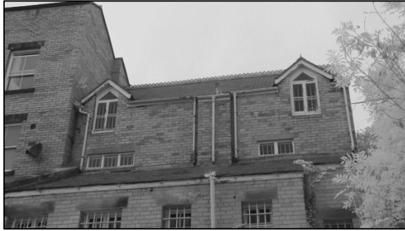
Figure 18: Camera C2 at the start of the survey.
