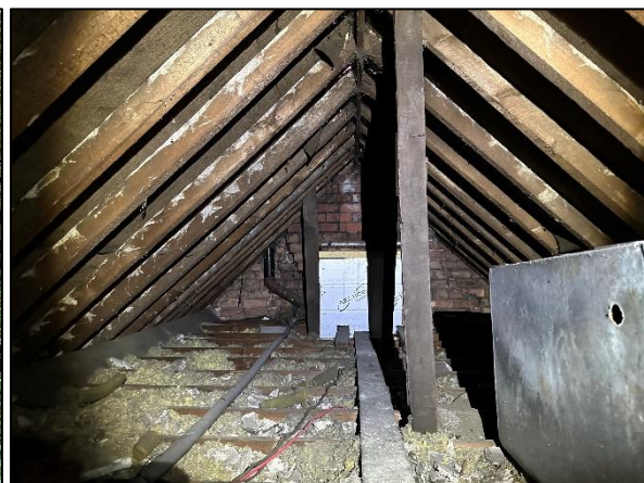
Figure 4: The loft space of the building.
