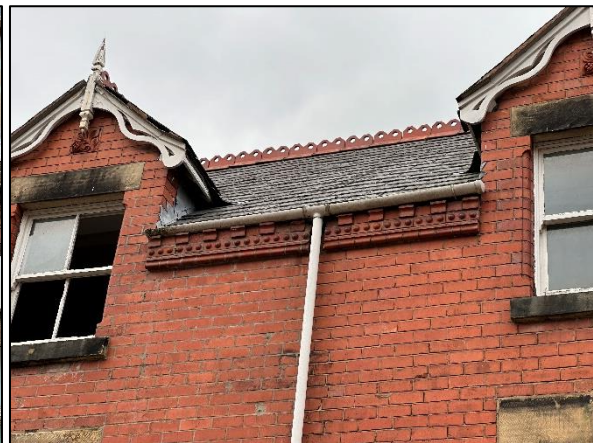
Figure 7: Decorative brickwork at the eaves to the west.
