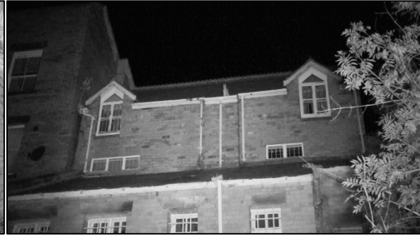
Figure 19: Camera C2 at the end of the survey.
