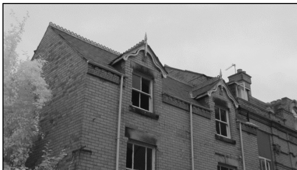
Figure 16: Camera C1 at the start of the survey.
