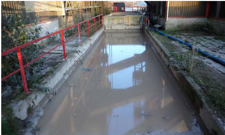
The water-filled tanks at Target Note 20 .
