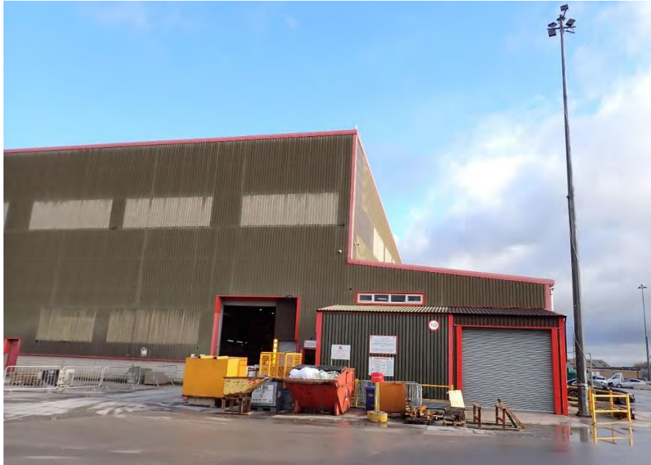
Part of the western elevation of the main CCP building ( Target Note 12 ). One of the flood-light stanchions is on the right.
