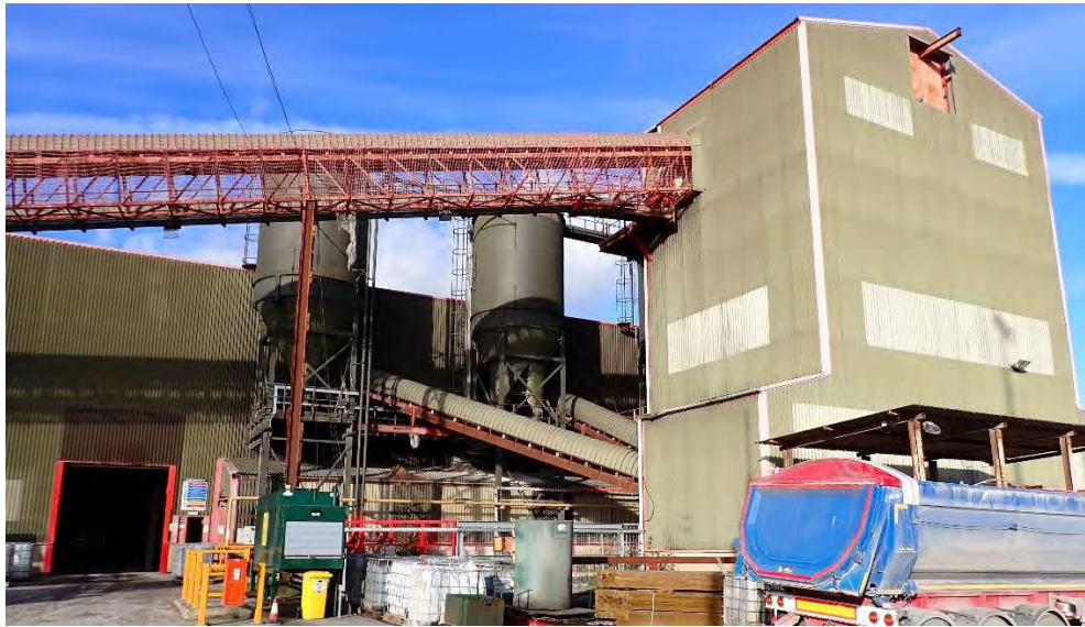
Part of the building at Target Note 14 .
