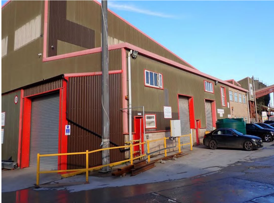
The southern elevation of the main building (Target Note 12).
