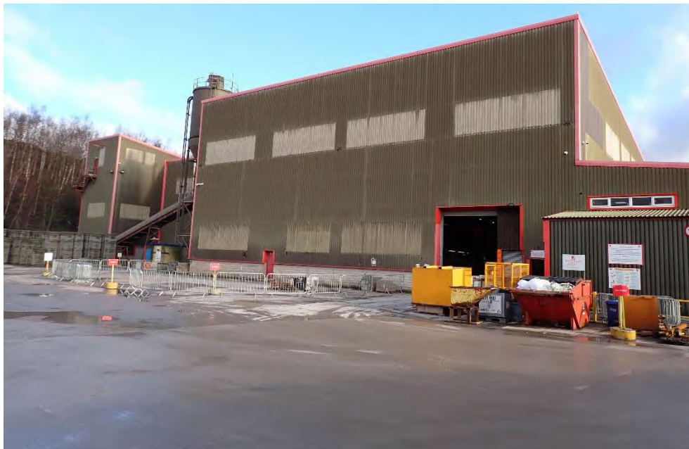
The western elevation of the main building (Target Note 12).
