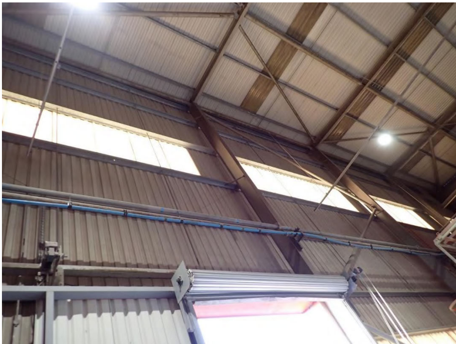
Part of the CCP building interior near the western elevation, showing the roof structure.
