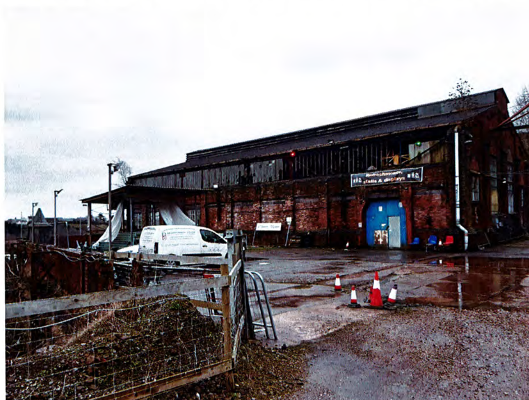
Photograph 4 Main building at front of site
