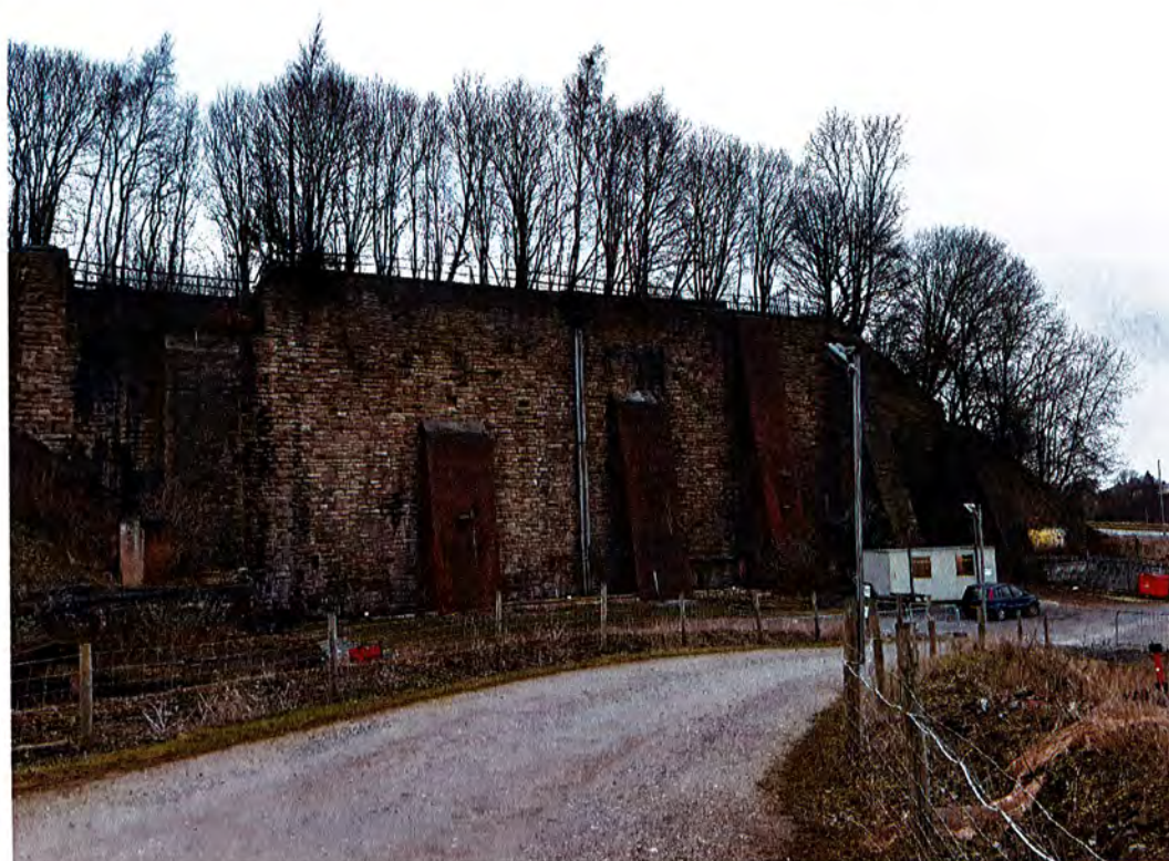
Photograph 6 Retaining structure on northern site boundary
