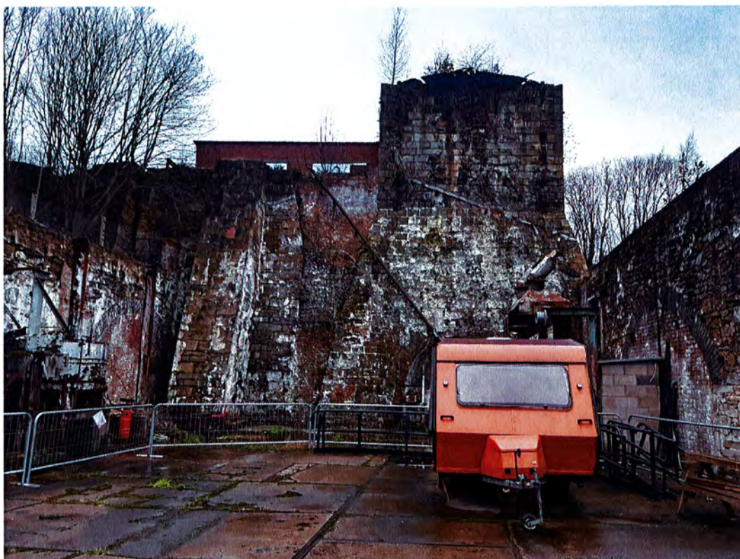
Photograph 9 Steel works structures on site
