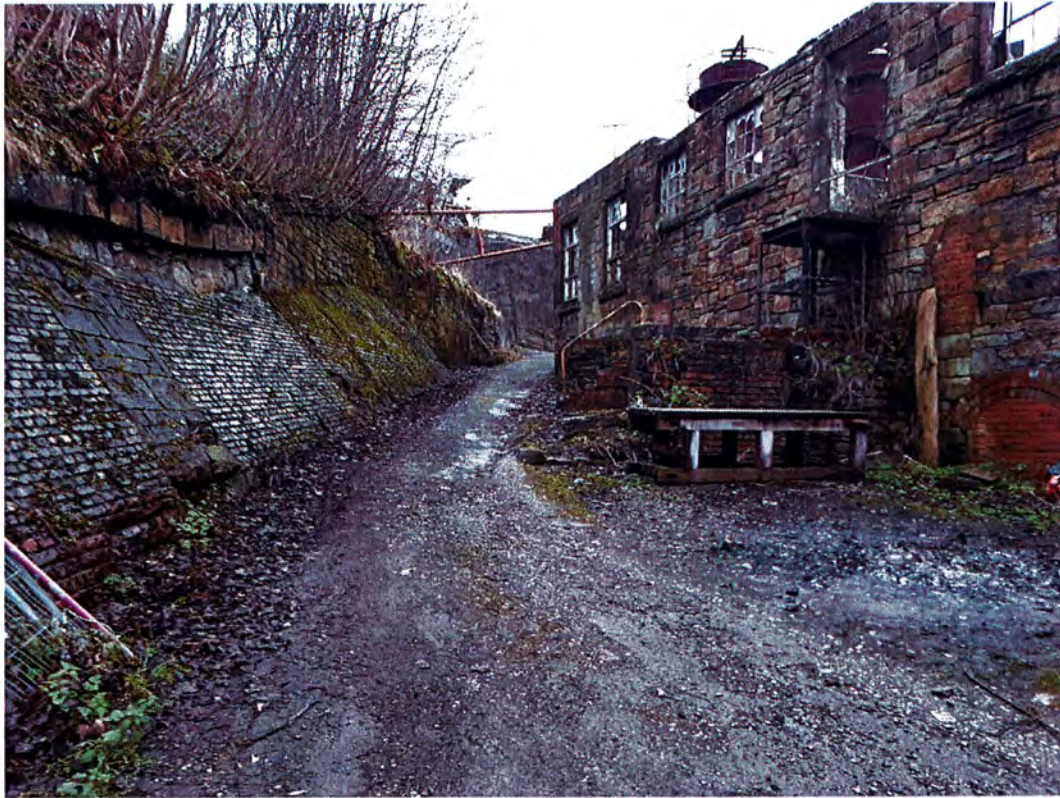
Photograph 13 Same path heading upslope
