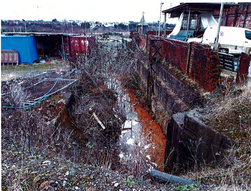
Photograph 5 drainage channel through site
