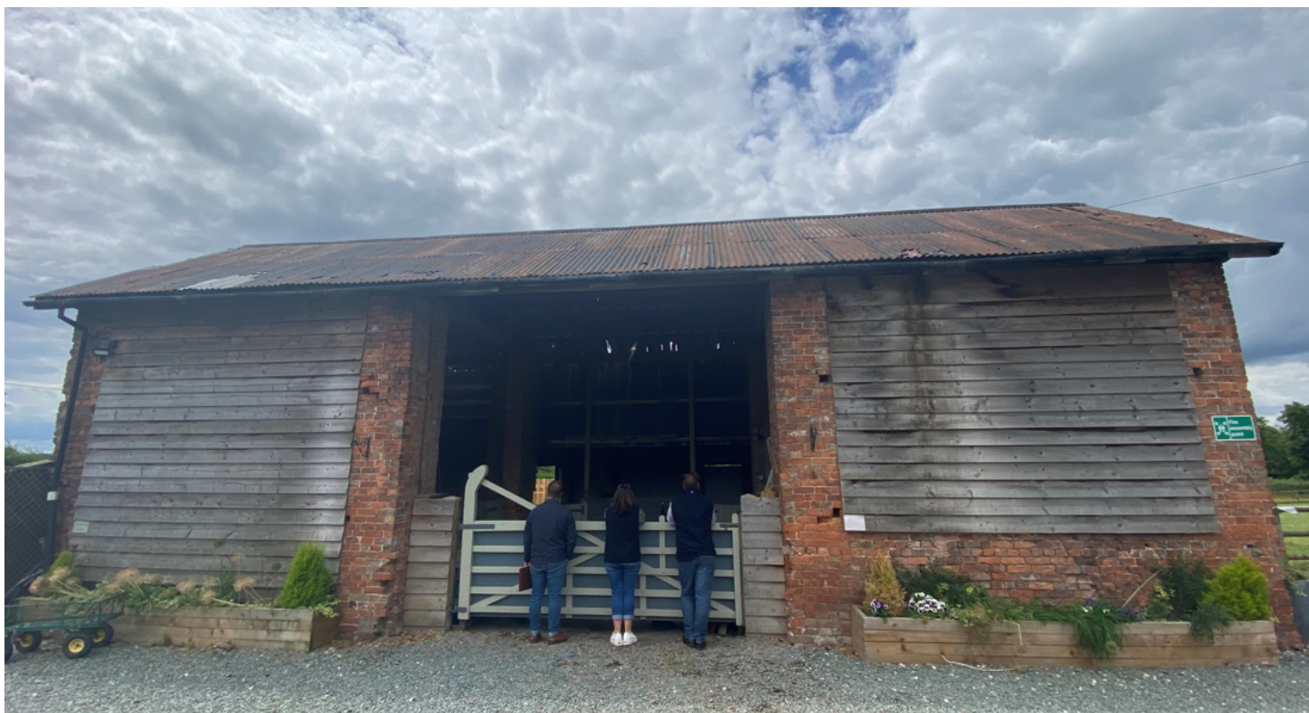
Fig. 5 Photograph of front elevation showing open portion and historic brickwork.
