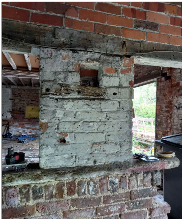
Plate 34. Detail of dividing wall between main barn and east room, looking west.
