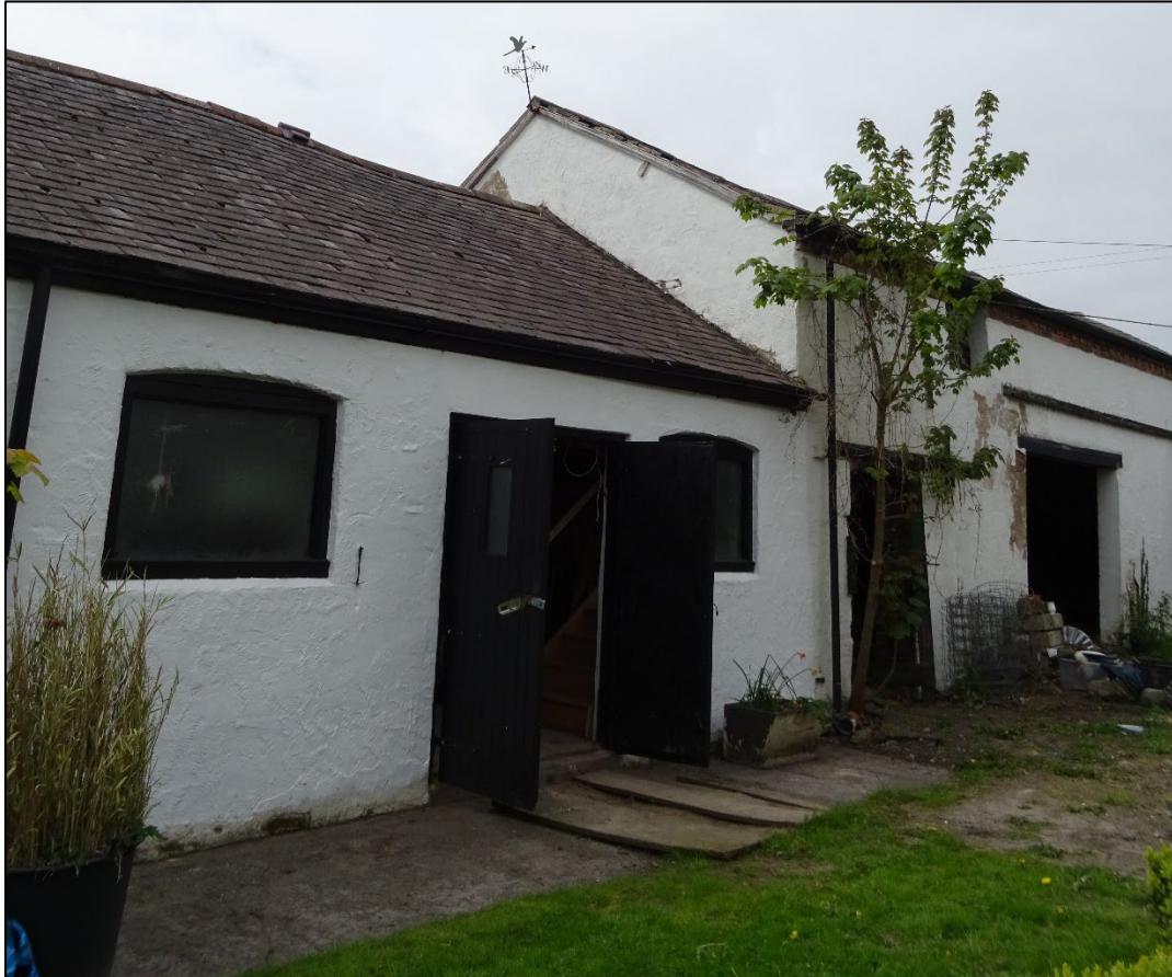
Plate 12. East-facing elevation of barn rising above adjoining single storey barn, looking south-west.
