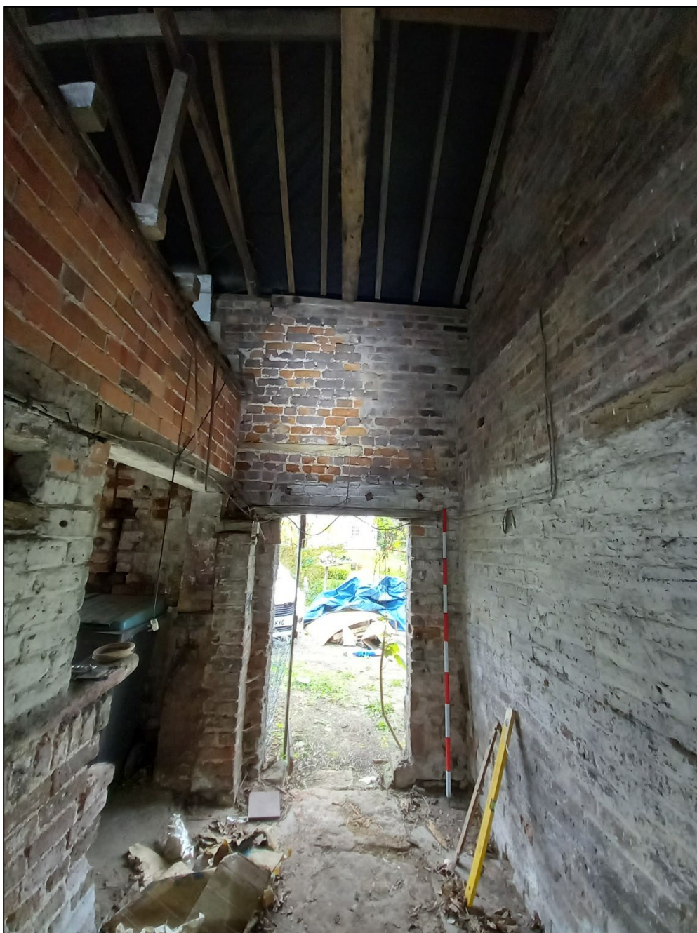
Plate 35. Front wall of east room of barn, looking north. 2m scale.
