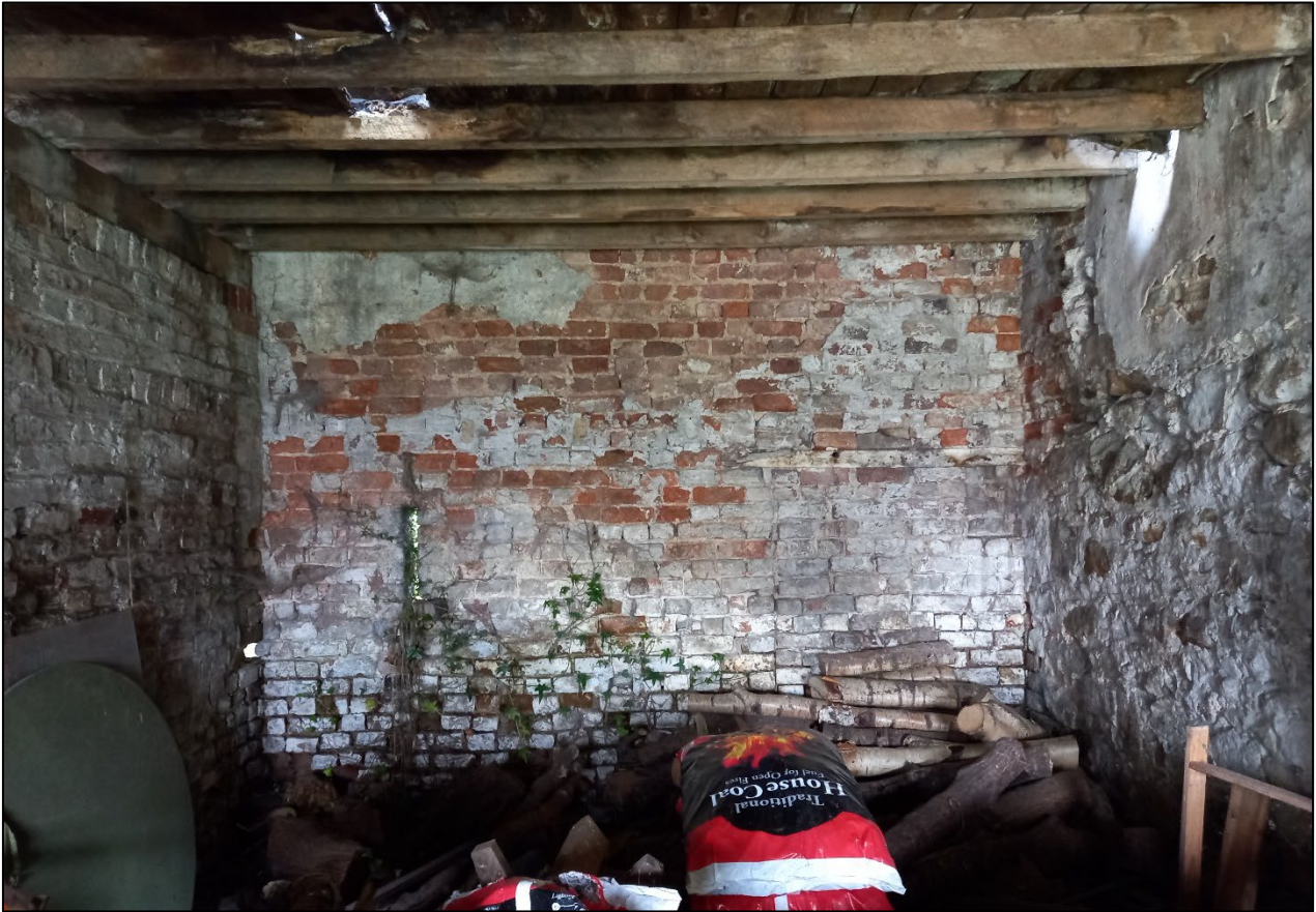
Plate 42. Rear wall of west room with blocked doorway to the west and slit window to the east, looking south.
