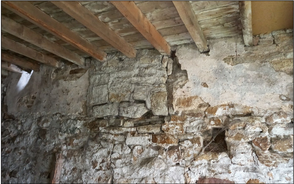
Plate 44. Blocked window to centre of west wall, rising above later floor level, looking west.
