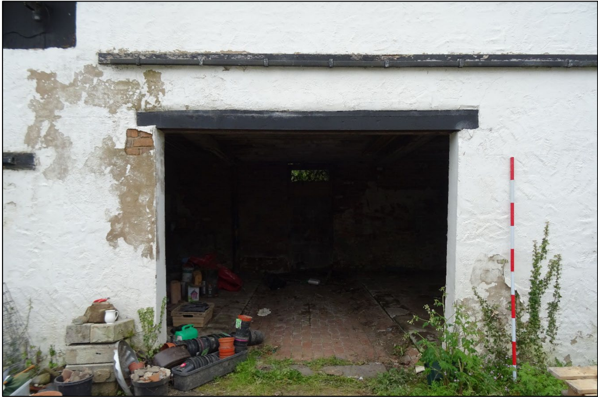
Plate 8. Cart doorway to centre of front elevation with track for sliding doors above, looking south. 2m scale.
