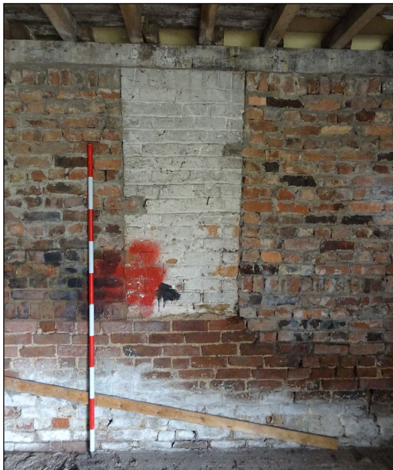
Plate 21. Detail of west interior wall with blocked opening, looking west. 2m scale.
