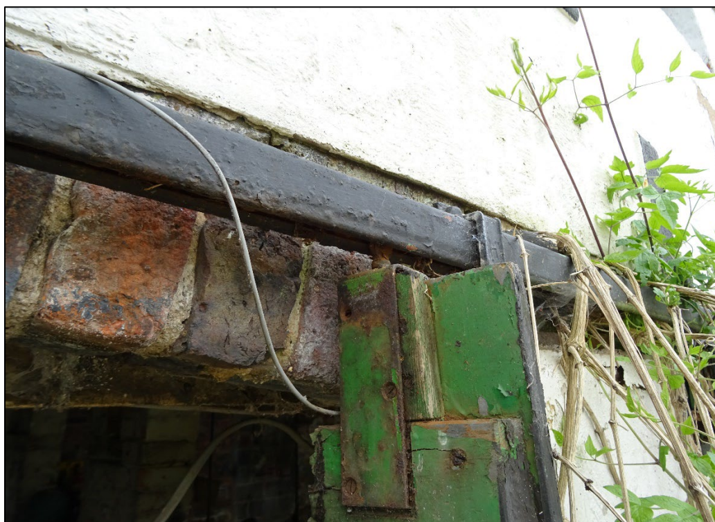
Plate 11. Detail of eastern door slide track with surviving section of wooden door, looking south-west.
