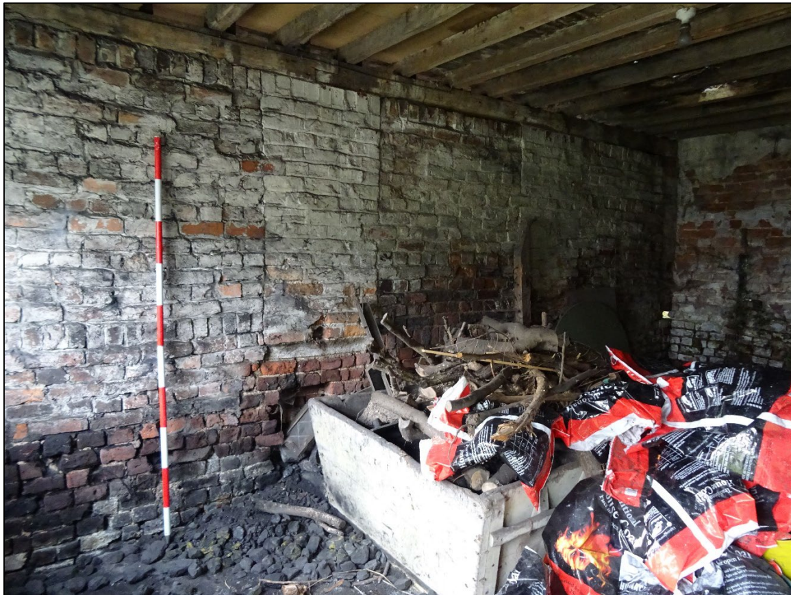
Plate 40. East interior wall with blocked openings, west room of barn, looking south-east. 2m scale.
