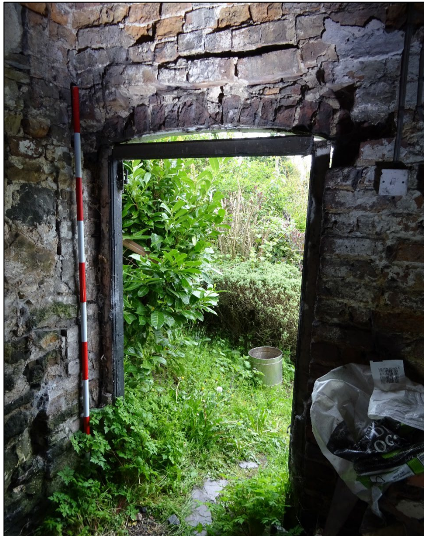
Plate 46. Doorway to front of west room of barn, looking north-west. 2m scale.
