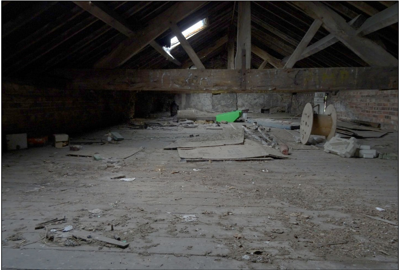
Plate 36. First floor/loft of barn, looking west.
