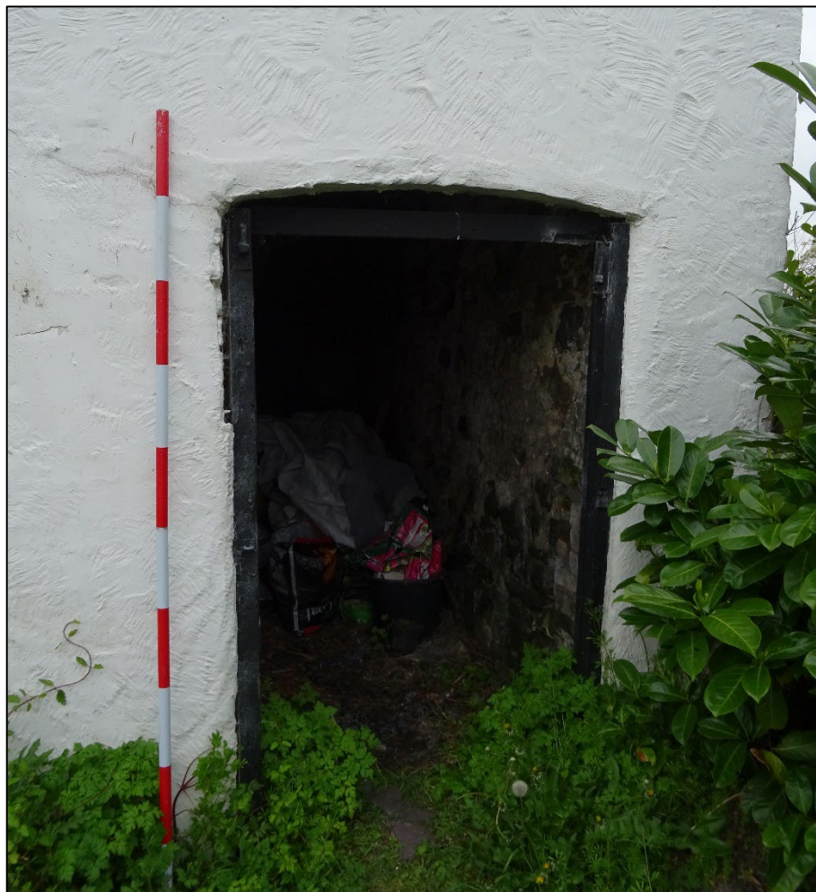
Plate 4. Wooden framed doorway at west end of front elevation of barn, looking south. 2m scale.
