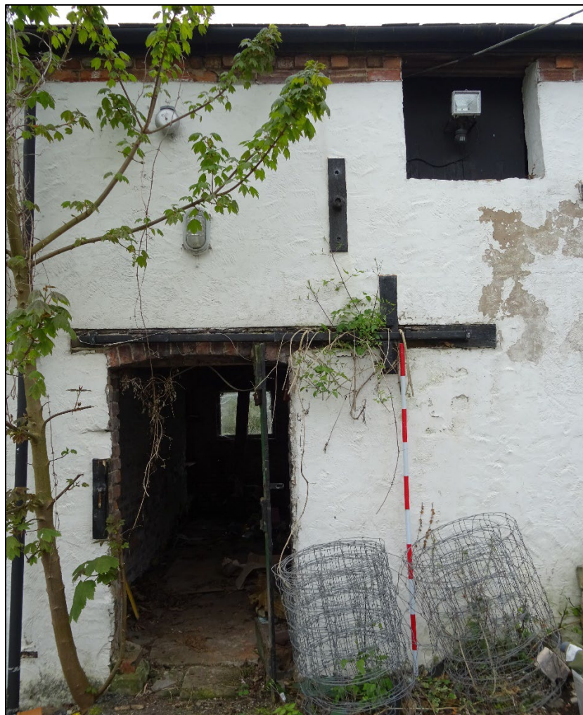
Plate 9. Doorway to east end of front elevation of barn with blocked window to first floor, looking south. 2m scale.
