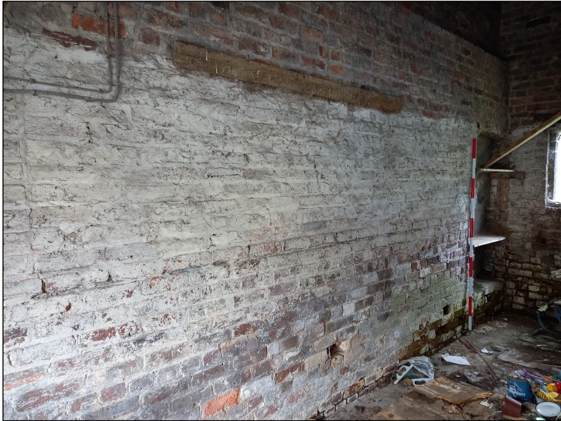
Plate 28. East wall of east room, looking south-east. 2m scale.
