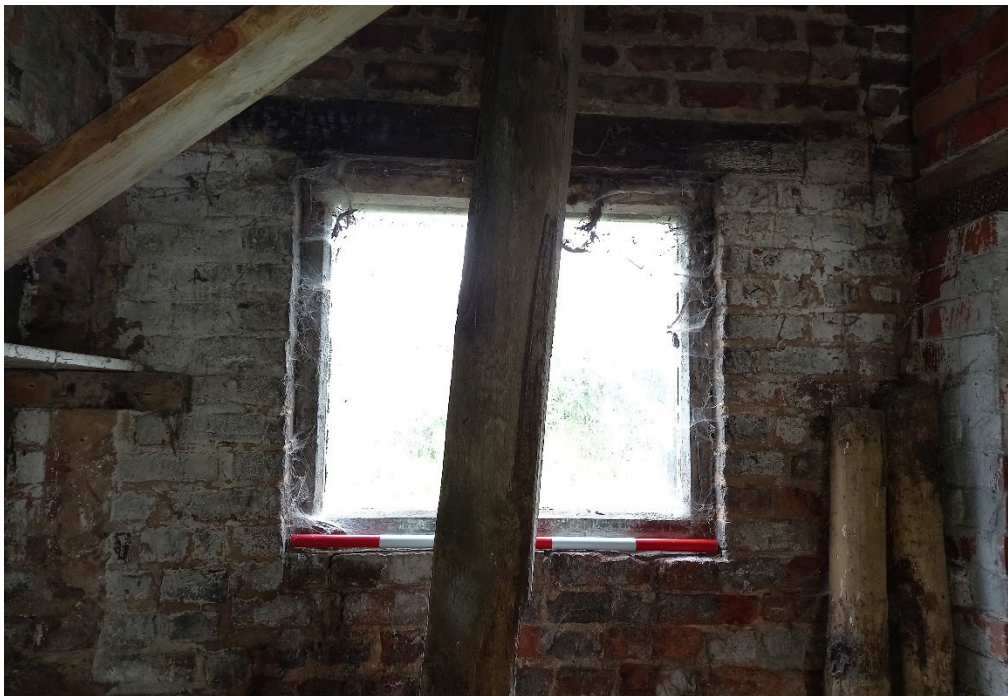
Plate 31. Wooden framed window to rear wall of east room, looking south. 1m scale.
