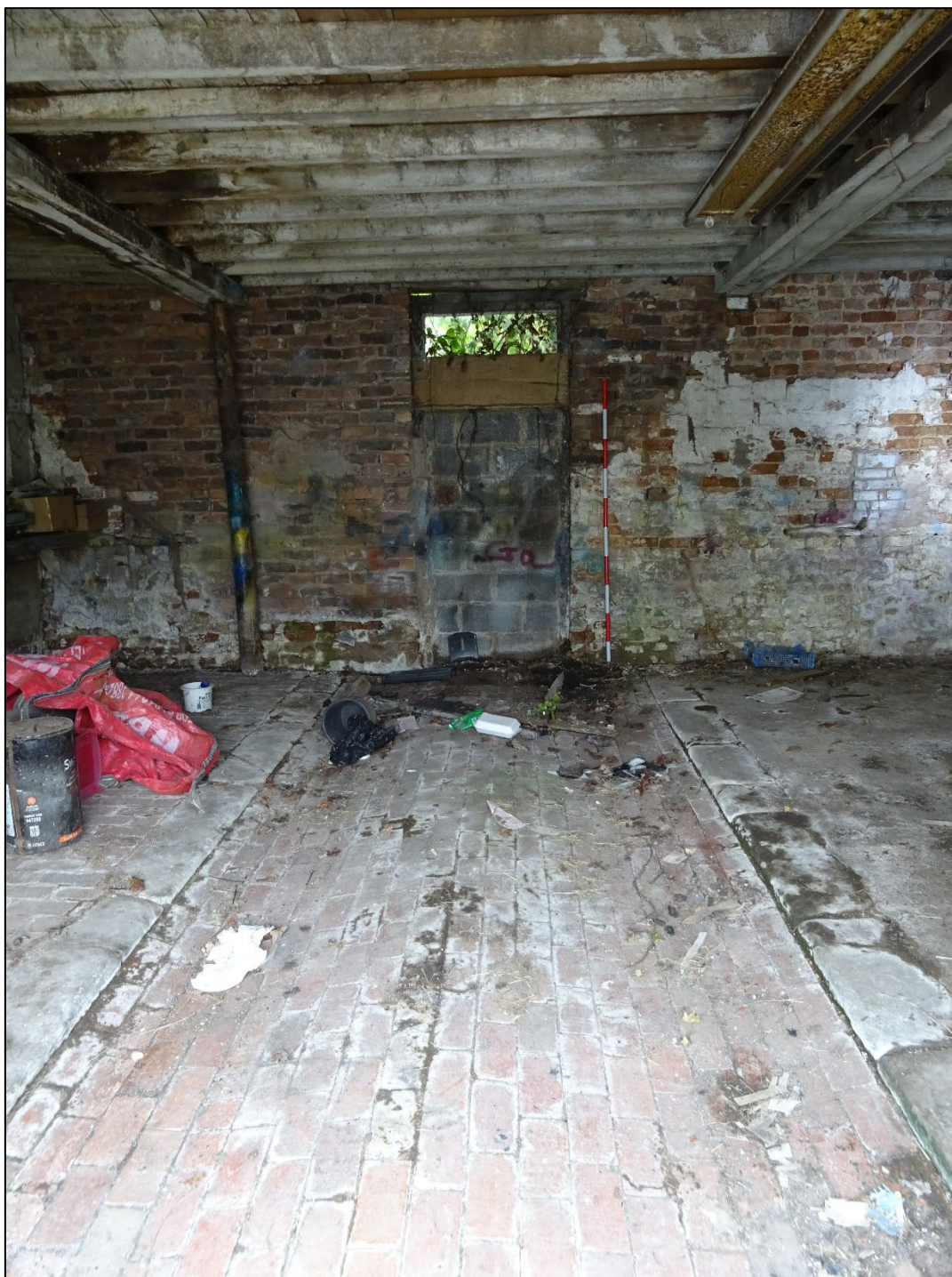
Plate 26. Brick floor with stone edging from cart doorway, looking south. 2m scale.
