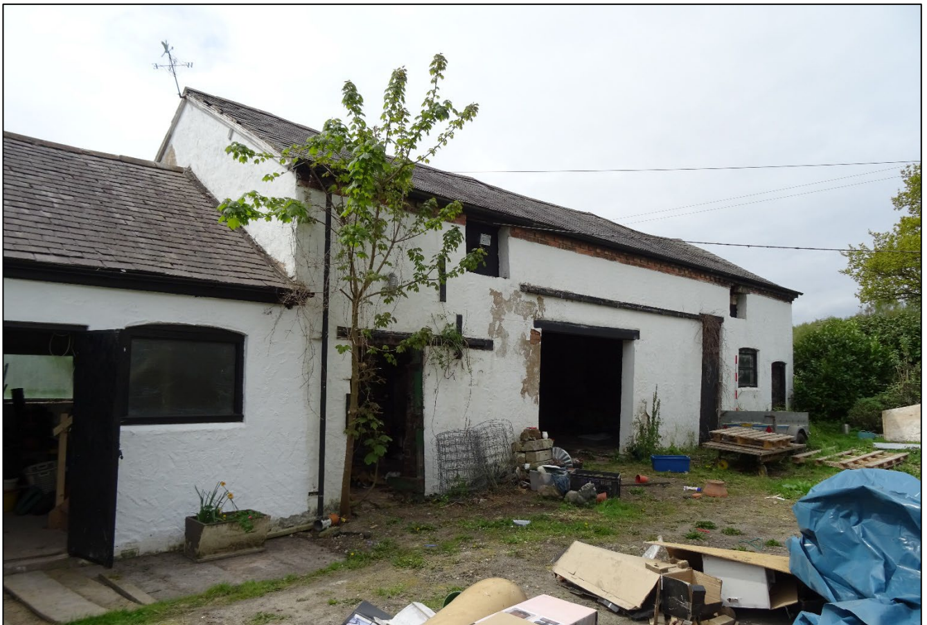
Plate 2. Front elevation of barn, looking south-west.
