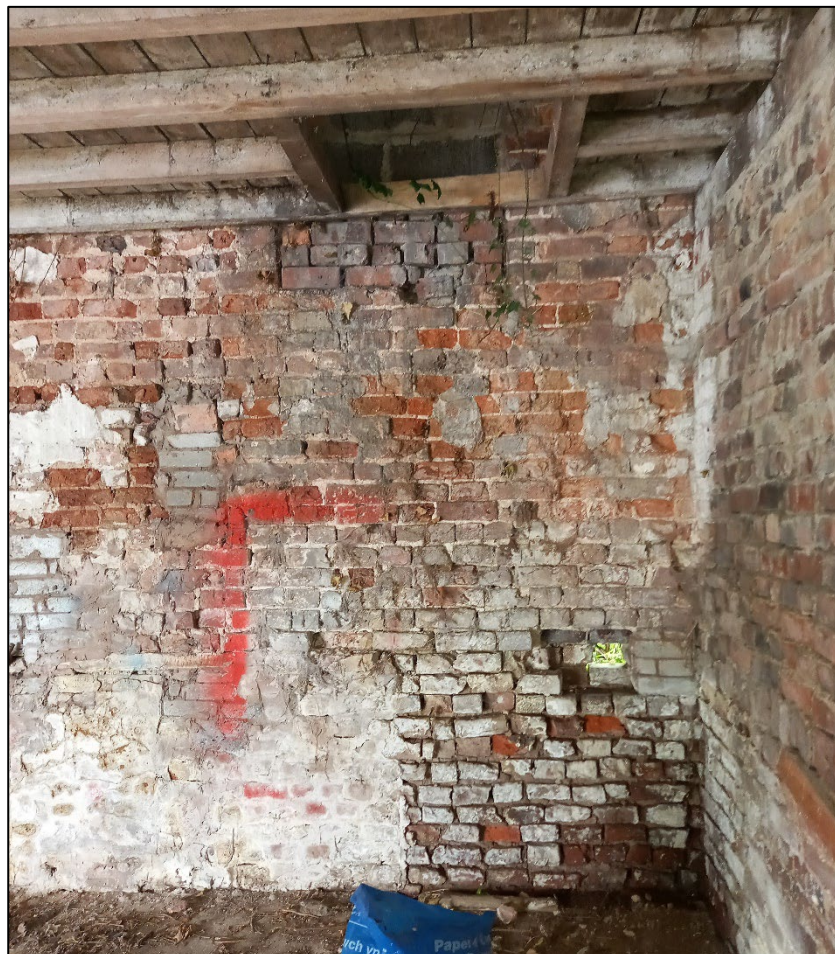
Plate 19. West end of rear wall with blocked window rising above later floor level, looking south.
