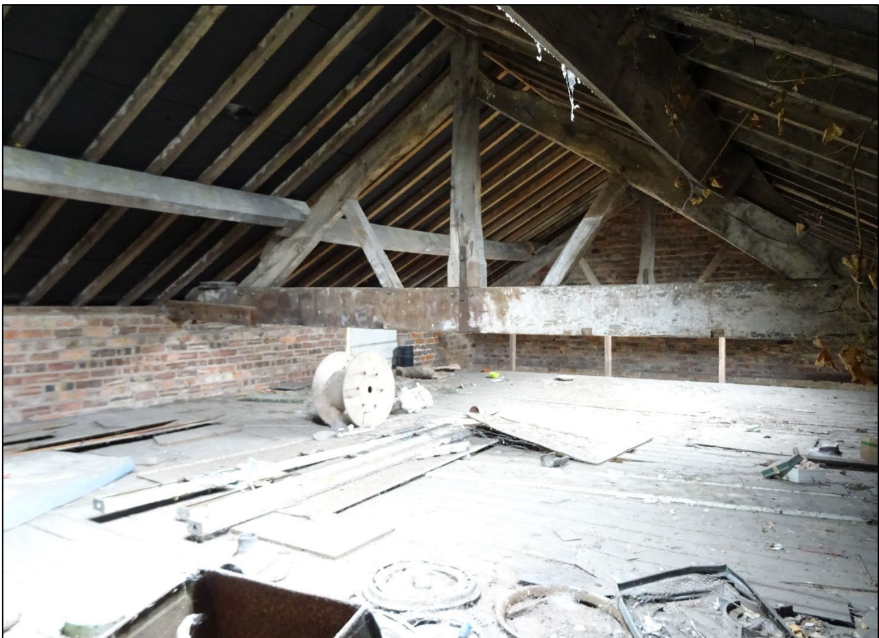
Plate 37. First floor/loft of barn, looking north-east.
