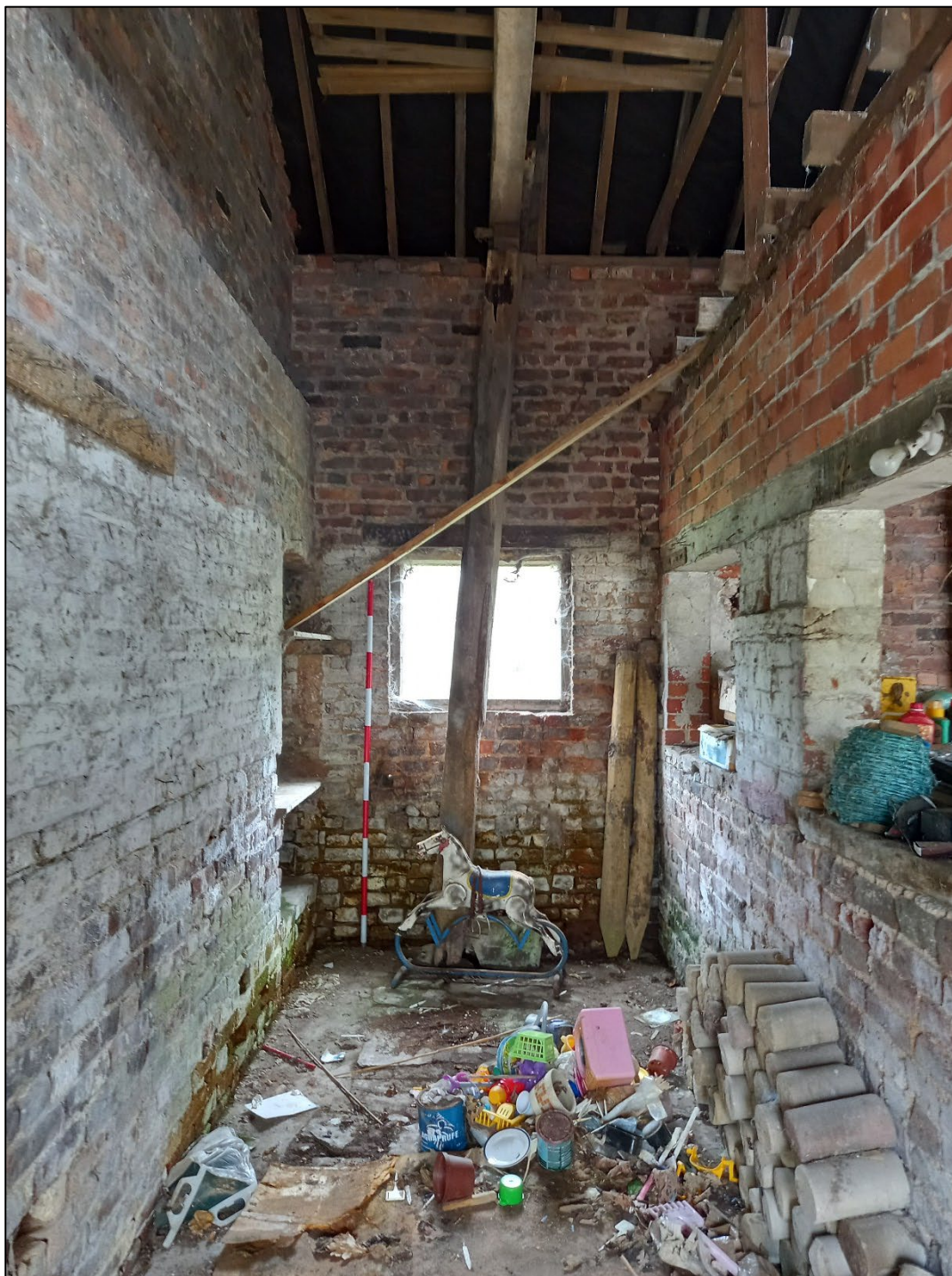
Plate 27. Small room to east end of barn, looking south. 2m scale.
