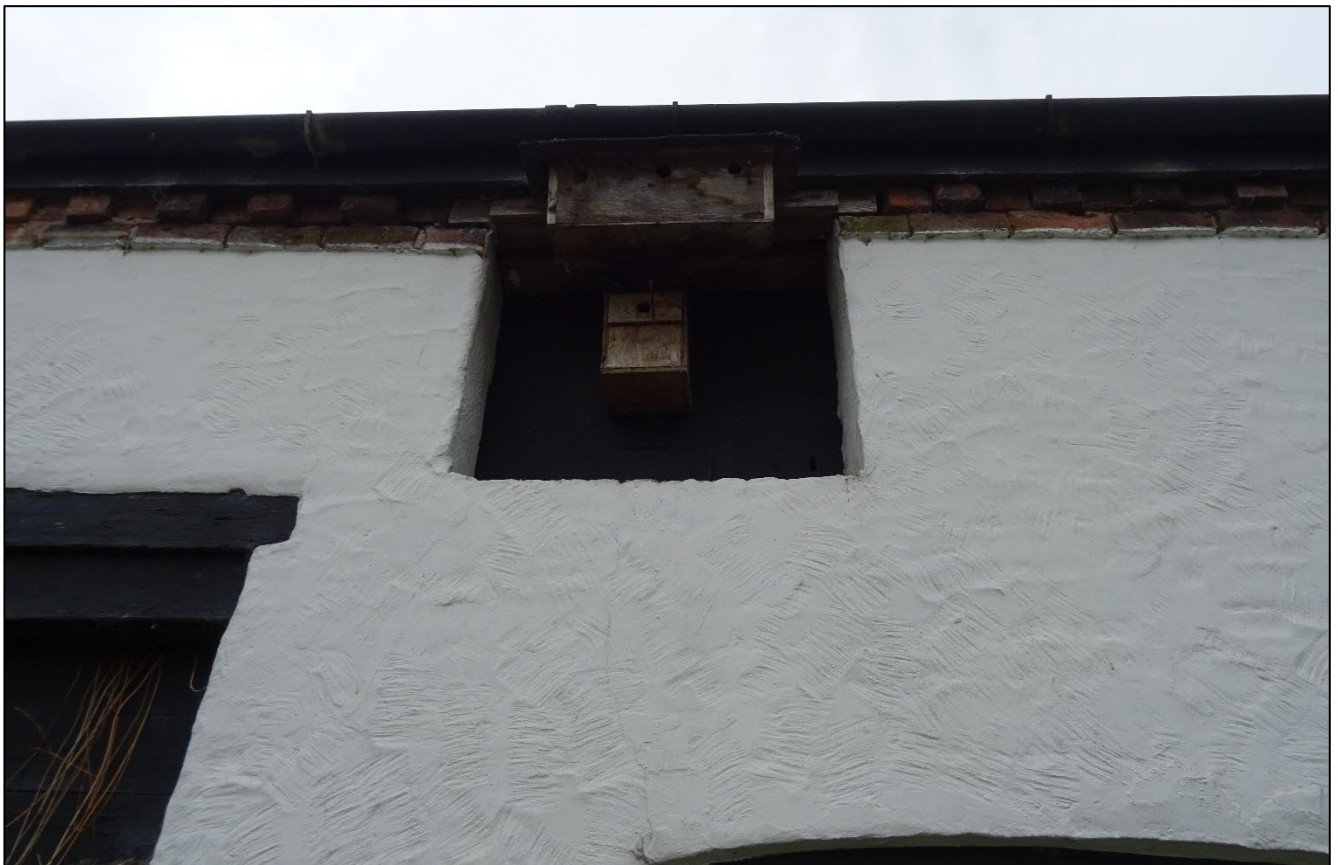
Plate 6. Blocked first floor window at west end of front elevation of barn, looking south.
