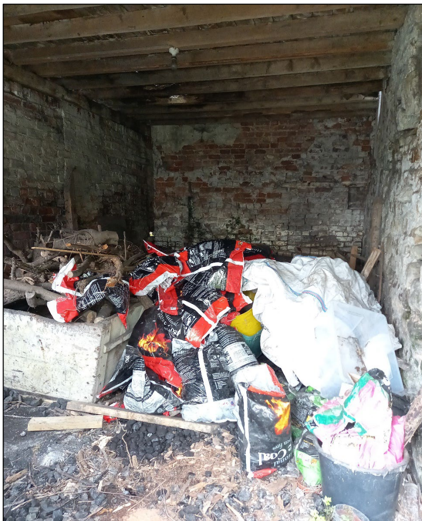
Plate 39. West room of barn, looking south.
