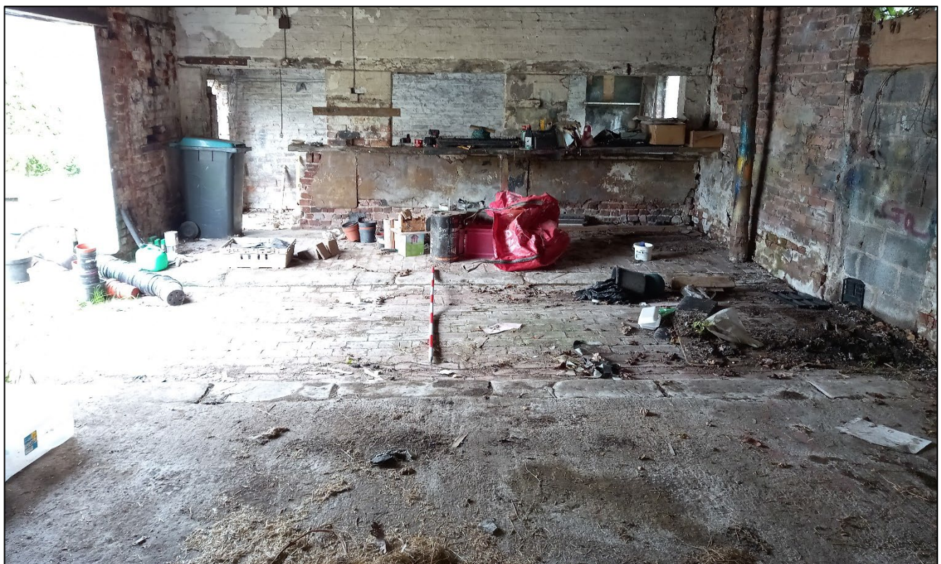
Plate 25. Poured concrete barn floor with stone edged brick section from the cart door, looking east. 2m scale.
