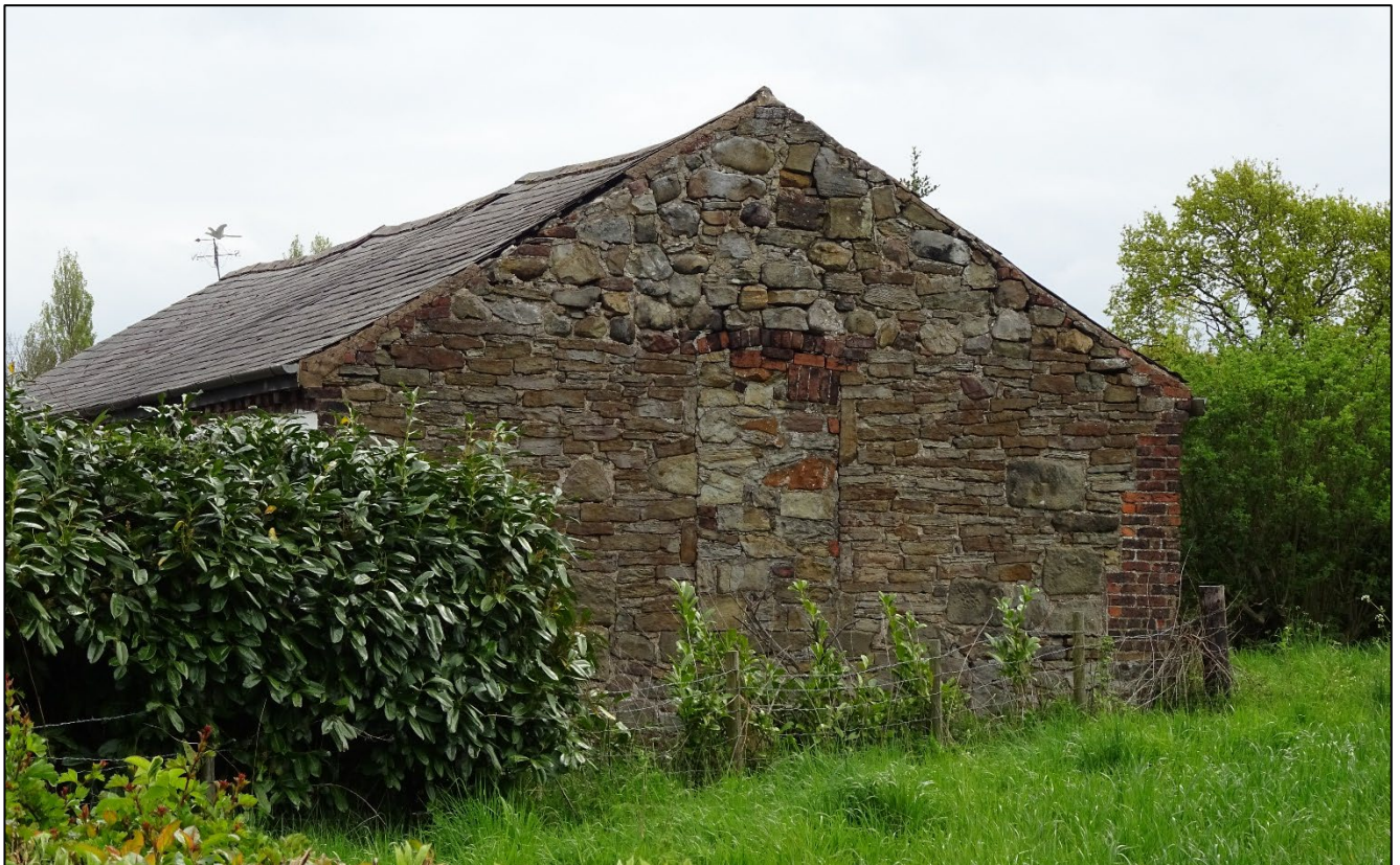
Plate 15. West-facing elevation of barn, looking south-east.
