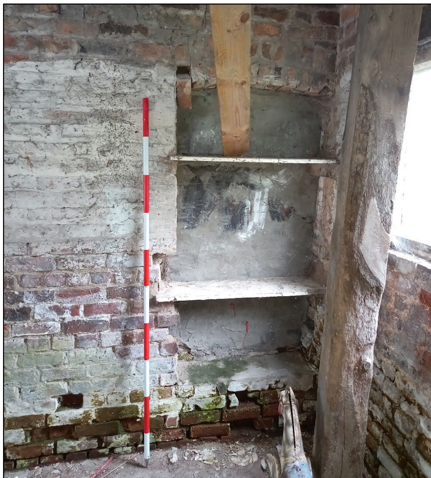
Plate 29. Alcove in blocked doorway at south end of east wall, looking east. 2m scale.
