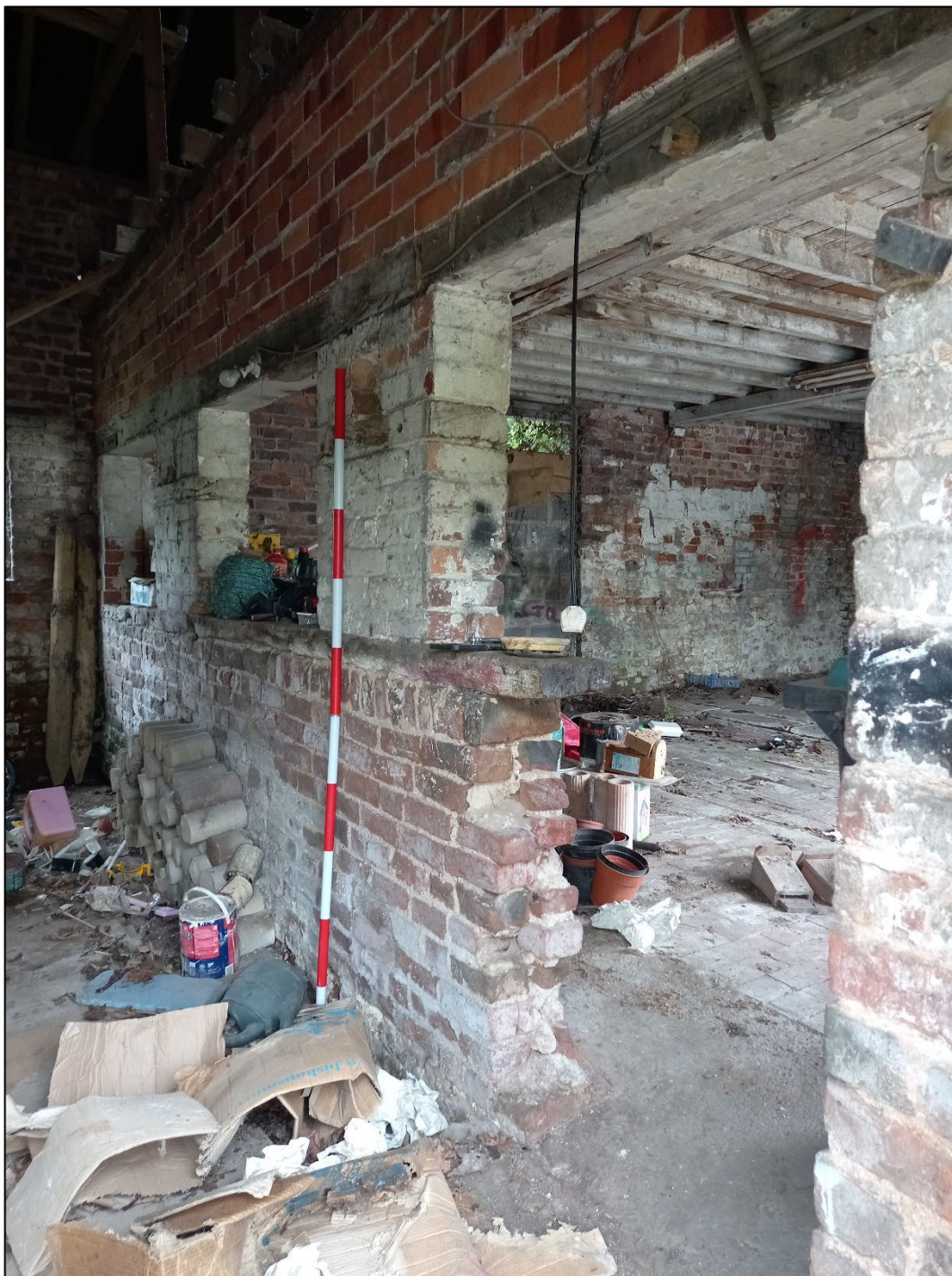
Plate 32. Interior wall between main barn and east room, looking south-west. 2m scale.
