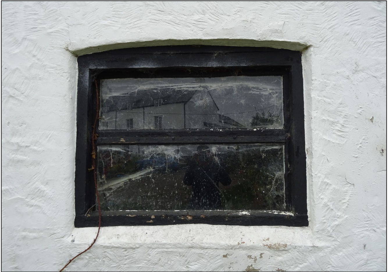
Plate 5. Ground floor wooden framed window to west end of front elevation, looking south.
