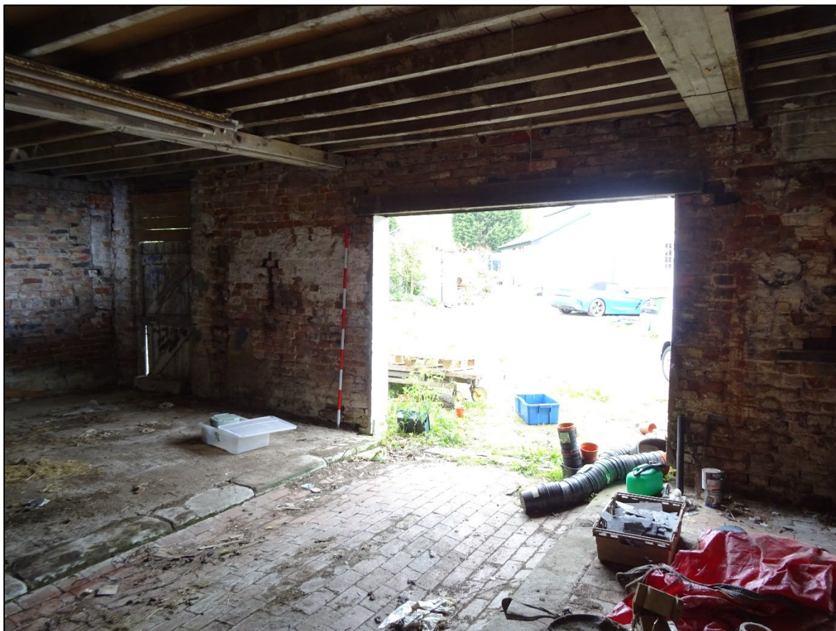
Plate 22. Front wall of barn, looking north-west. 2m scale.
