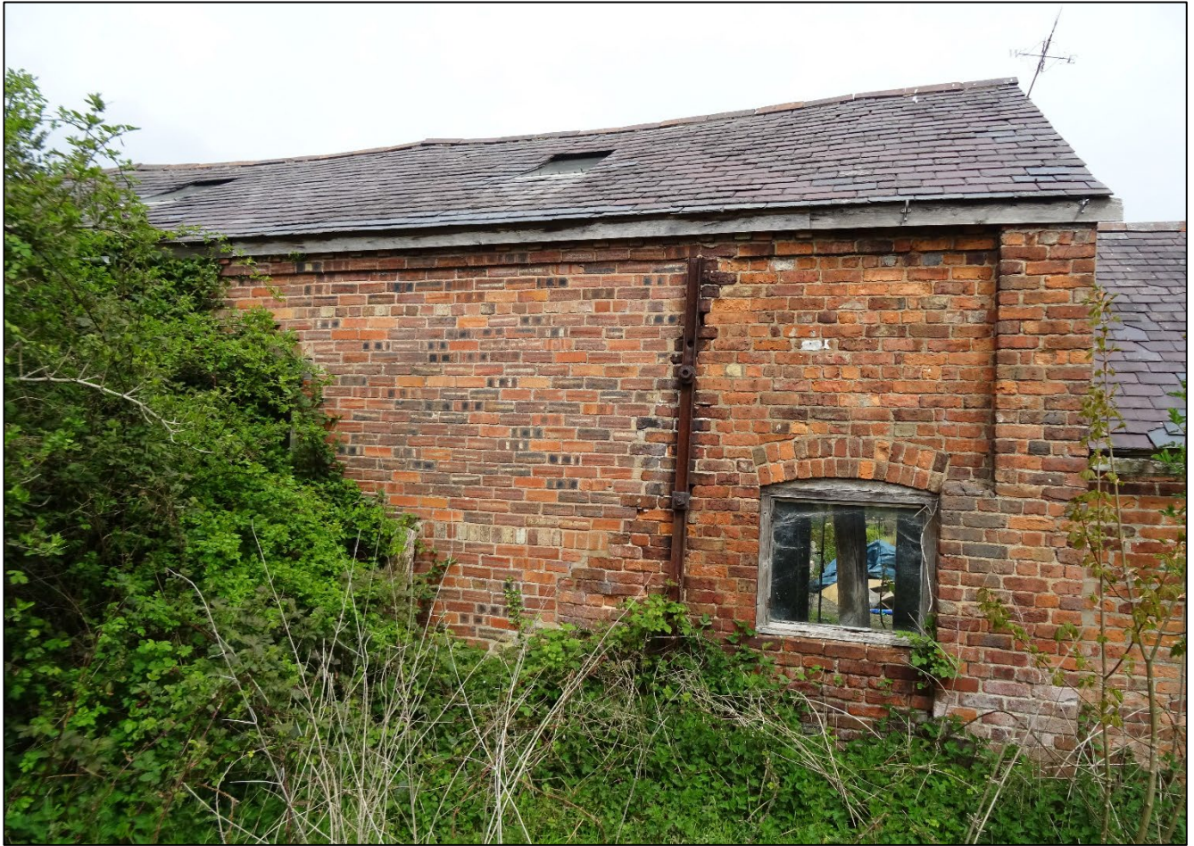
Plate 14. South-facing elevation of barn, looking north.
