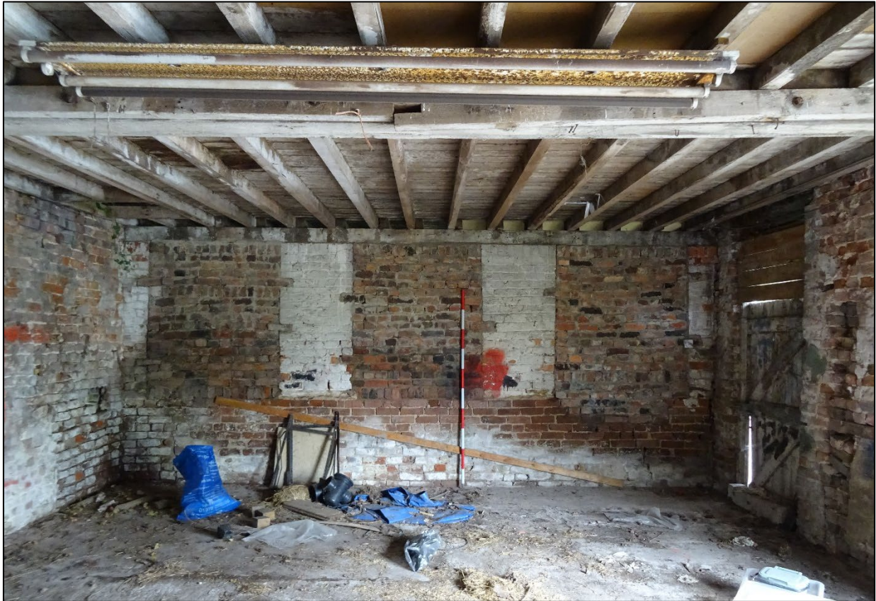
Plate 20. West interior wall of barn, with blocked openings to western room, looking west. 2m scale.
