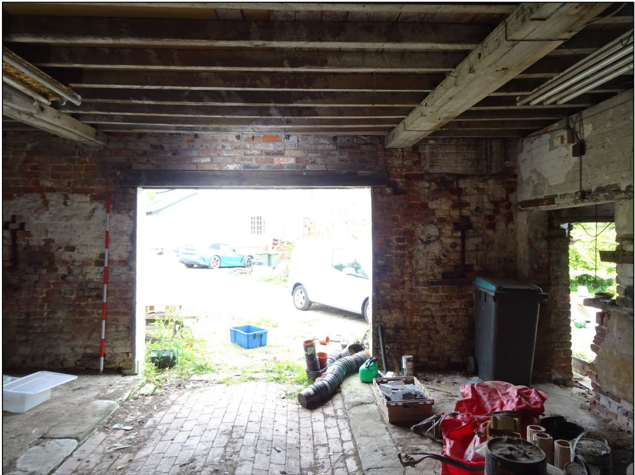
Plate 24. Cart doorway to centre of front wall of barn, looking north. 2m scale.
