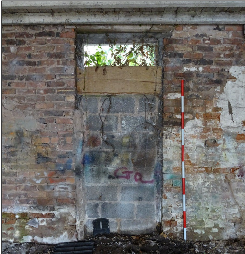
Plate 18. Blocked doorway to centre of rear wall of barn, looking south. 2m scale.
