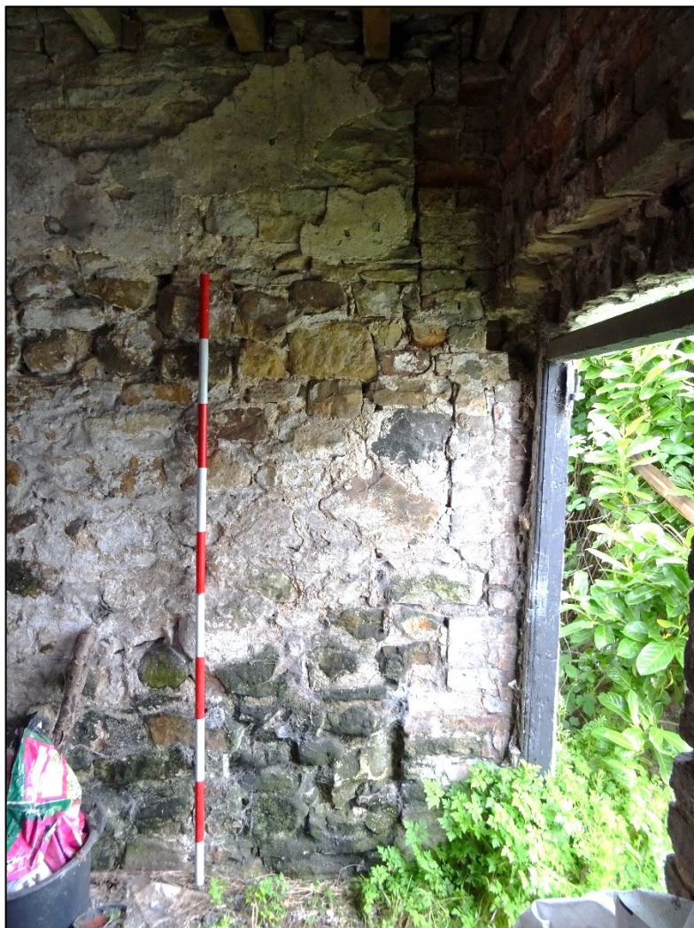
Plate 45. North end of west wall of barn interior, looking west. 2m scale.
