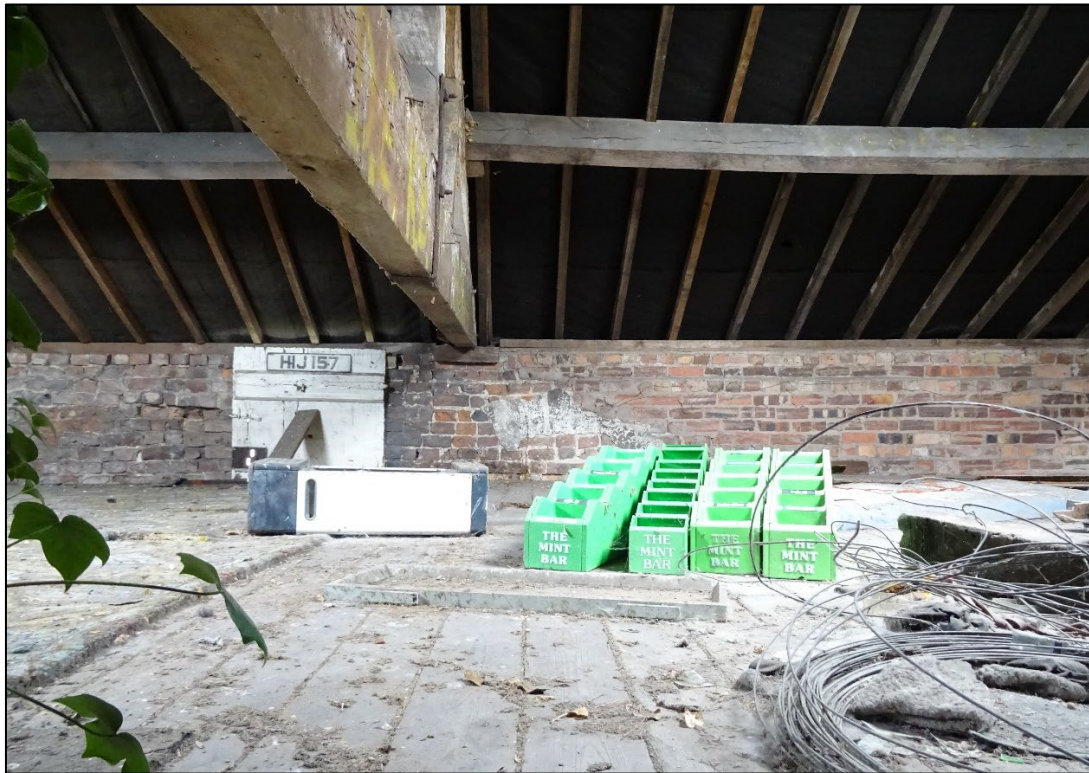
Plate 38. First floor/loft of barn, looking north.
