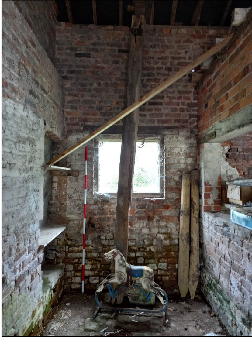
Plate 30. Rear wall of east room, looking south. 2m scale.
