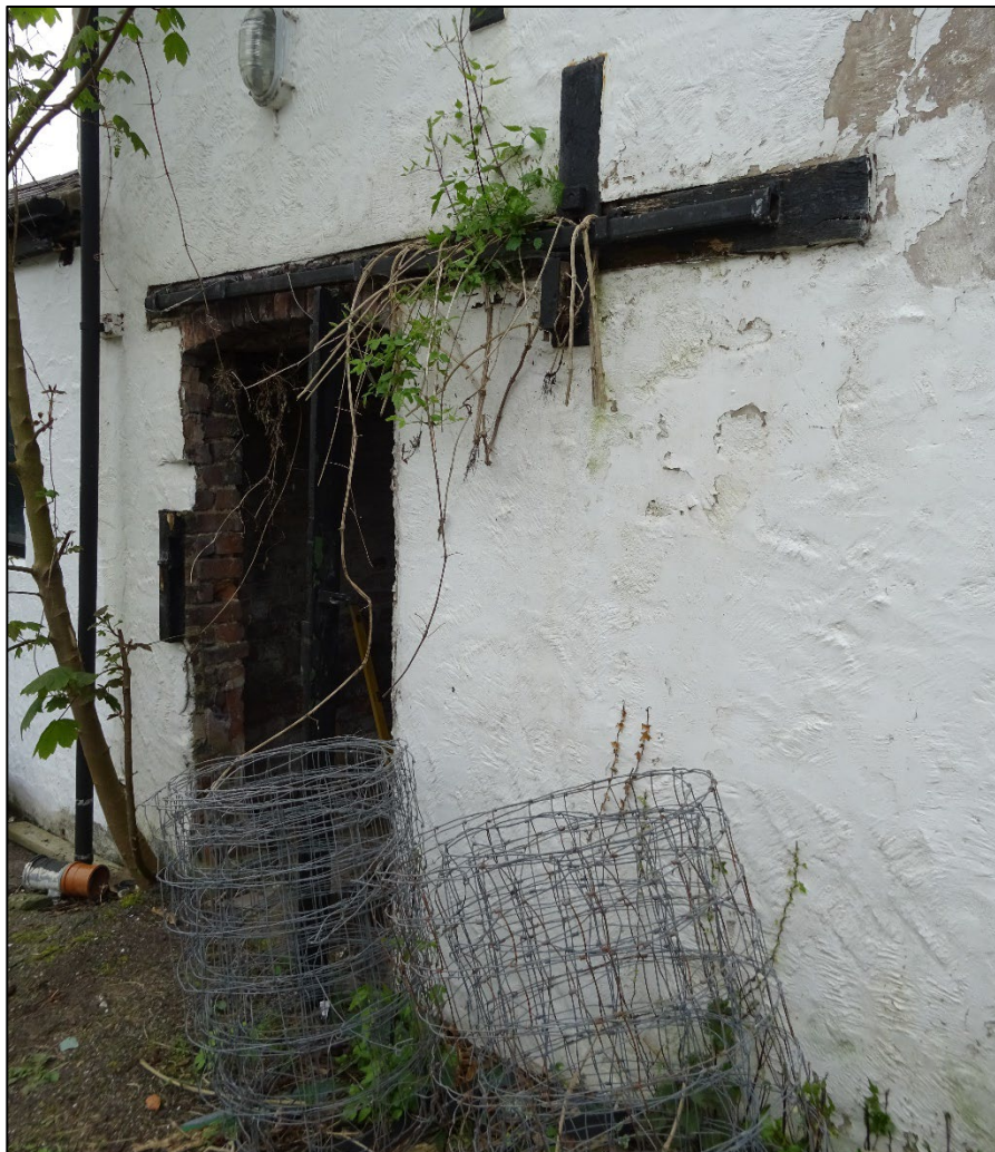
Plate 10. Door to east end of front elevation with sliding door track above, looking south-east.
