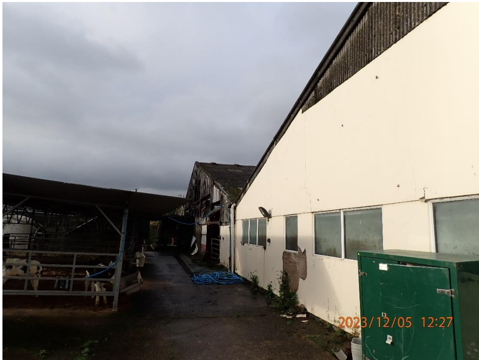
Southern elevation of existing dairy sheds at Target Note 9.
