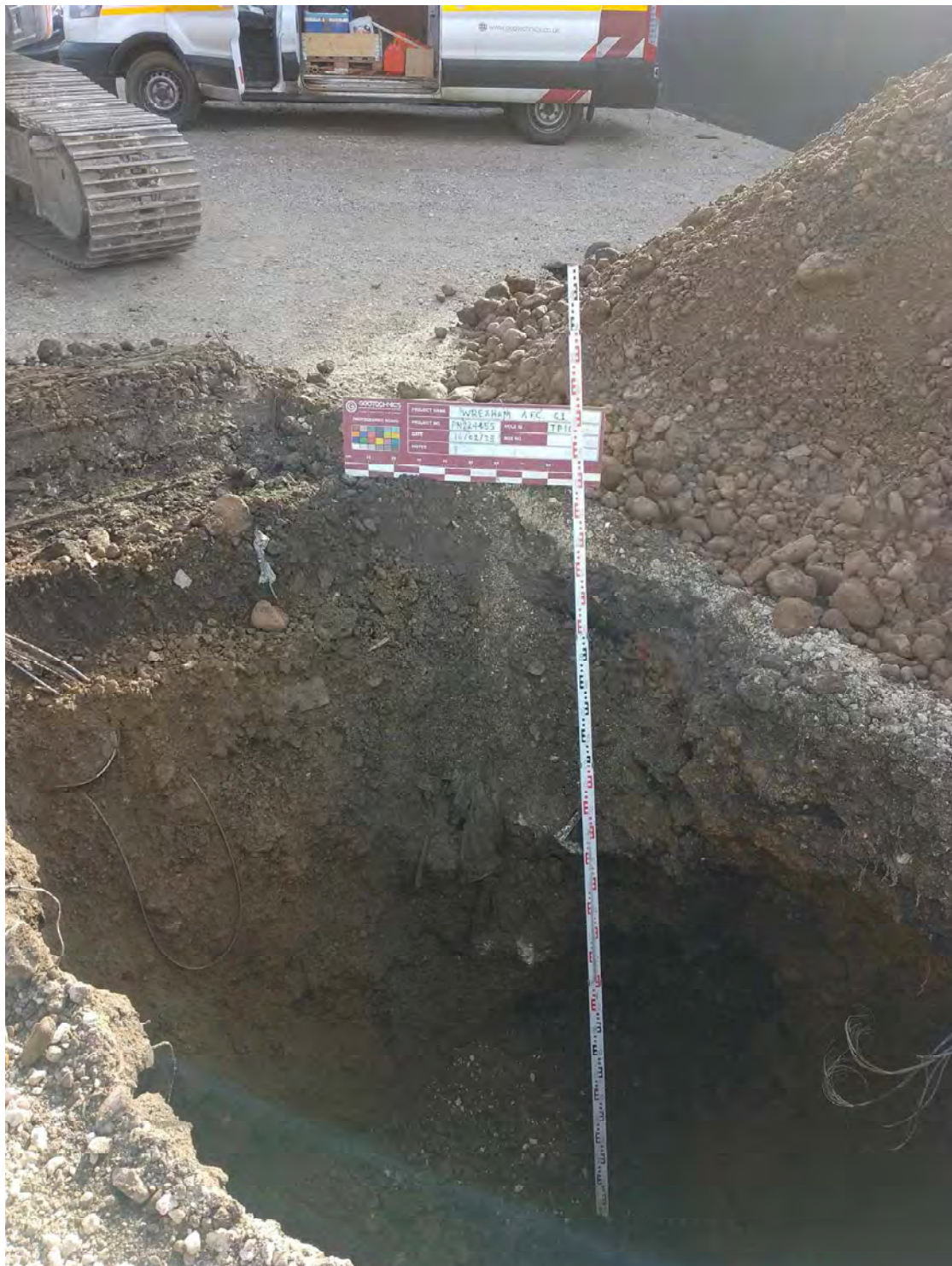
Trial Pit TPI04 (5) - Looking Southeast
