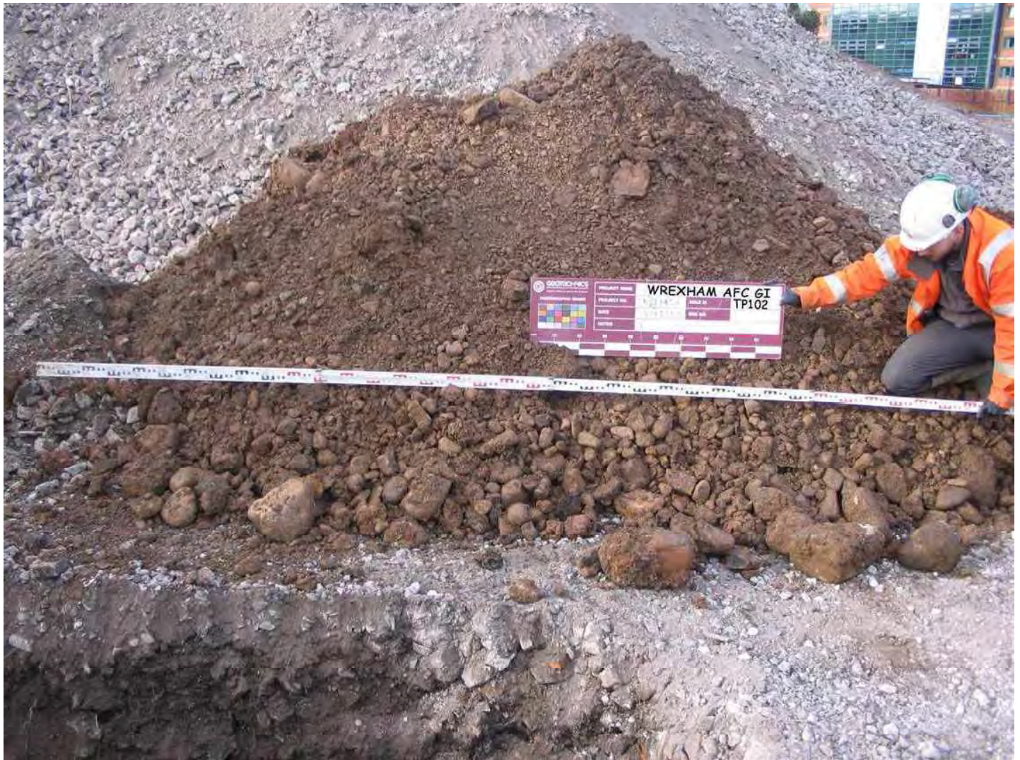
Trial Pit TP102 (3) Arisings
