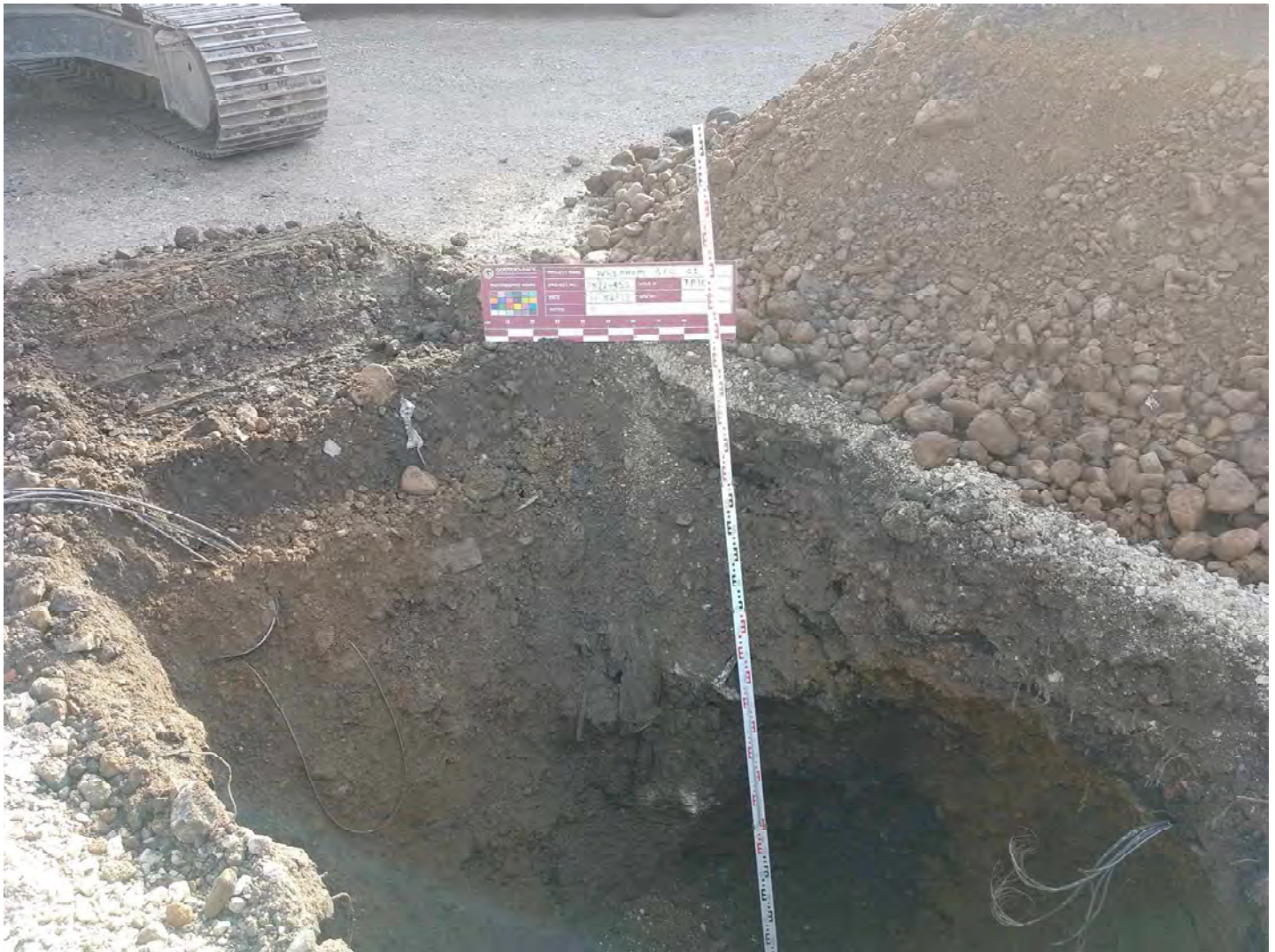
Trial Pit TPI04 (6) - Looking Southeast
