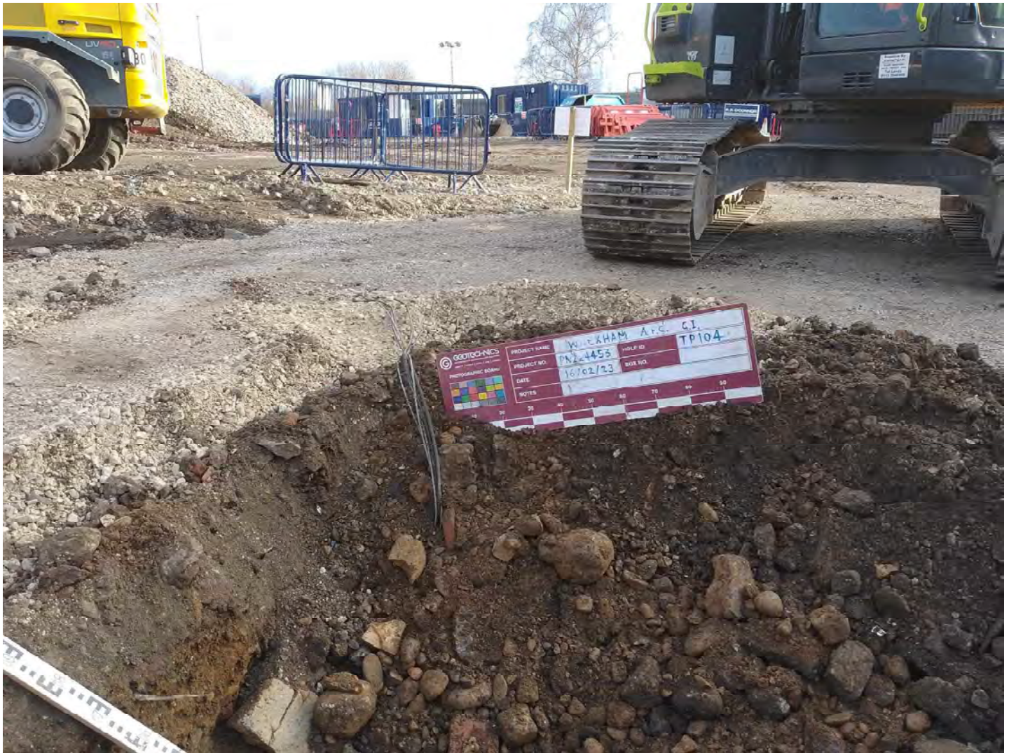
Trial Pit TP104 (3) - Looking Northeast
