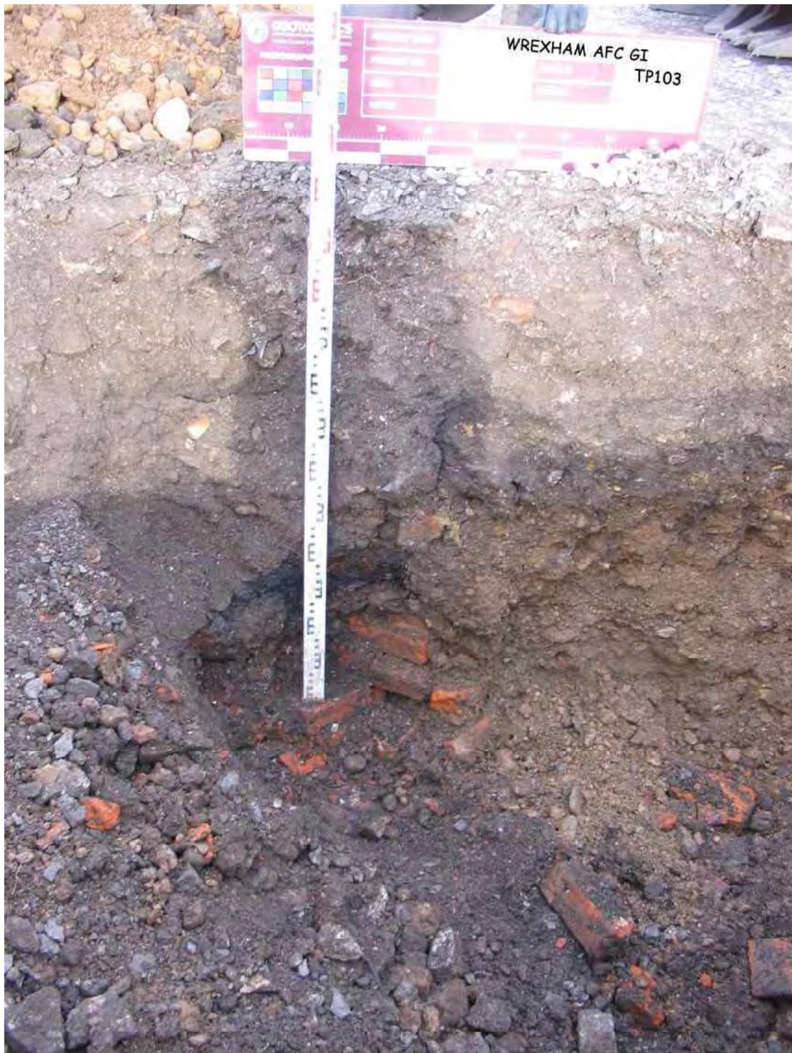
Trial Pit TP103 (I) - Close-up of brick wall
