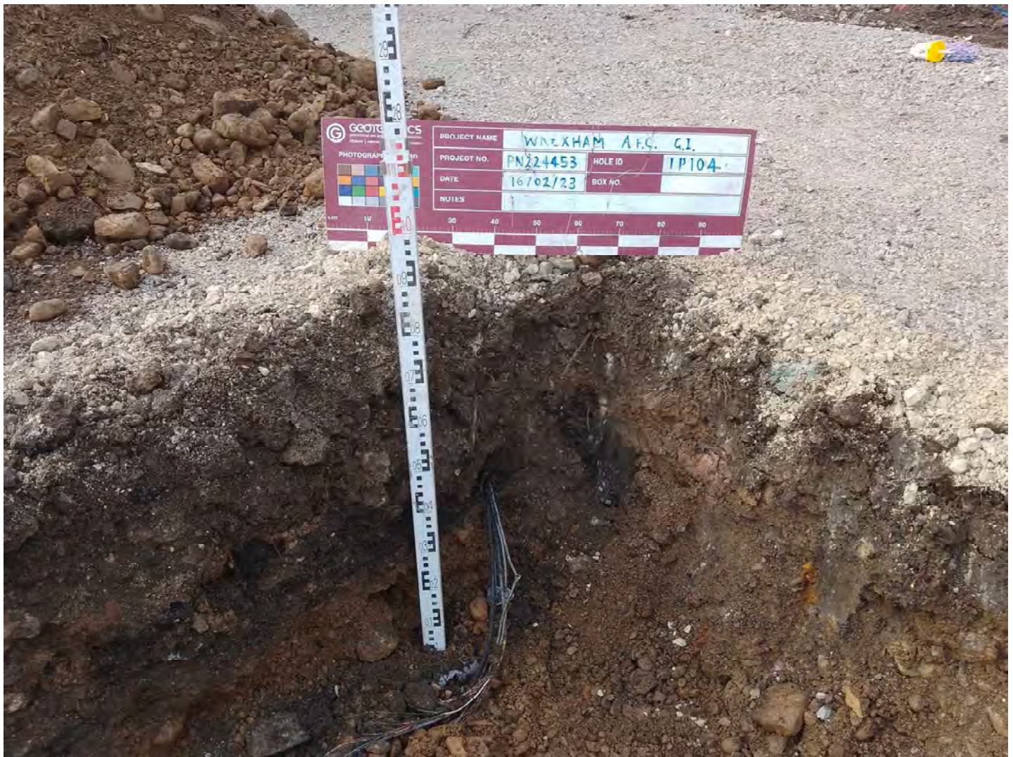
Trial Pit TP104 (2) - Looking Southwest
