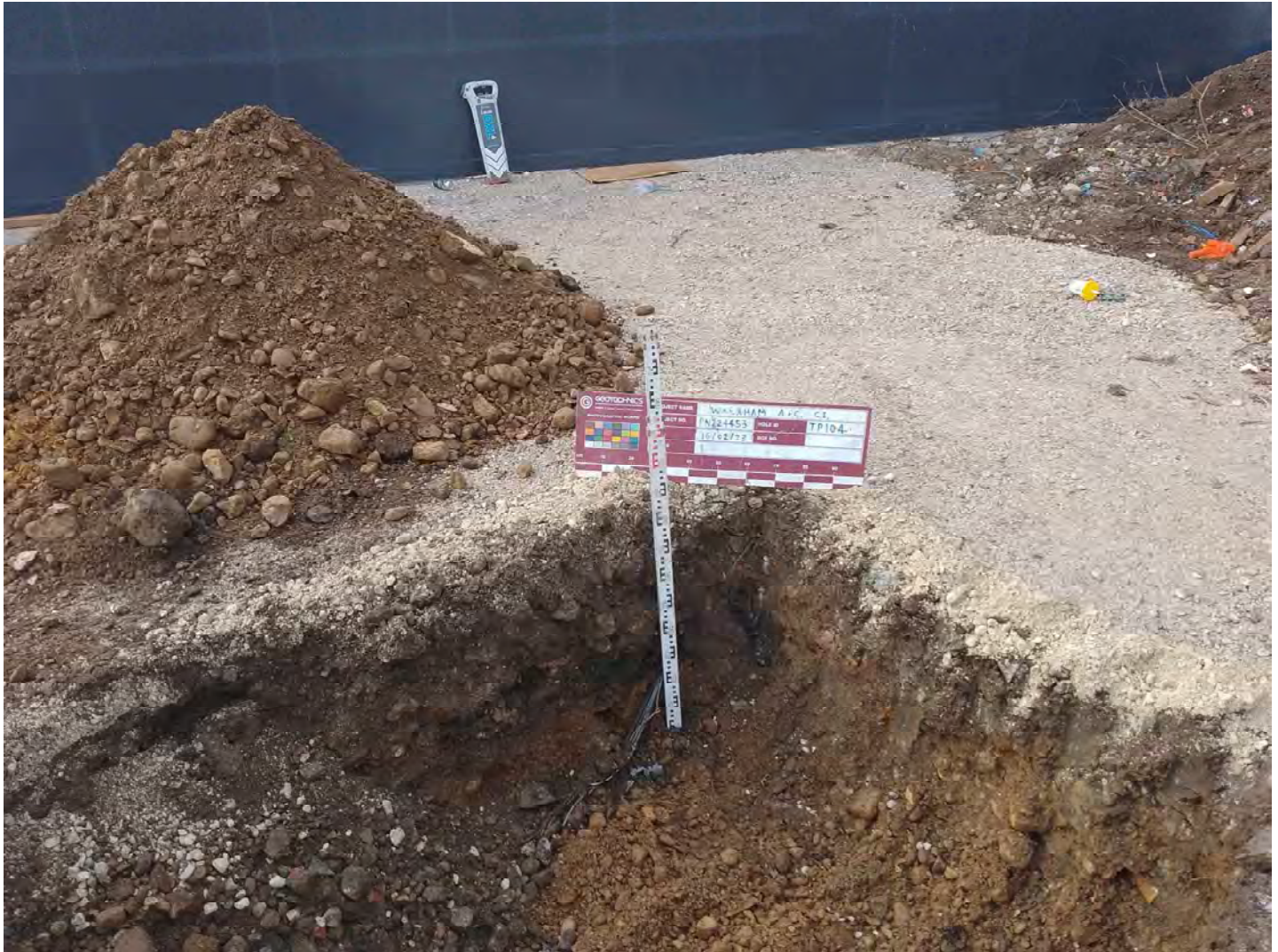
Trial Pit TP104 (I) - Looking Southwest
