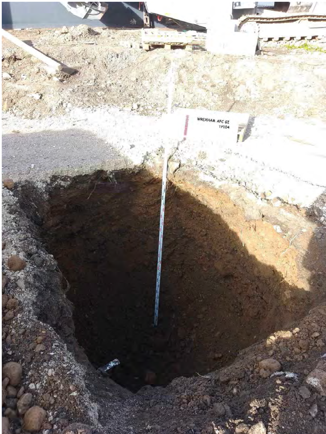
Trial Pit TP104 (7) - Looking Northwest
