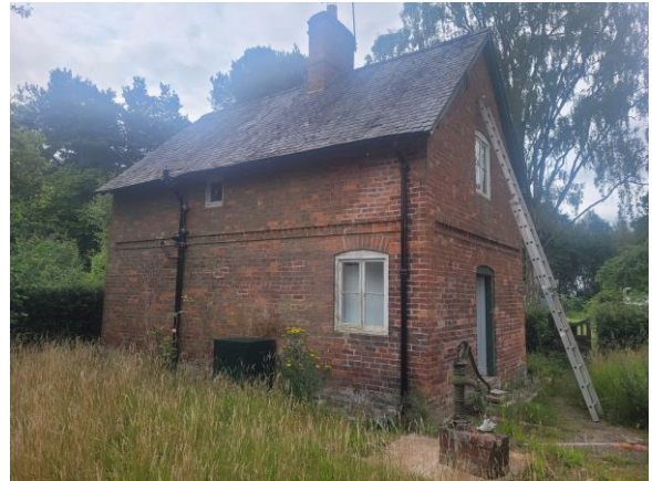
P2: NE (side) + NW (gable) elevations: looking S
