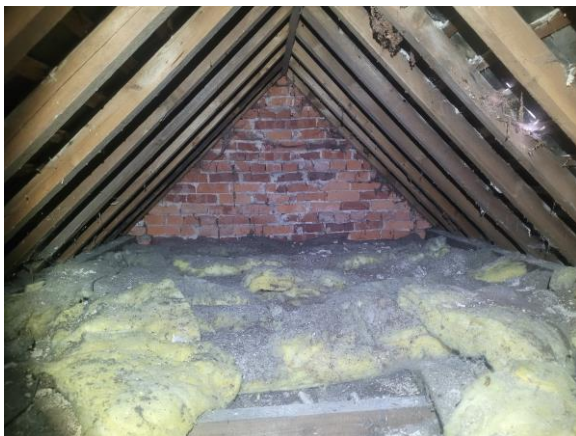
P3: S loft: viewed from the N end, looking SE
