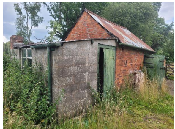
P10: SW (end) + SE (side) elevations: looking NNE
