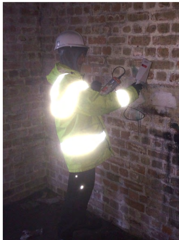
Figure A4 Carrying out internal building surveys
