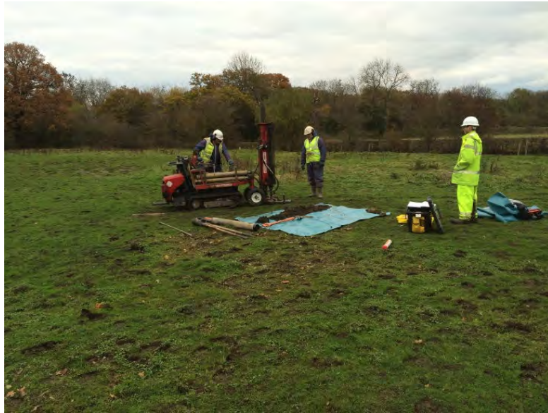
Figure A7 The health physics surveyor supervises drilling works and monitors excavated material.
