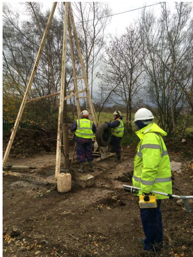
Figure A8 Supervising and monitoring drilling works.
