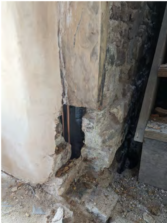
ABOVE - A before and after of the repaired brickwork during the drying out process, the lime mortar lightens in colour as it dries.
