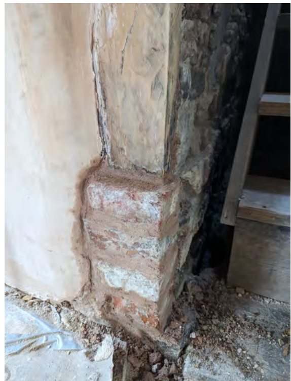
ABOVE - A before and after of the repaired brickwork during the drying out process, the lime mortar lightens in colour as it dries.
