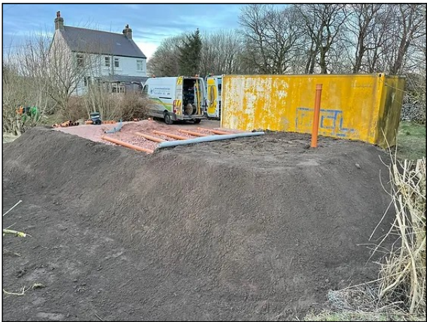
Drainage Mound Completion - ready for landscaping
