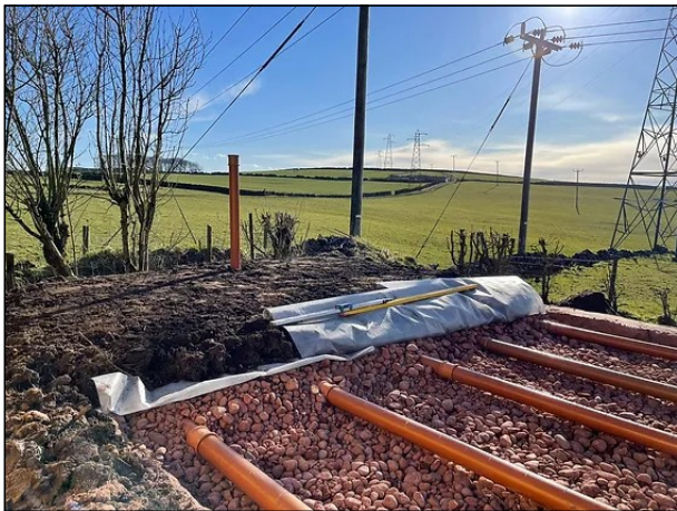
Drainage Mound detail and material that goes into the mound landscaping can be added to disguise the mound
