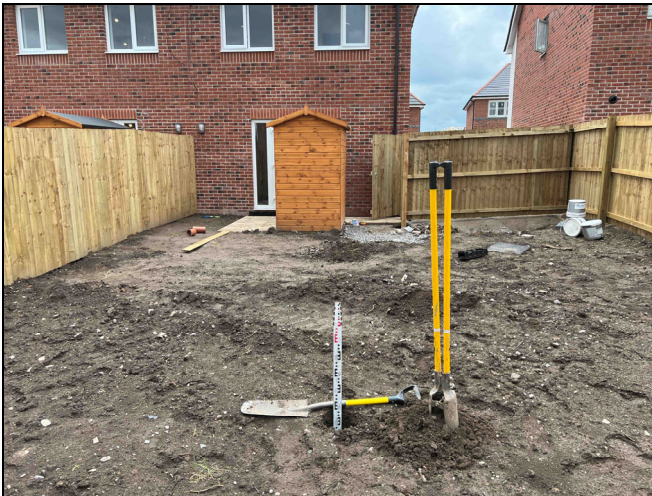
Photographs 7 & 8: Showing the depth of the inert cover and location of the validation hole within the rear garden of Plot 352 and the depth of inert cover achieved. Photographs taken 20 th June 2023.
