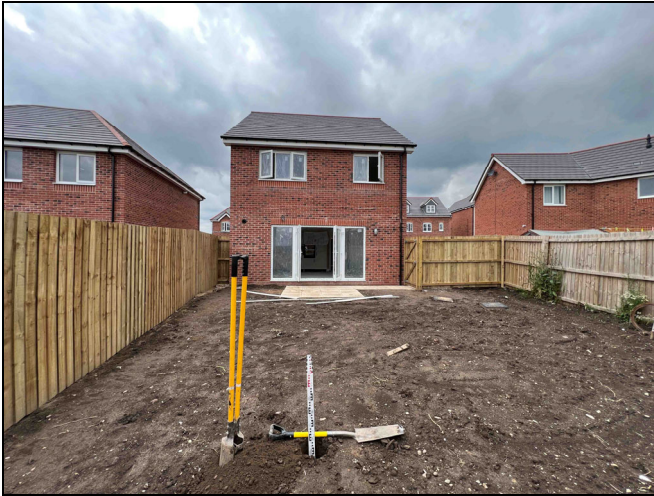
Photographs 4 & 5: Showing the depth of the inert cover and location of the validation hole within the rear garden of Plot 351 and the depth of inert cover achieved. Photographs taken 20 th June 2023.
