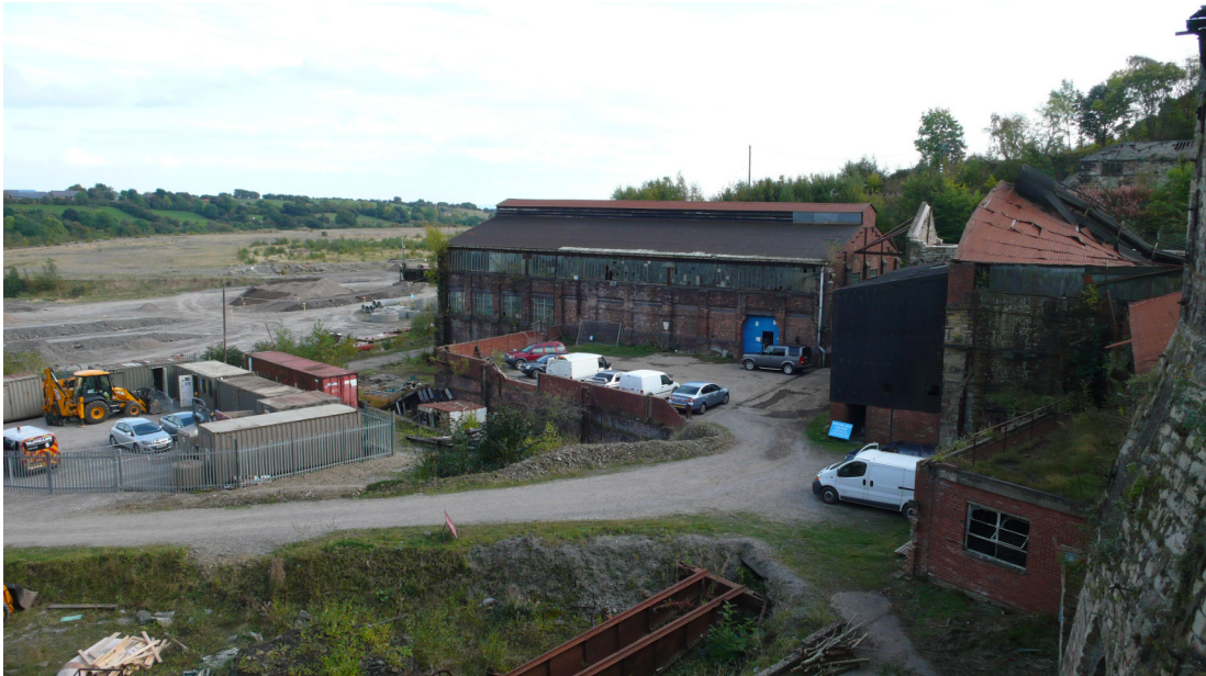
North elevation and existing car park
