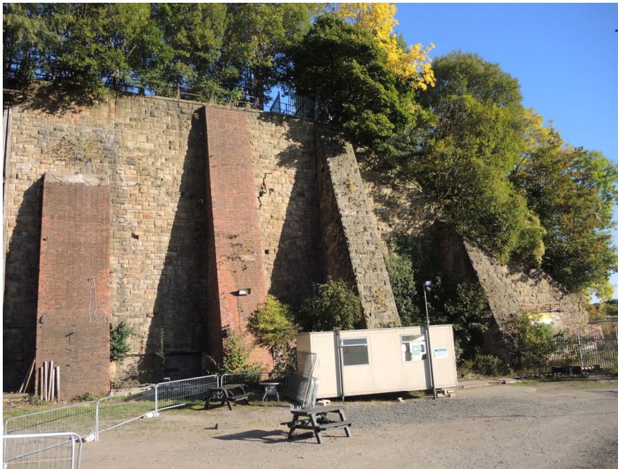
Charging Wall (North) image
