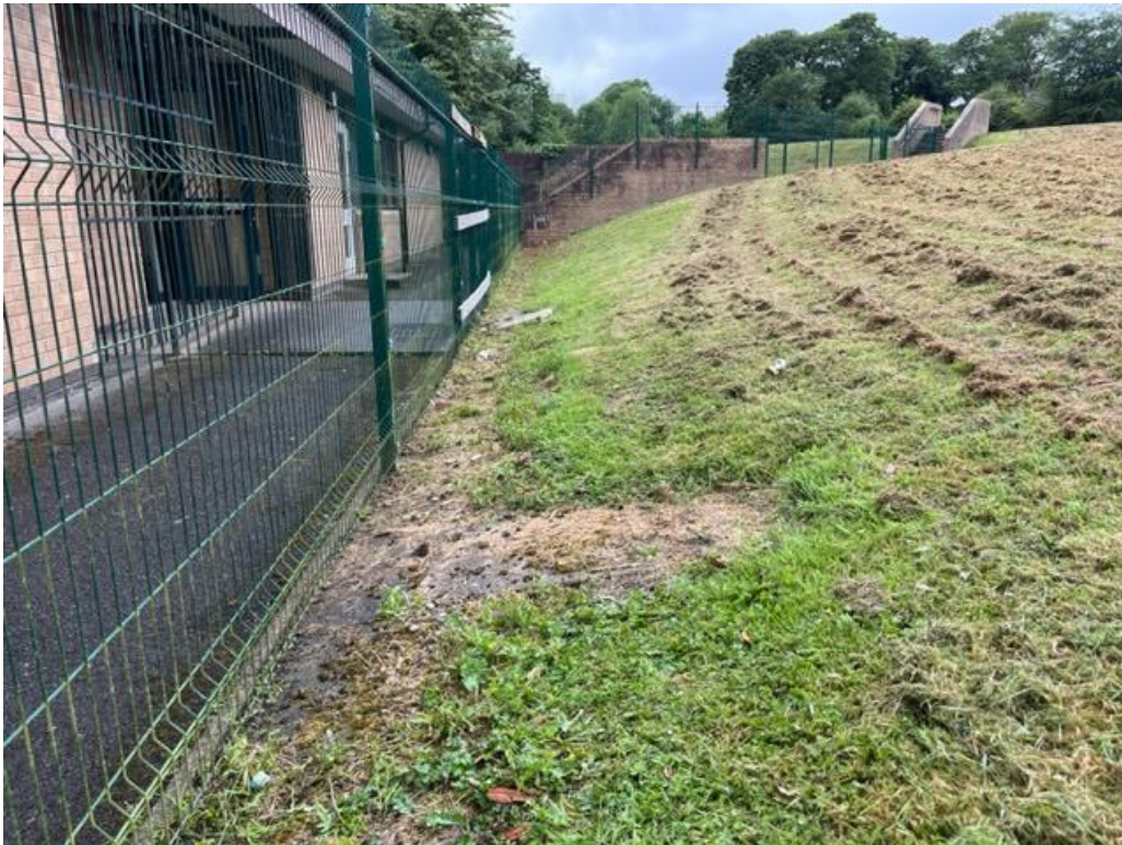
Existing security fence around the school
