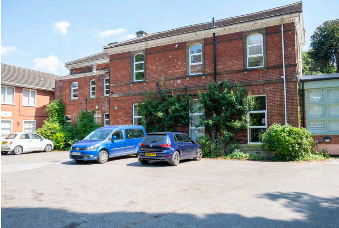
Photograph 8: The northern aspect of the house has less ornamentation. There are no pediments, and all of the windows are uPVC.
