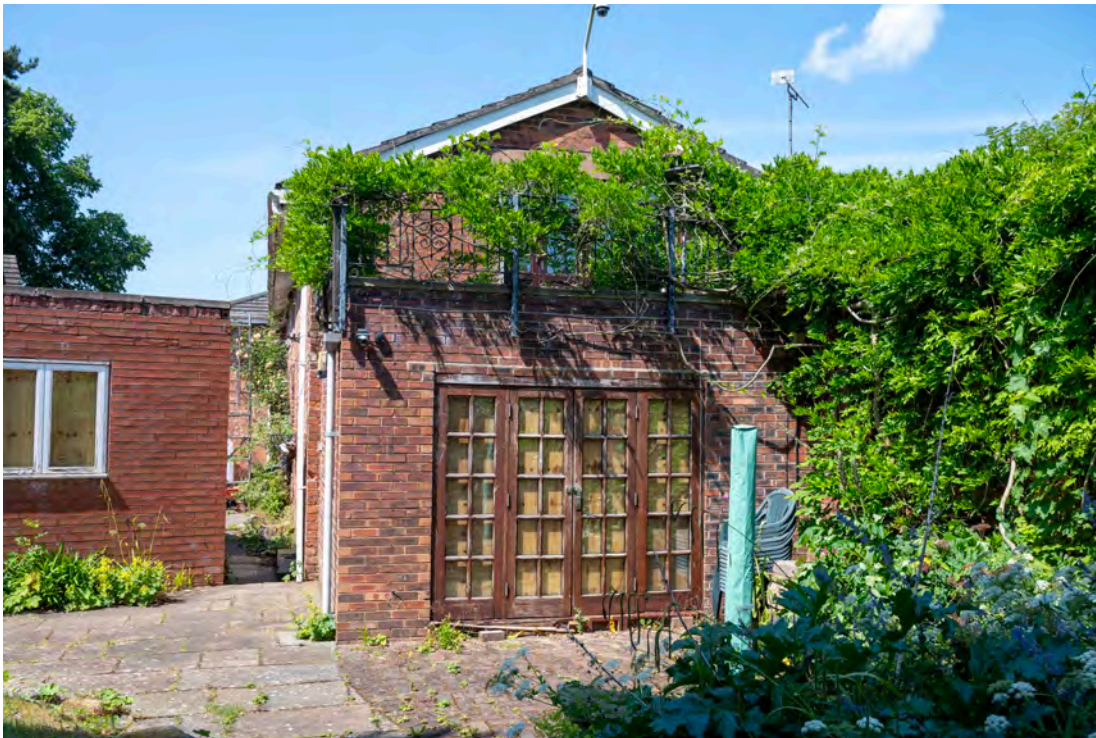
Photograph 13: The southern end of the coach house was watched on two occasions. There was no indication that bats were entering or leaving the building.
