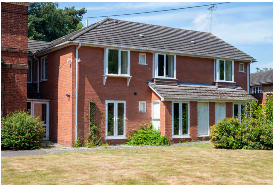
Photograph 10: The modern extension (Building 2) is in good decorative condition and has uPVC windows.
