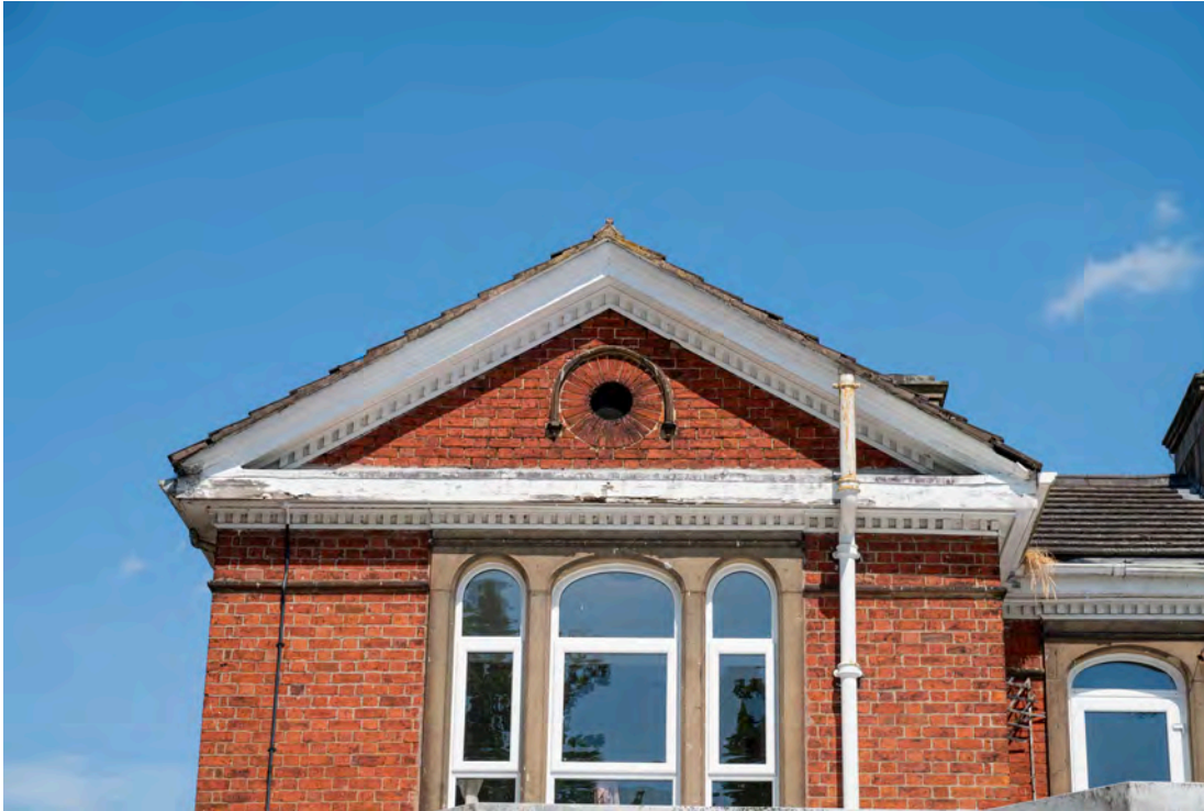
Photograph 4: The building was surveyed on three occasions. Bats were seen to enter and leave the tympanum on the south-western aspect of the house.
