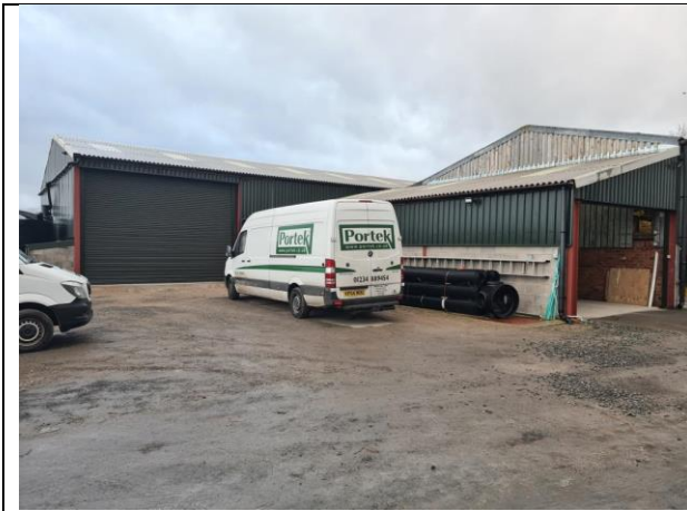
The site. Lean-to removed and replaced.
