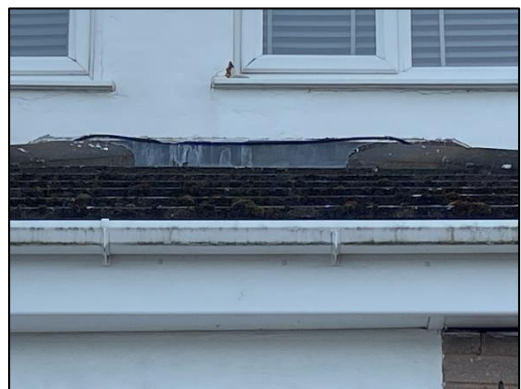
Photograph 8 showing the lead flashing
