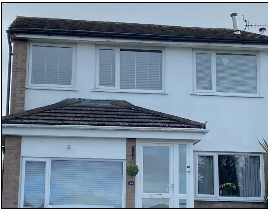
Photograph 1 showing the front facing elevation of the property
