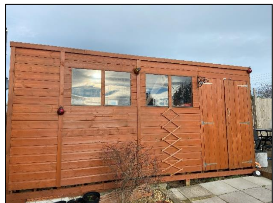
Photograph 12 showing the front elevation of the shed
