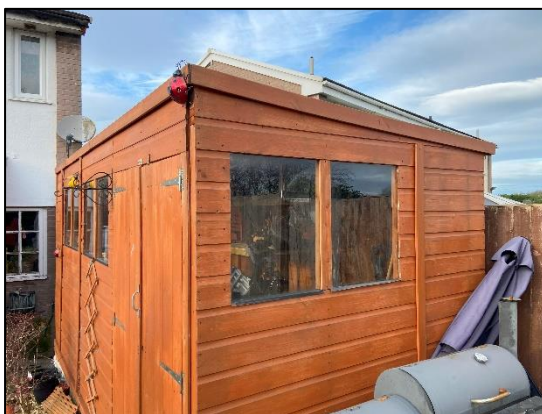
Photograph 11 showing the shed looking west
