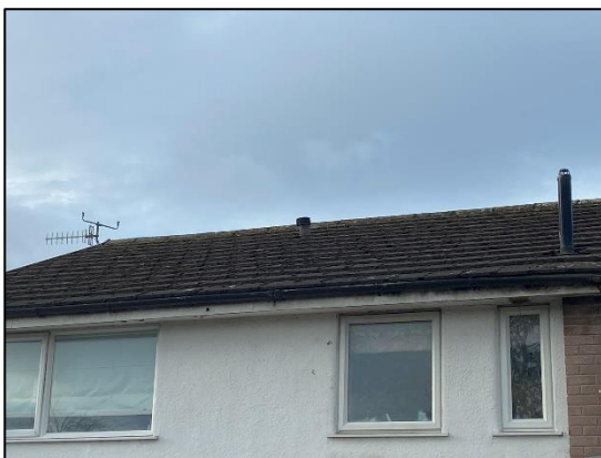
Photograph 3 showing the roof of the property
