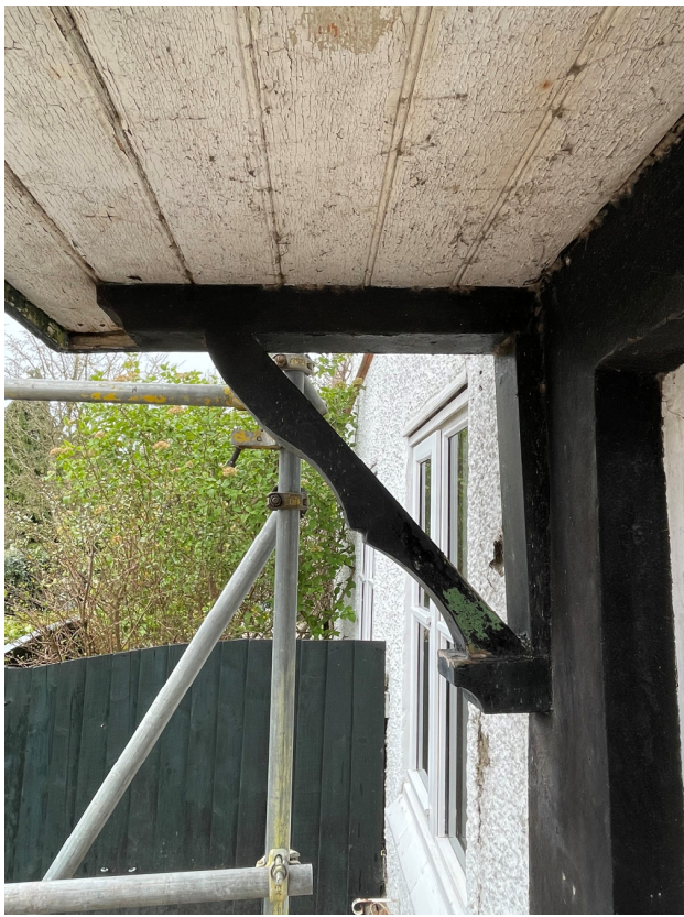
Existing timber canopy which is to be overhauled.
