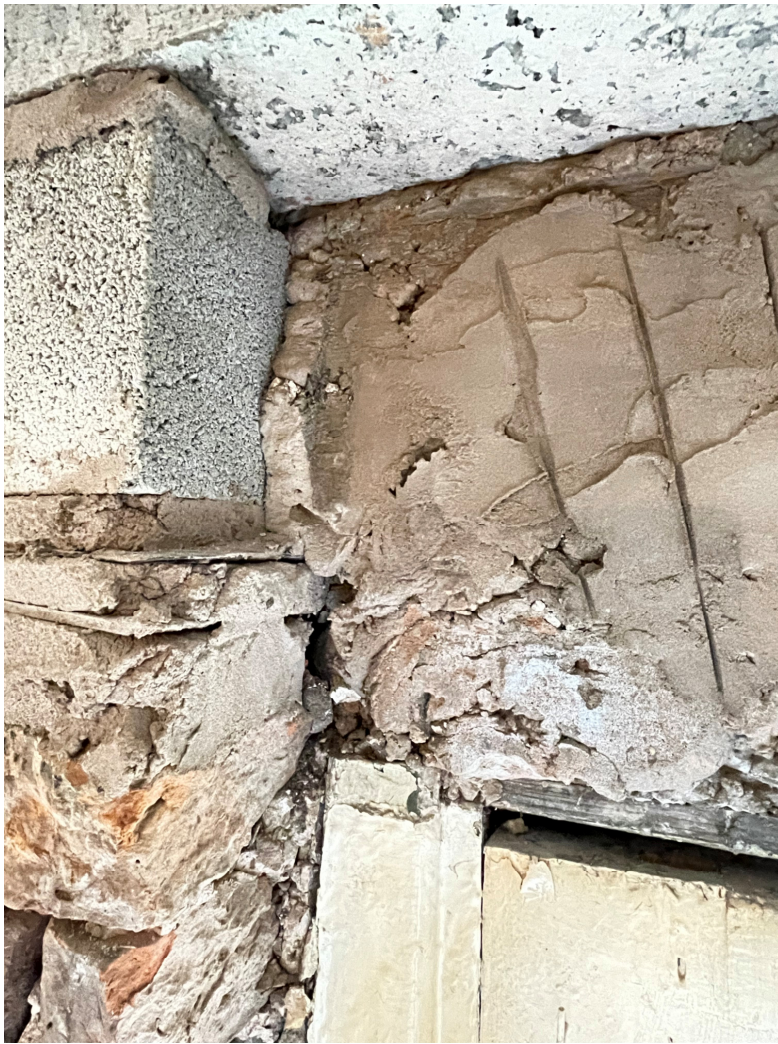
The existing door head which has been lowered and the door frame cut down.
