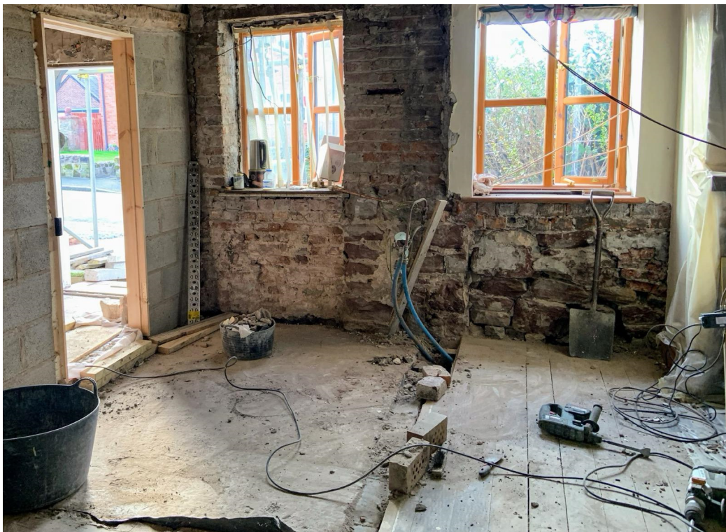
The exposed original doorway which has since been bricked up to form a window.
