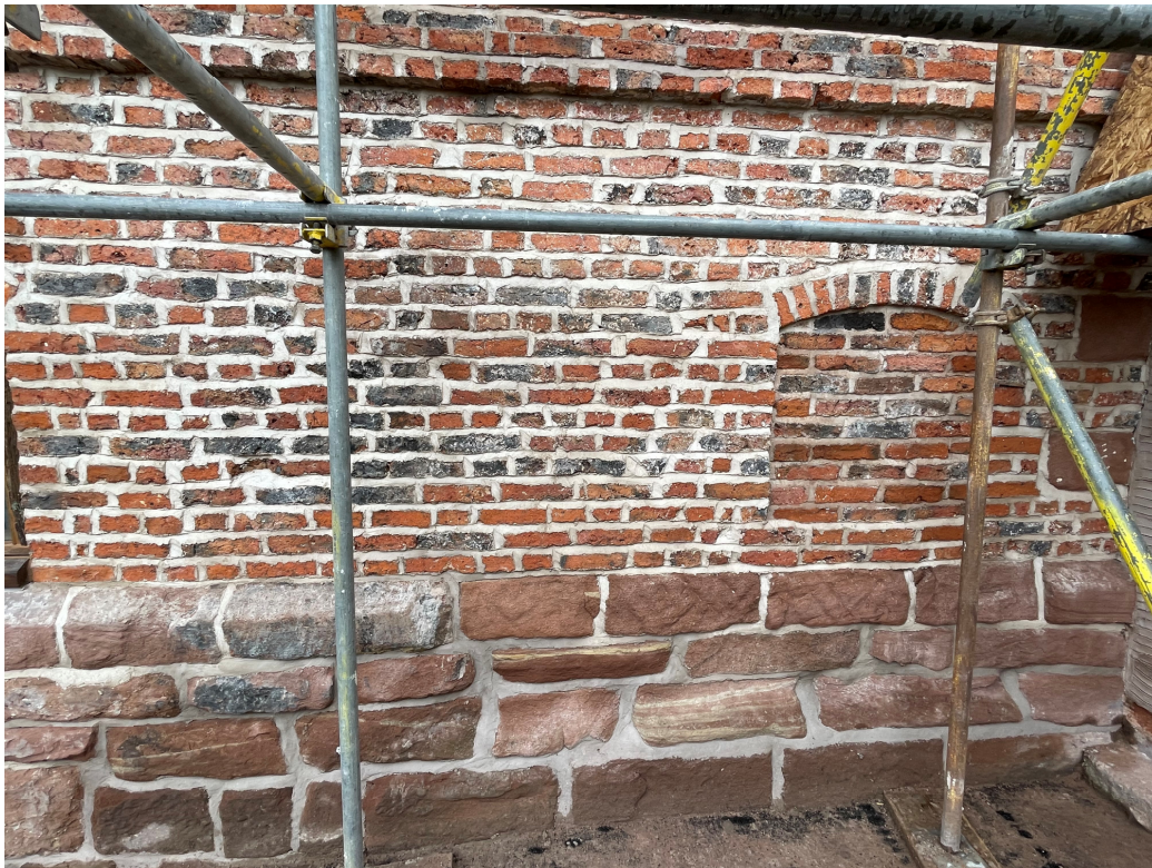
The existing inset window on the gable end.
