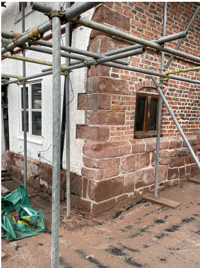
Original stone quoining that has now been exposed at the lower level and proposes to be exposed at first floor level.
