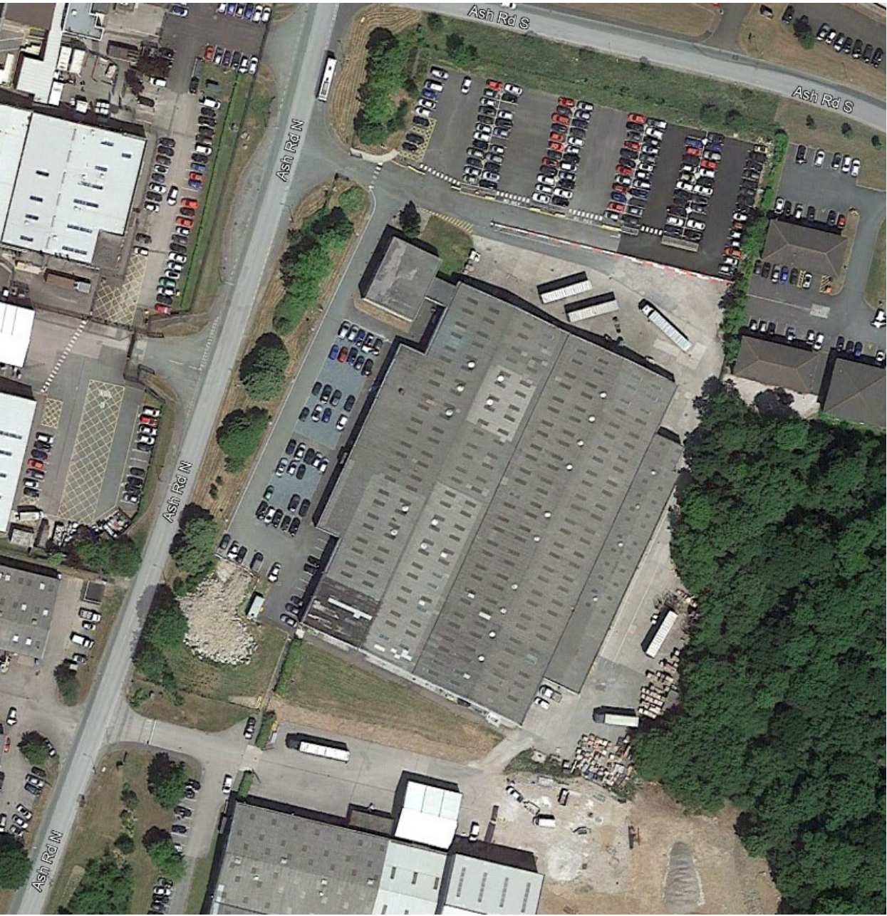
aerial photo in 2018, pre-demolition not to scale
