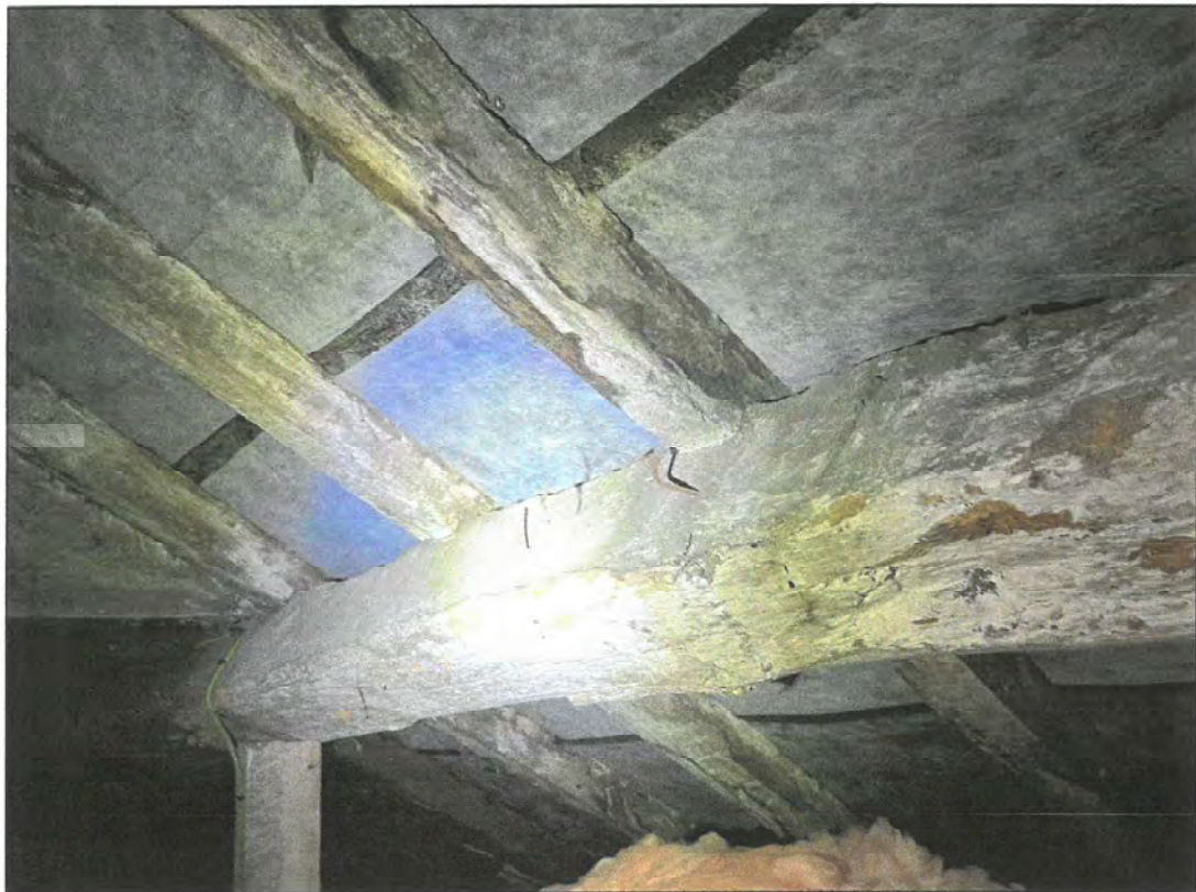
Plate 6 – Bitumen roof lining in loft space
