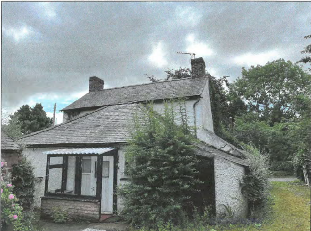
Plate 2 – Northern aspect of the house
