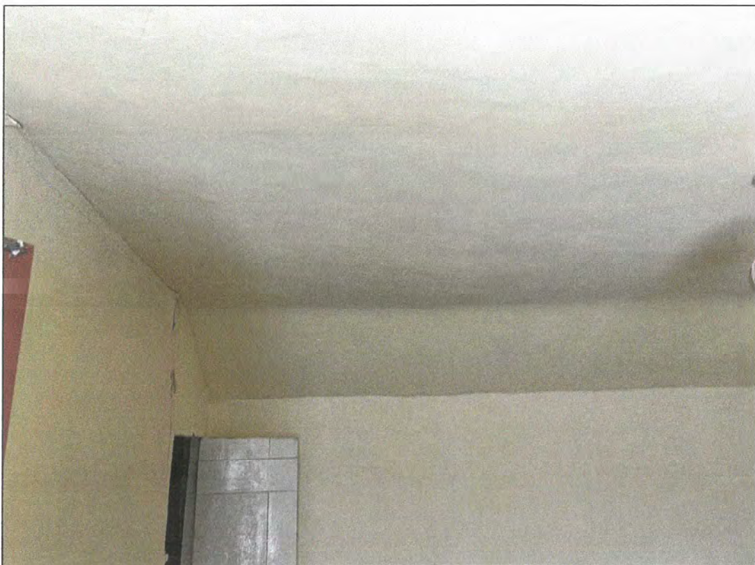
Plate 4 – Interior of the pitched roof section of the building
