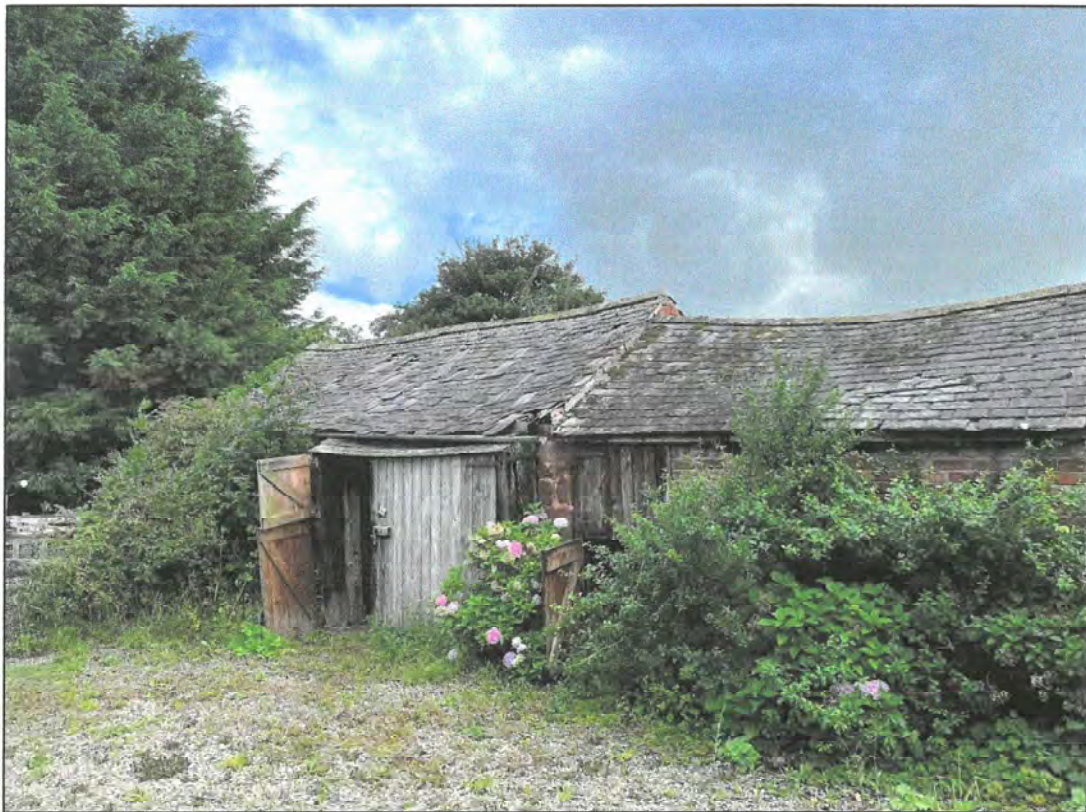
Plate 10 – The outbuilding as seen from the west
