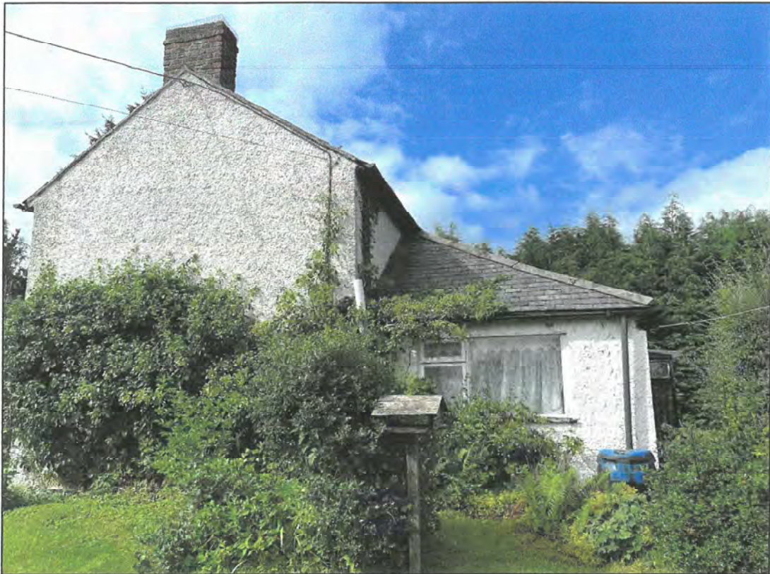
Plate 3 – The eastern elevation of the house
