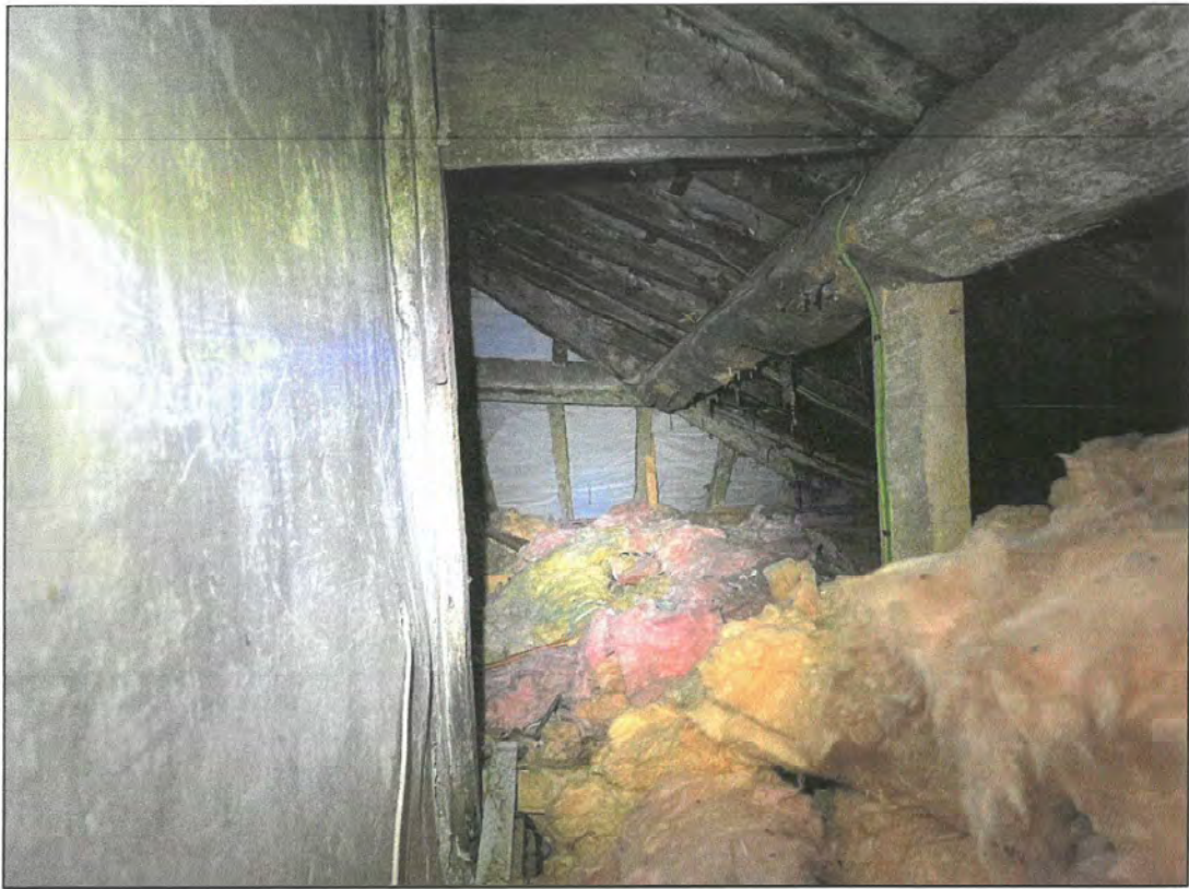
Plate 5 – Character of the loft void beneath the hipped roof section, with BRM evident at rear
