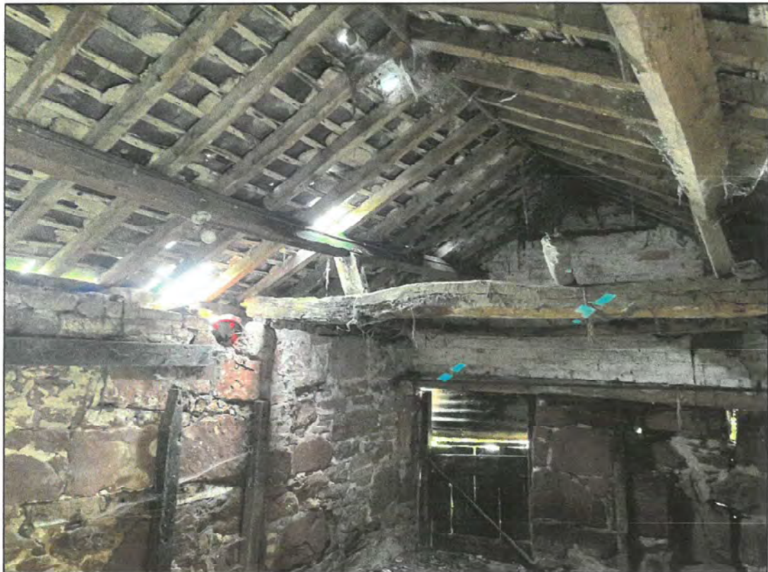
Plate 12 – Internal character of the outbuilding
