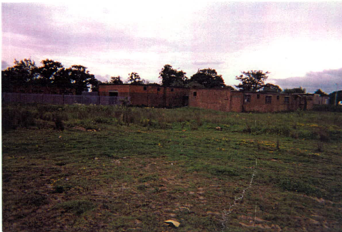
Plate 14 View from the North West to the South East showing the buildings within which radio active catalyst was previously stored.
