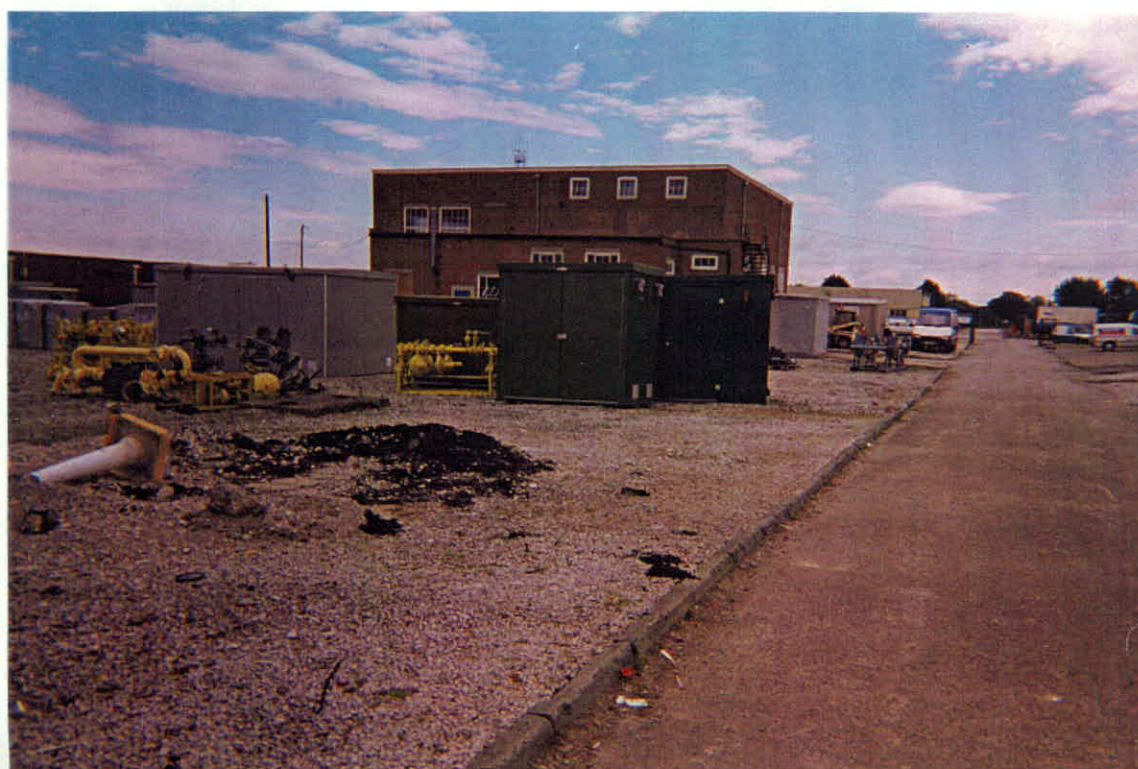
Plate 7. View looking from the West to the East showing the former location of the Wet Purification Plant, comprising the Detarrer and Static Scrubbers. Beneath this gravel area lay the tar and liquor tanks. It is not known if they have been removed.
