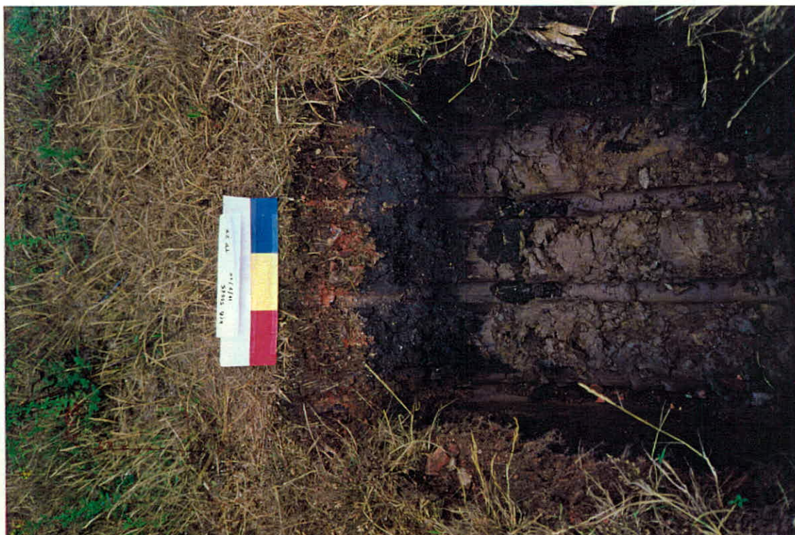
PLATE 35: Trial Pit TP 28. Showing clay below fill materials.
