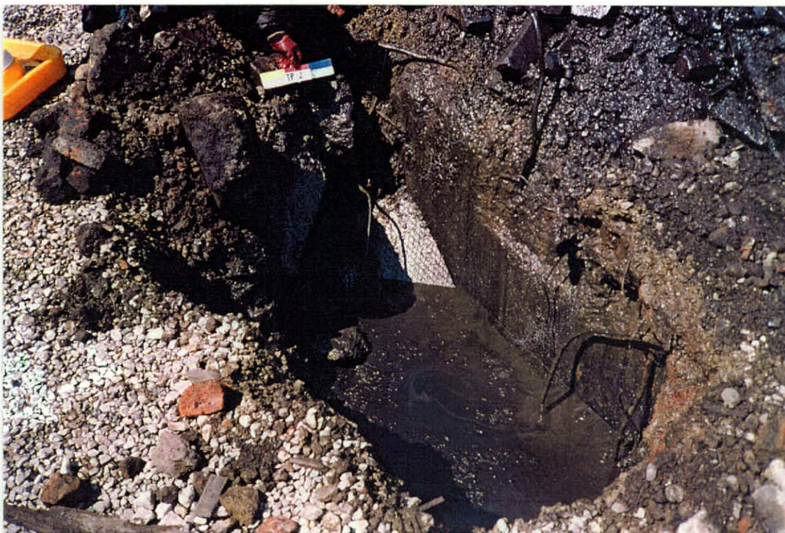
PLATE 26: Trial Pit TP21. Dug into an underground tank in the vicinity of the tar separator next to the CWG Plant.
