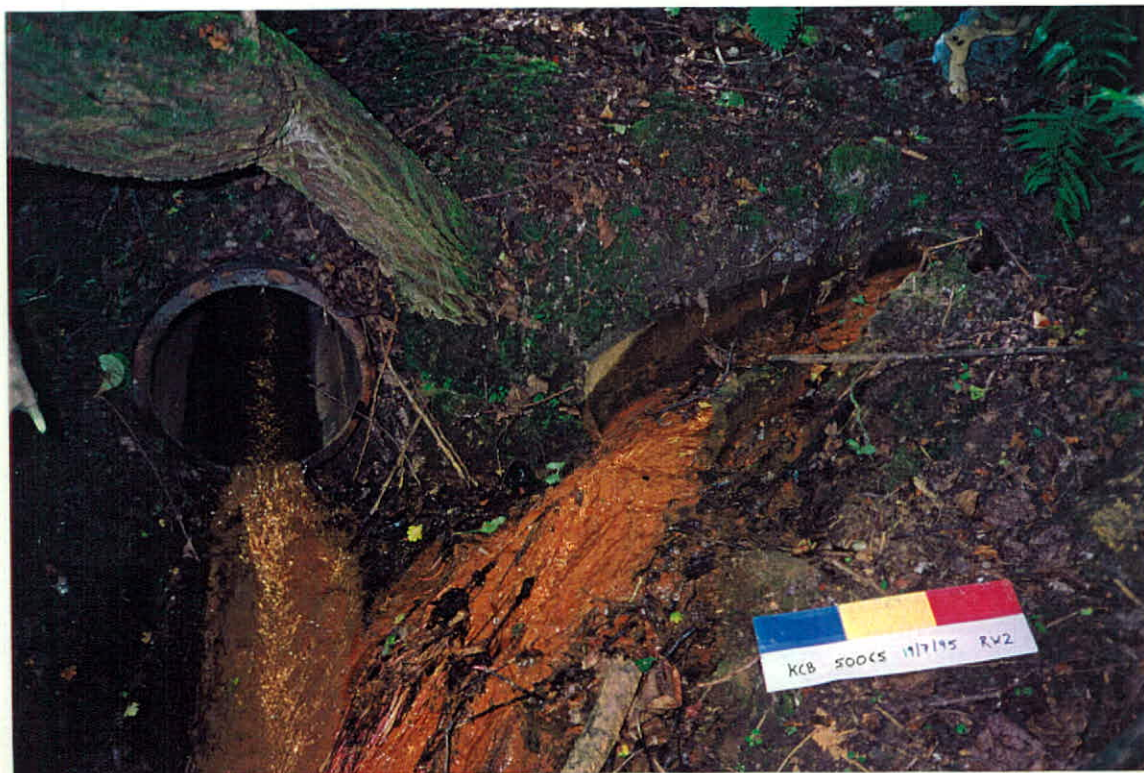
PLATE 39: Storm drain outfalls into the stream in the southeast of the site. Sample collection point RW 2.
