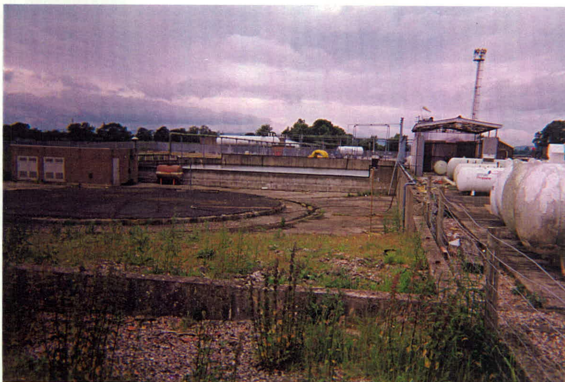
Plate 11. View looking from the east to the West showing the former location of the LDF Storage Tanks. The secondary containment of the furthest tank is now used as a lagoon for the storage of sprinkler water.
