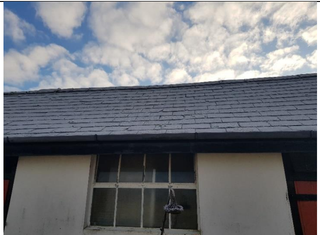
Slate roof and clay ridge on stable block.
