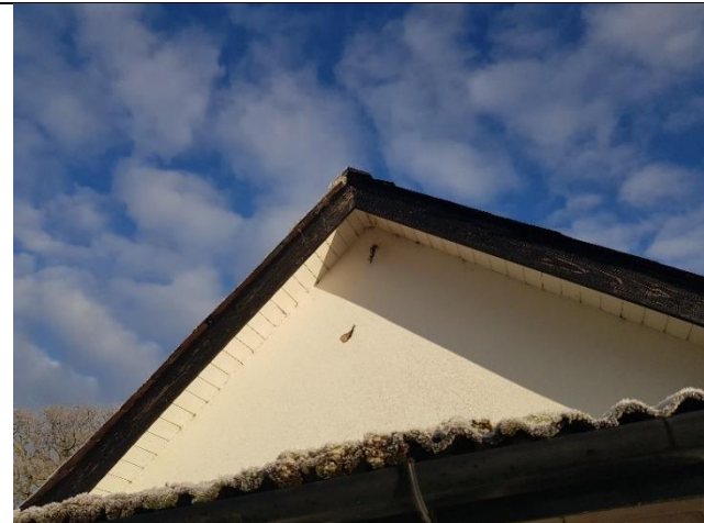
Gable ends sealed and eaves boxed in with timber soffits.
