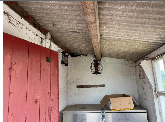
Interior of single storey lean-to at south gable.
