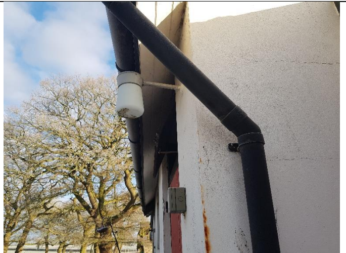
Eaves around the stable block are sealed with timber soffits.
