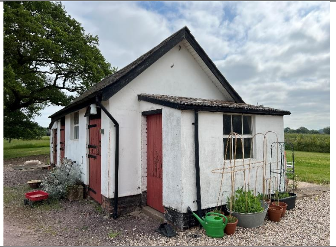
Stable block to be removed.
