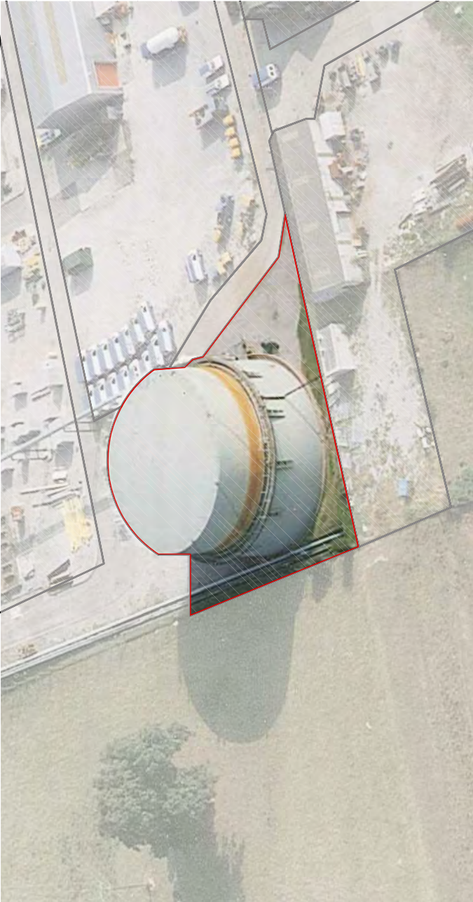
Gas holder - highlighted aerial image
