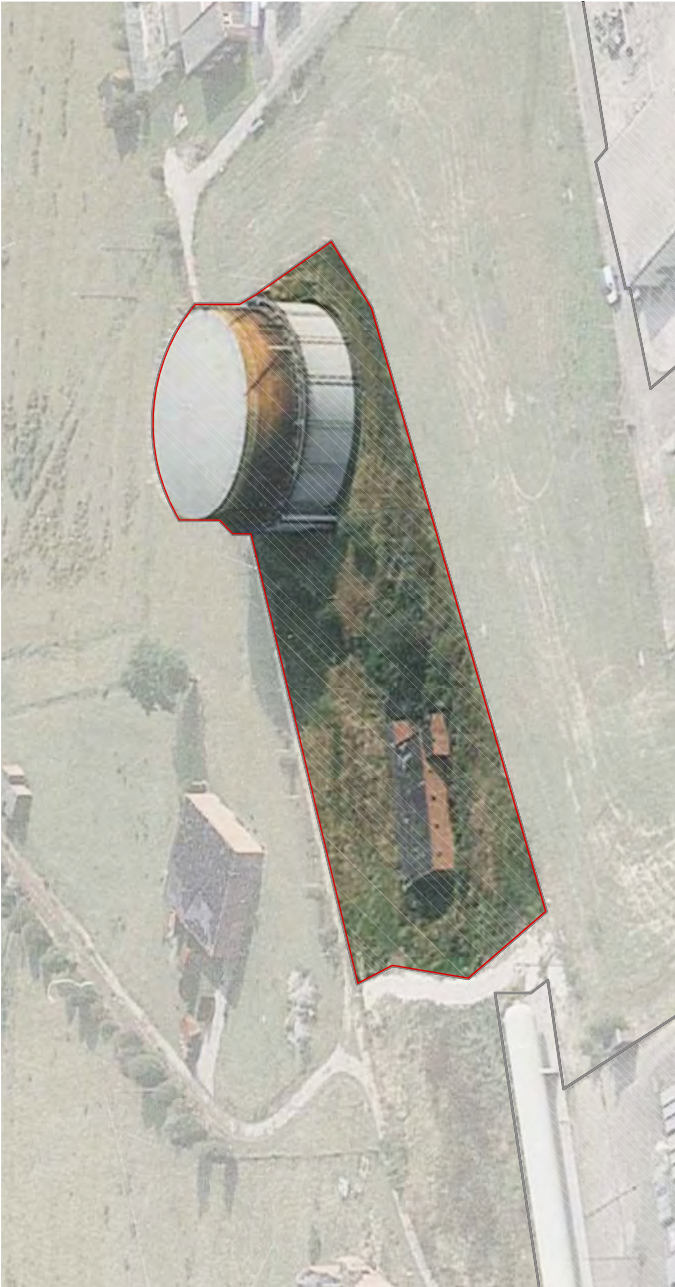
Gas holder and paint store - highlighted aerial image
