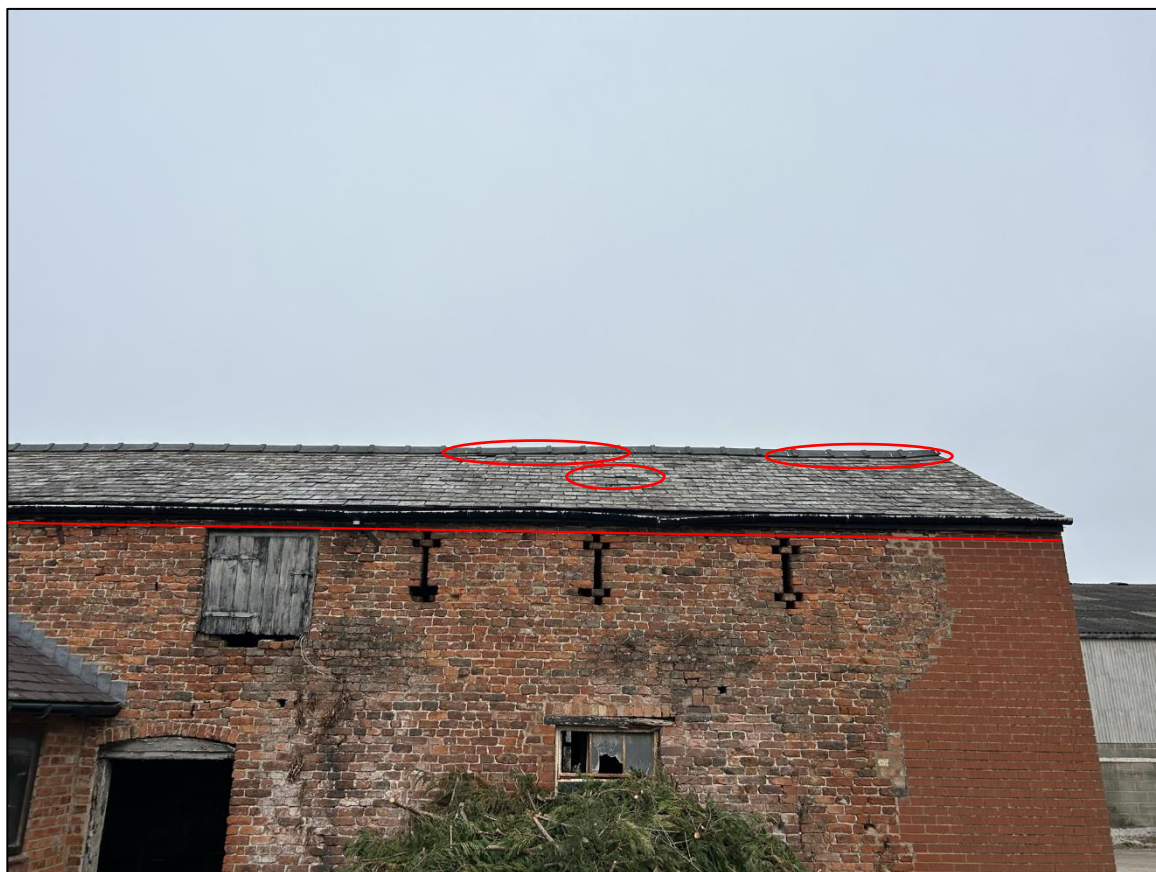
Plate 5 – PRFs on southern elevation
