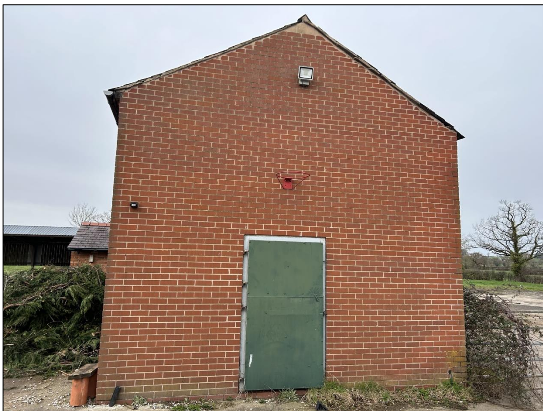
Plate 2 – The eastern aspect of the building
