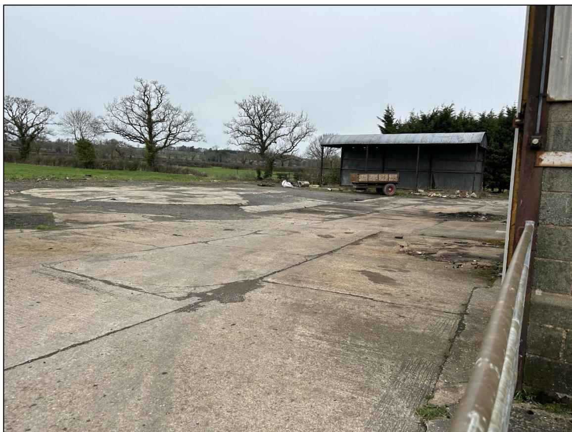
Plate 12 – Nature of the hardstanding surrounding site
