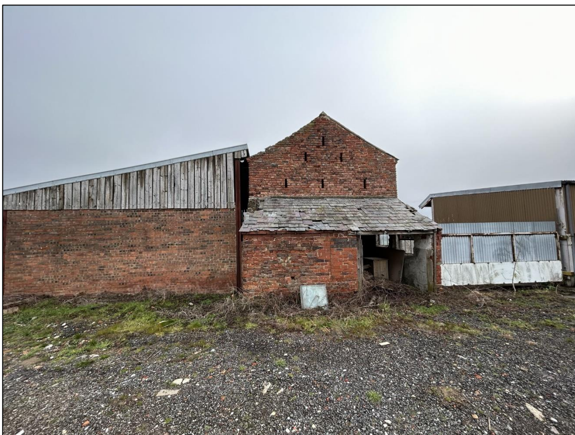
Plate 4 – The western aspect, with airbricks visible
