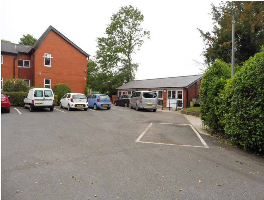
Photograph 7: View of hard standing to south of site and associated with current parking provision.
