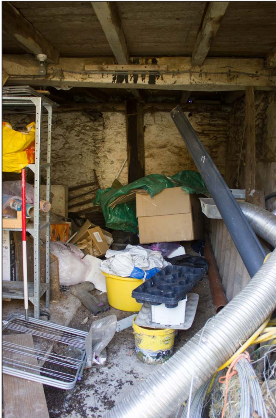
Plate 20: Ground floor storage room of Outbuilding at Tŷ Mawr, Pontfadog, Llangollen, Wrexham - from the north - 1.00m scale
