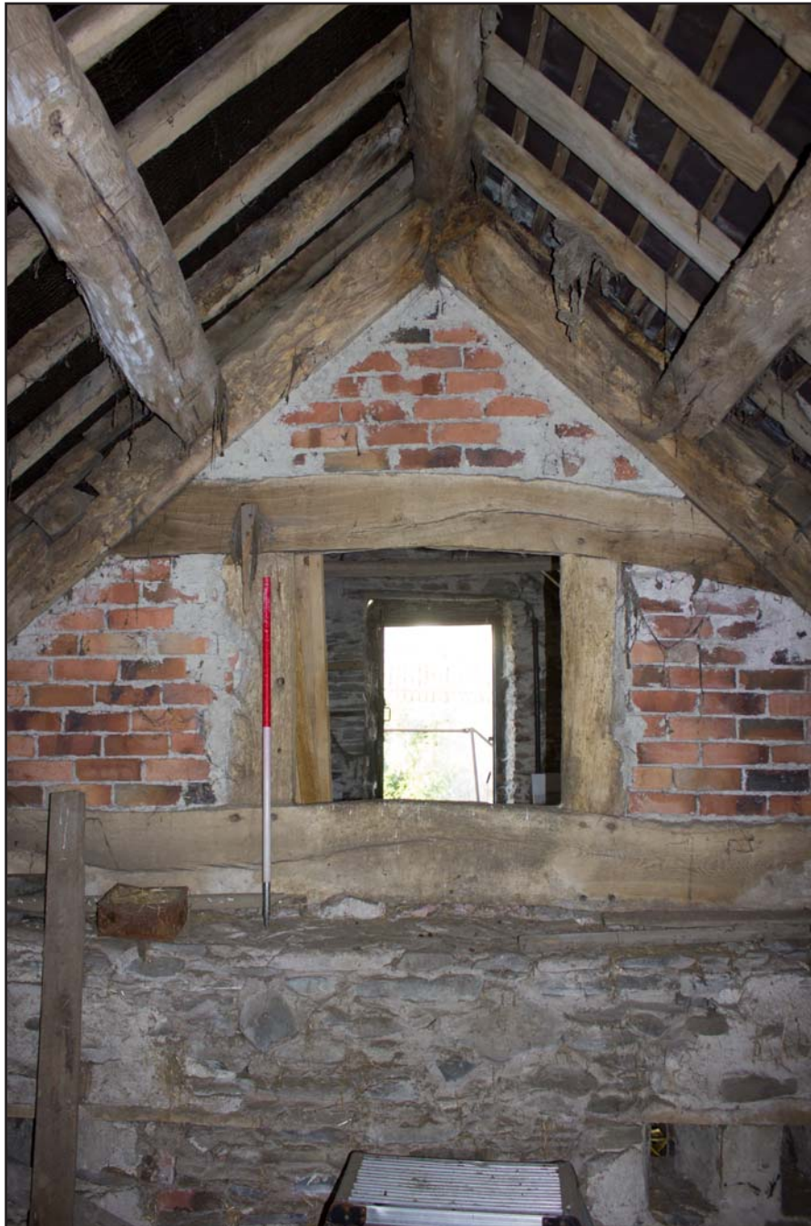
Plate 34: Brick infilled truss between, 1st Floor storage room and the Hayloft within Outbuilding at Tŷ Mawr, Pontfadog, Llangollen, Wrexham - from the east - 1.00m scale
