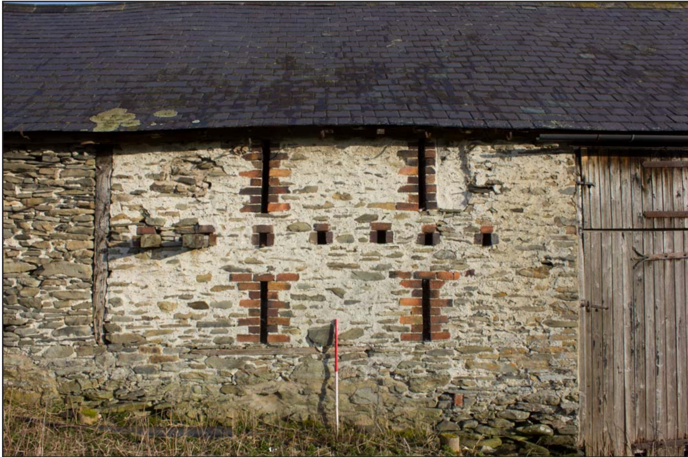
Plate 16: Ventilation embrasure slots in southern elevation of Outbuilding at Tŷ Mawr, Pontfadog, Llangollen, Wrexham - from the south - 1.00m scale
