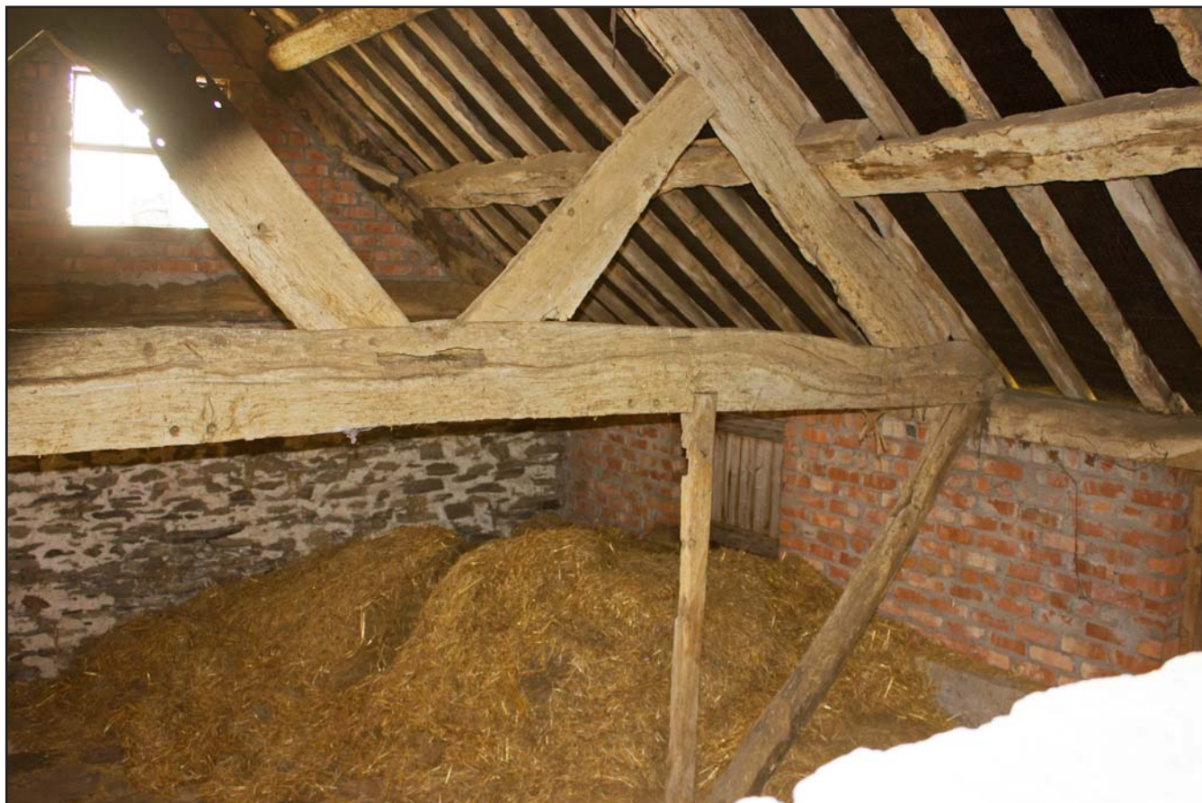
Plate 38: Eastern end of hayloft within Outbuilding at Tŷ Mawr, Pontfadog, Llangollen, Wrexham - from the northwest - no scale
