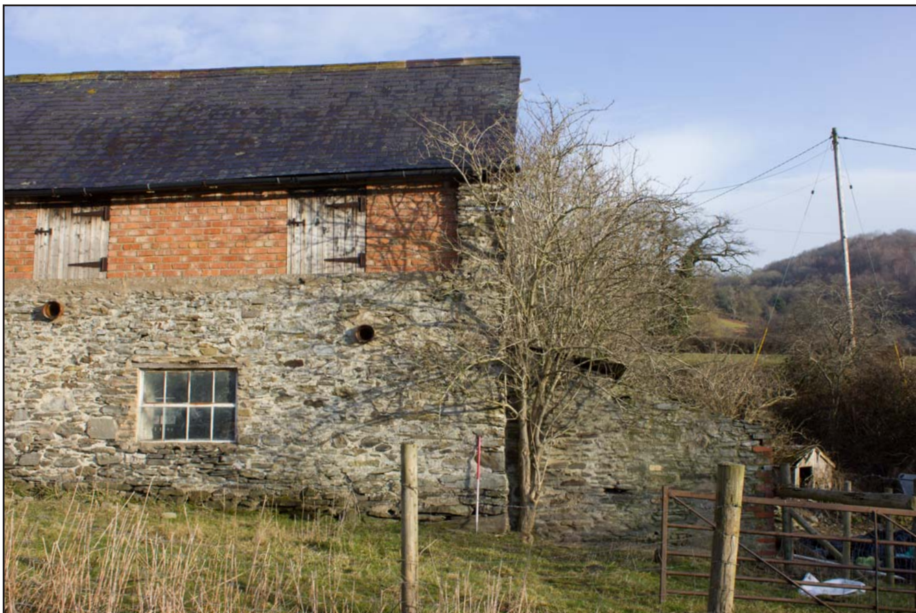
Plate 12: Southern elevation (right) of Outbuilding at Tŷ Mawr, Pontfadog, Llangollen, Wrexham - from the south - 1.00m scale
