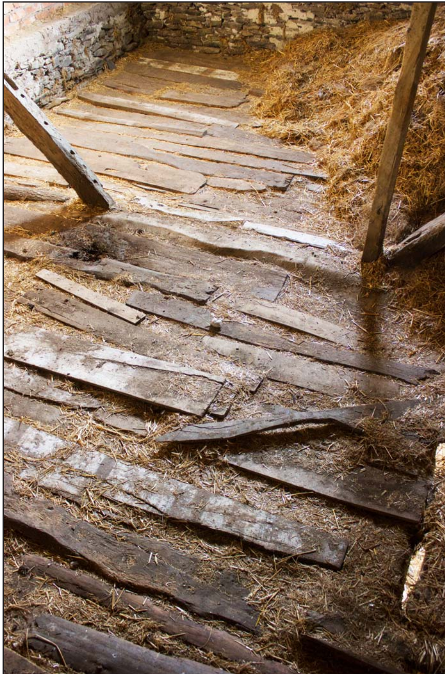
Plate 40: Floor at eastern end of hayloft within Outbuilding at Tŷ Mawr, Pontfadog, Llangollen, Wrexham - from the southwest - no scale
