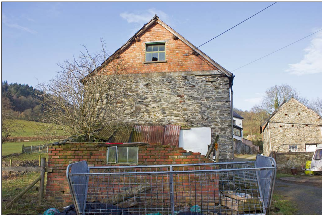
Plate 10: Eastern elevation of Outbuilding at Tŷ Mawr, Pontfadog, Llangollen, Wrexham - from the east - 1.00m scale
