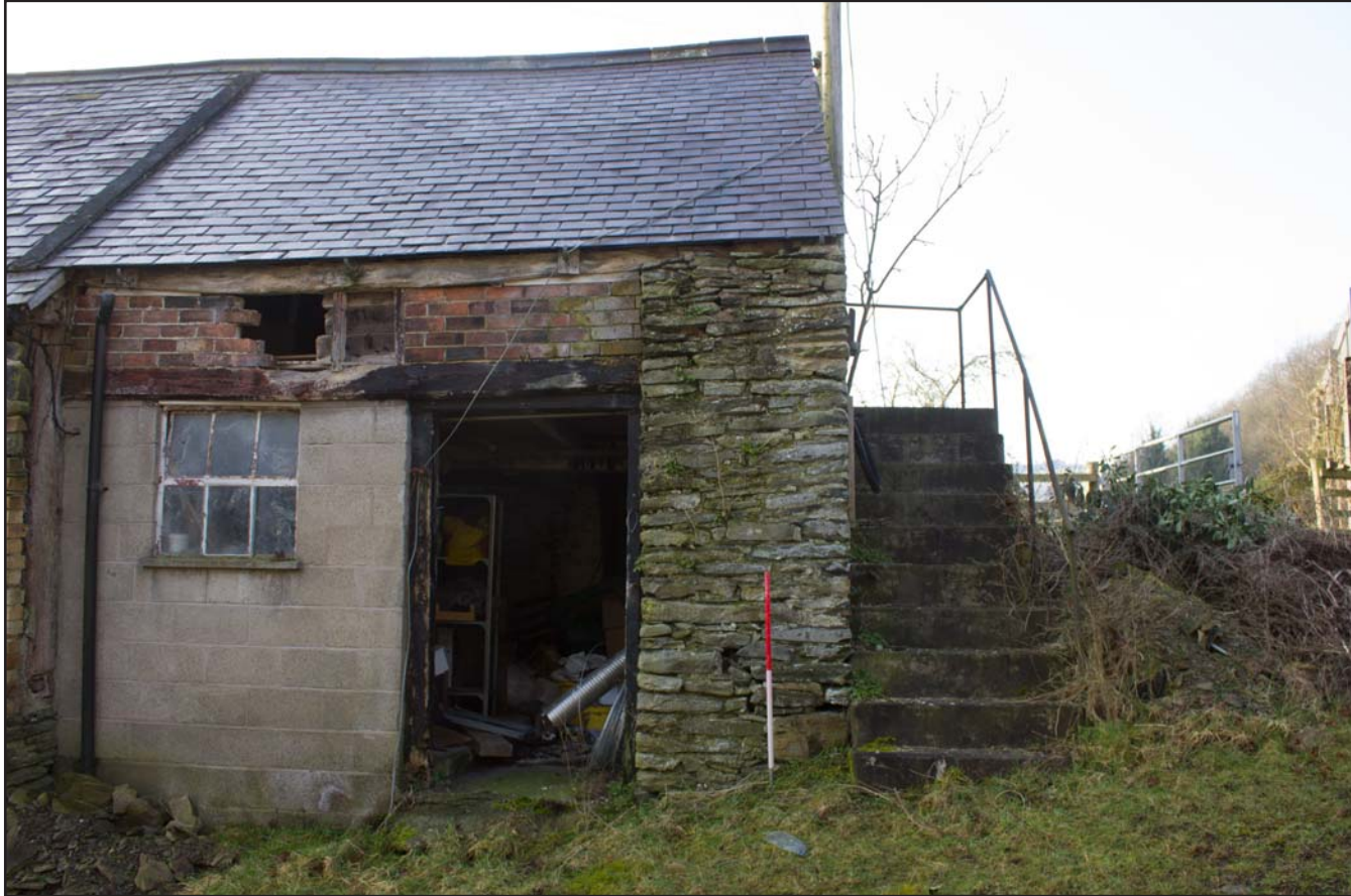
Plate 06: Northern elevation (right) of Outbuilding at Tŷ Mawr, Pontfadog, Llangollen, Wrexham - from the north - 1.00m scale
