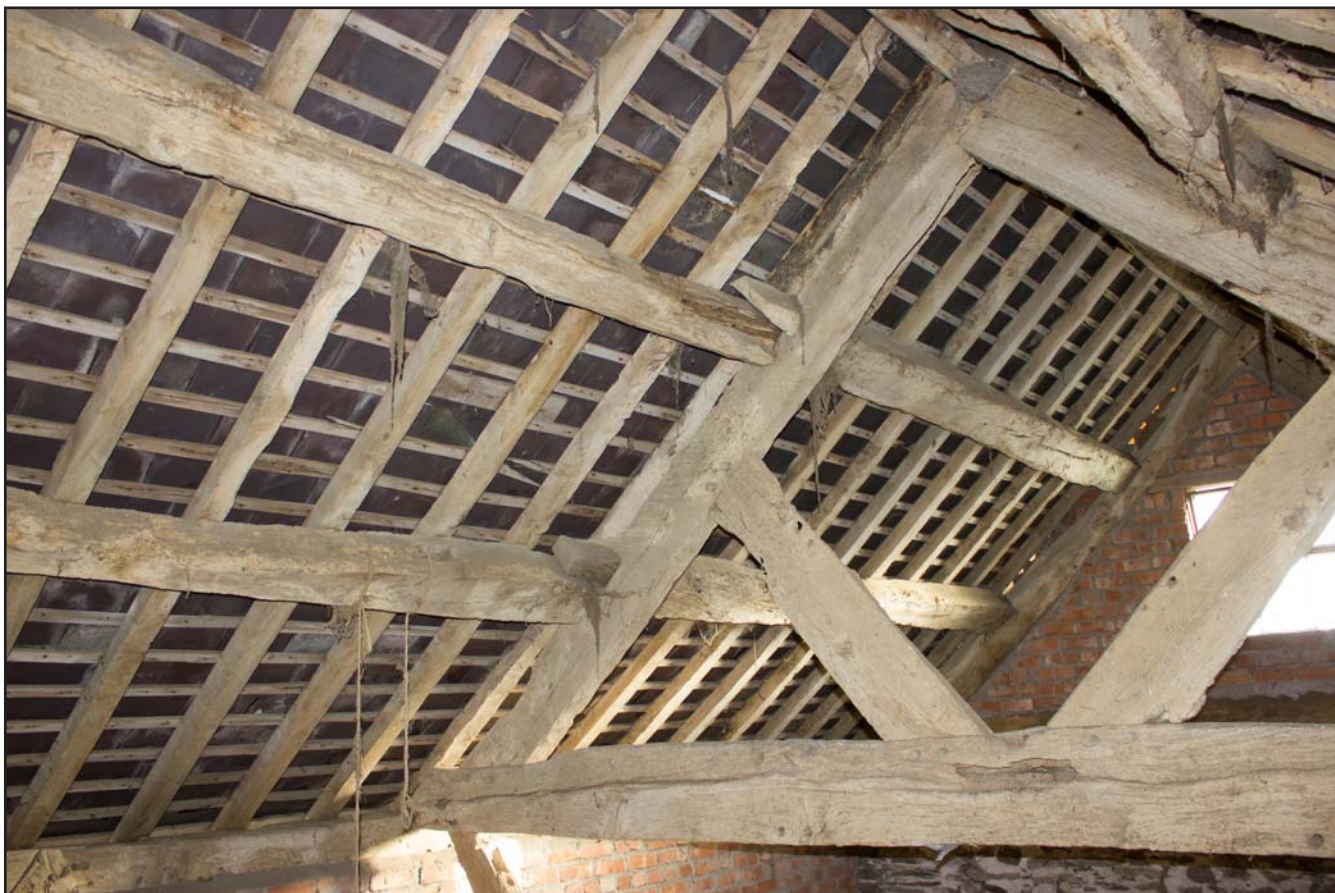
Plate 41: Ceiling construction at eastern end of hayloft within Outbuilding at Tŷ Mawr, Pontfadog, Llangollen, Wrexham - from the southwest - no scale
