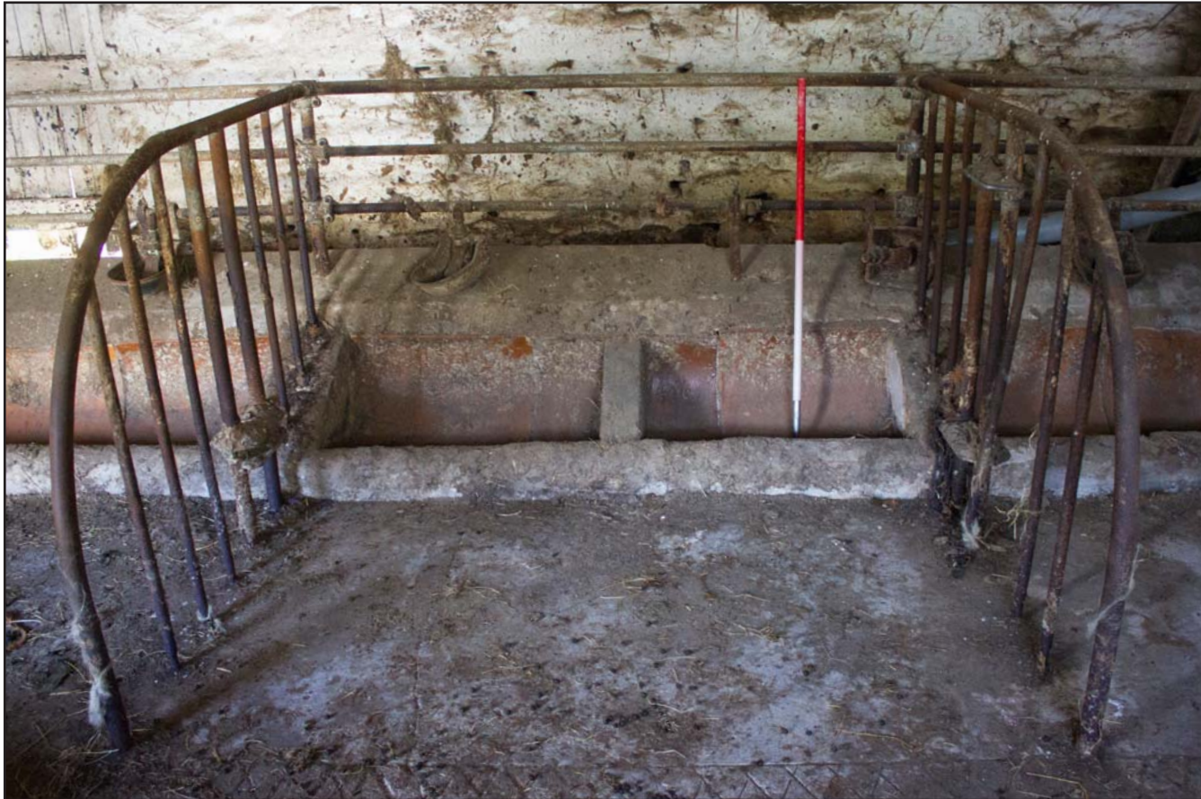
Plate 23: Milking Parlour, cattle stall, within Outbuilding at Tŷ Mawr, Pontfadog, Llangollen, Wrexham - from the north - 1.00m scale
