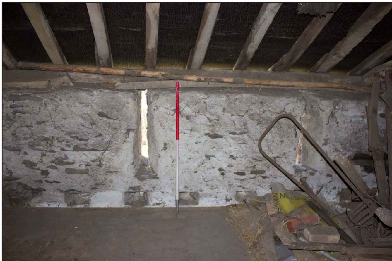
Plate 42: Embrasure ventilation slots in southern elevation of Hayloft at Tŷ Mawr, Pontfadog, Llangollen, Wrexham - from the north - 1.00m scale
