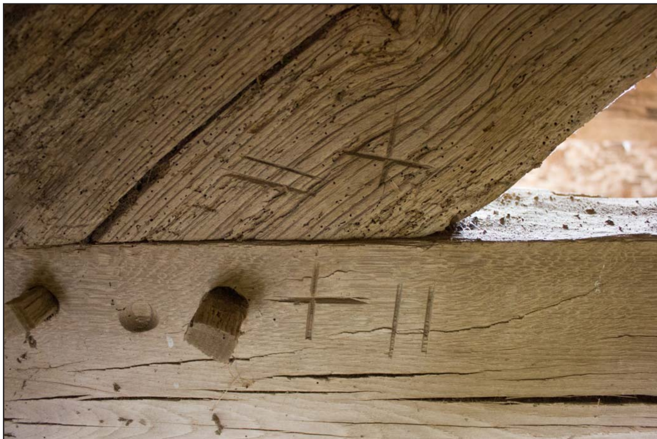
Plate 44: Carpenter's marks and dowel joint reinforcement on trusses in Hayloft Outbuilding at Tŷ Mawr, Pontfadog, Llangollen, Wrexham - from the west - no scale
