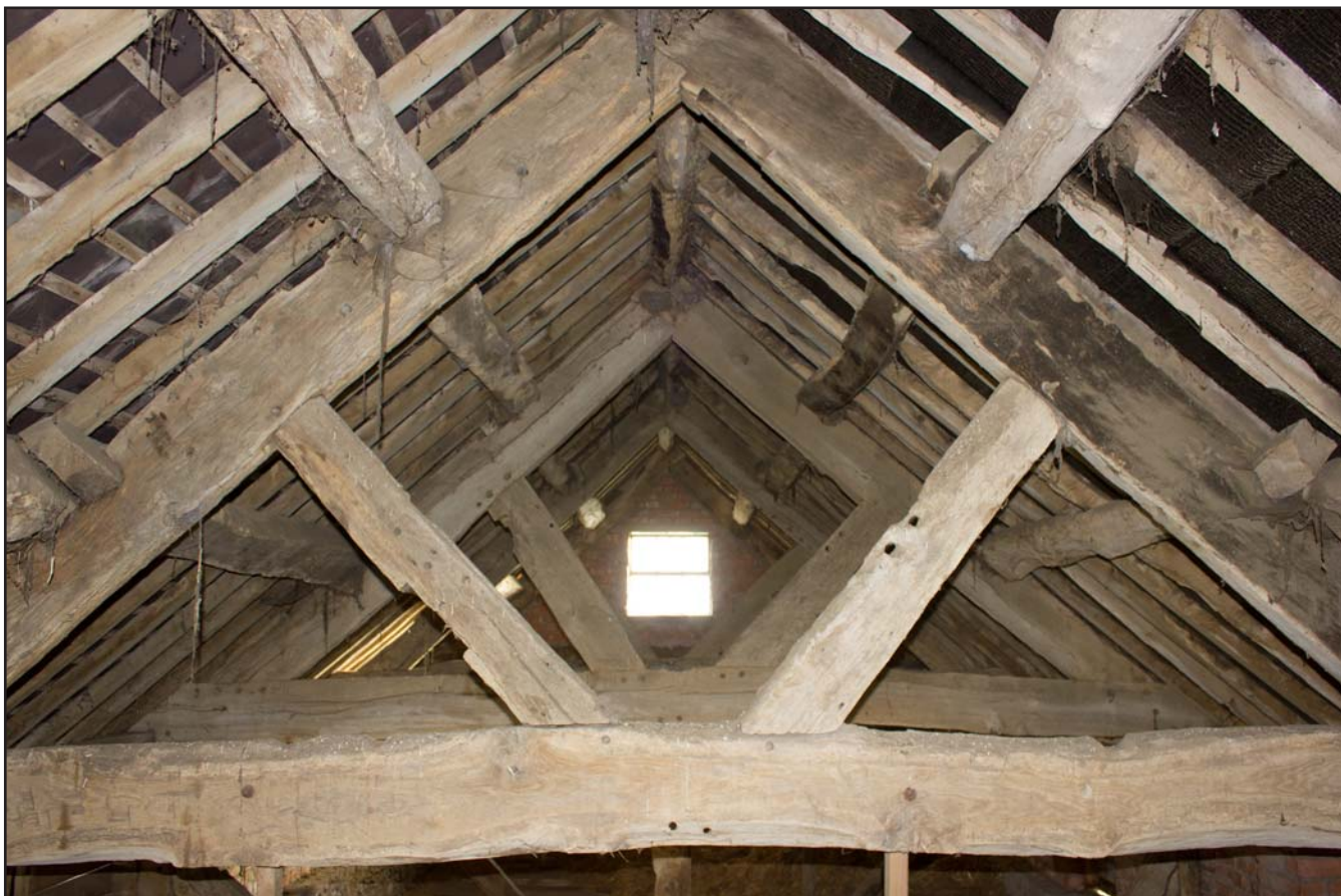
Plate 36: Collar tie beam trusses with raking struts within the Hayloft inside the Outbuilding at Tŷ Mawr, Pontfadog, Llangollen, Wrexham - from the west - no scale
