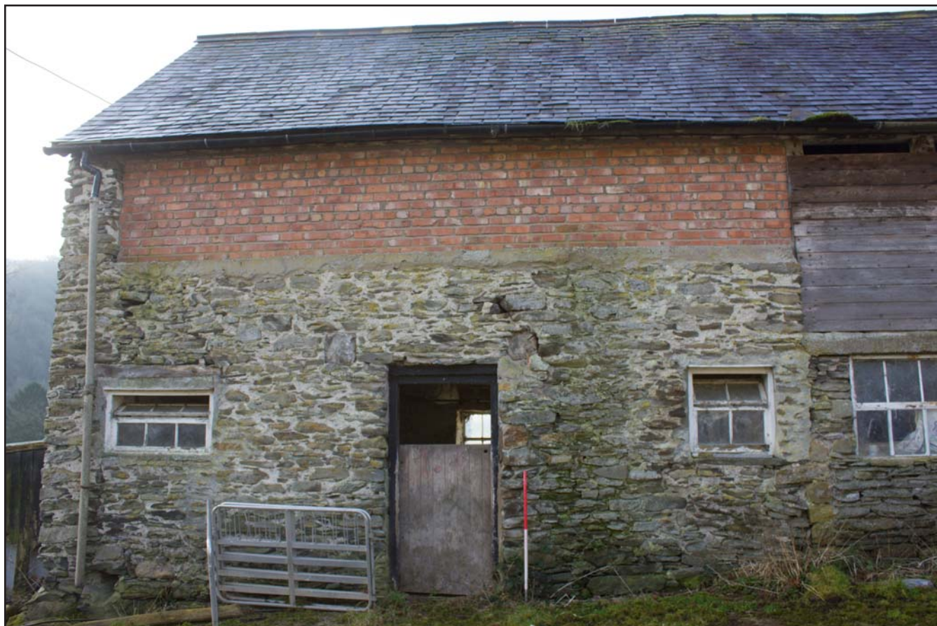
Plate 08: Northern elevation (left) of Outbuilding at Tŷ Mawr, Pontfadog, Llangollen, Wrexham - from the north - 1.00m scale
