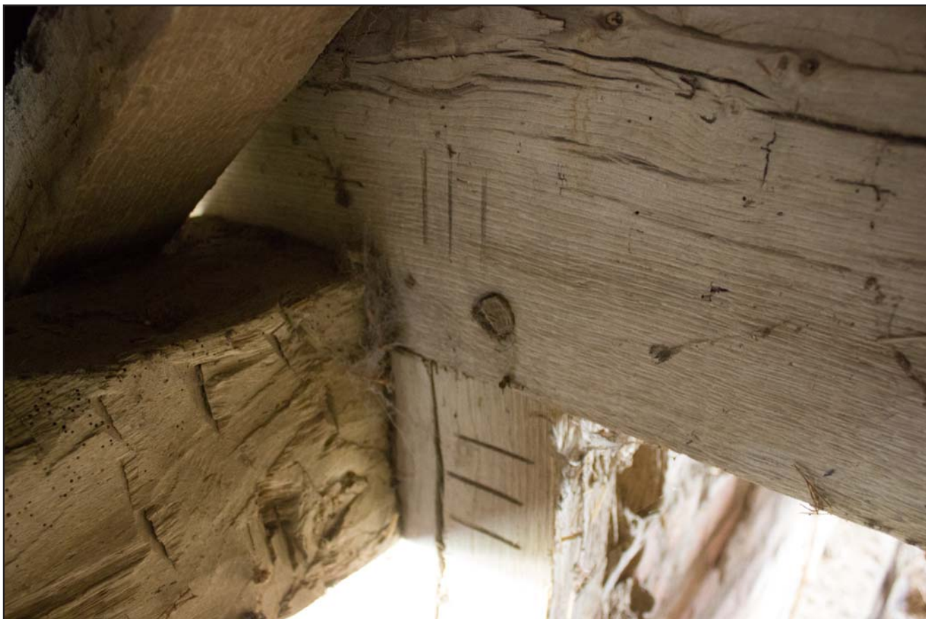
Plate 46: Carpenter's marks and dowel joint reinforcement on trusses in Hayloft Outbuilding at Tŷ Mawr, Pontfadog, Llangollen, Wrexham - from the southeast - no scale
