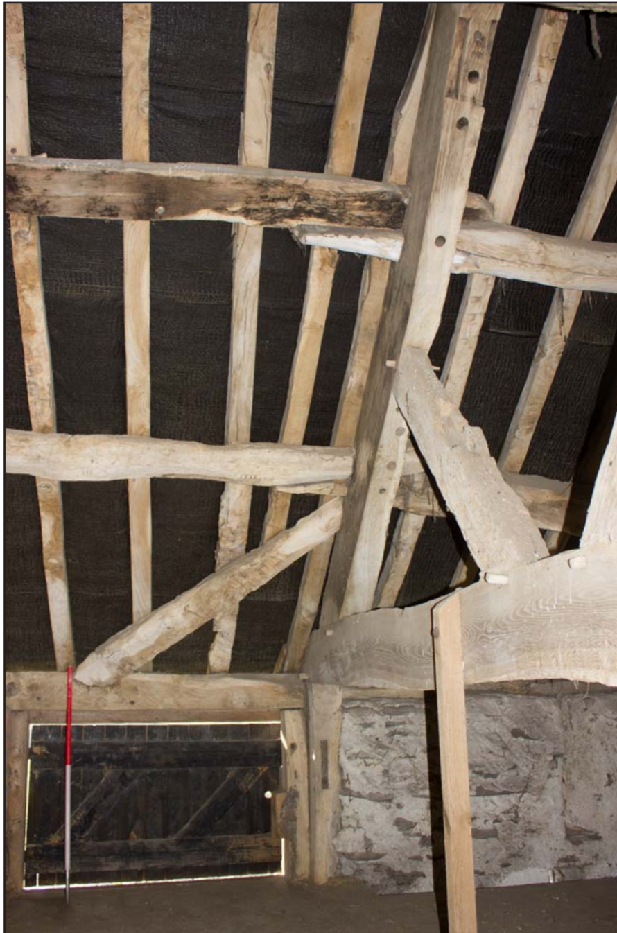
Plate 37: Side strut or wind brace in Hayloft roof of Outbuilding at Tŷ Mawr, Pontfadog, Llangollen, Wrexham - from the north - 1.00m scale
