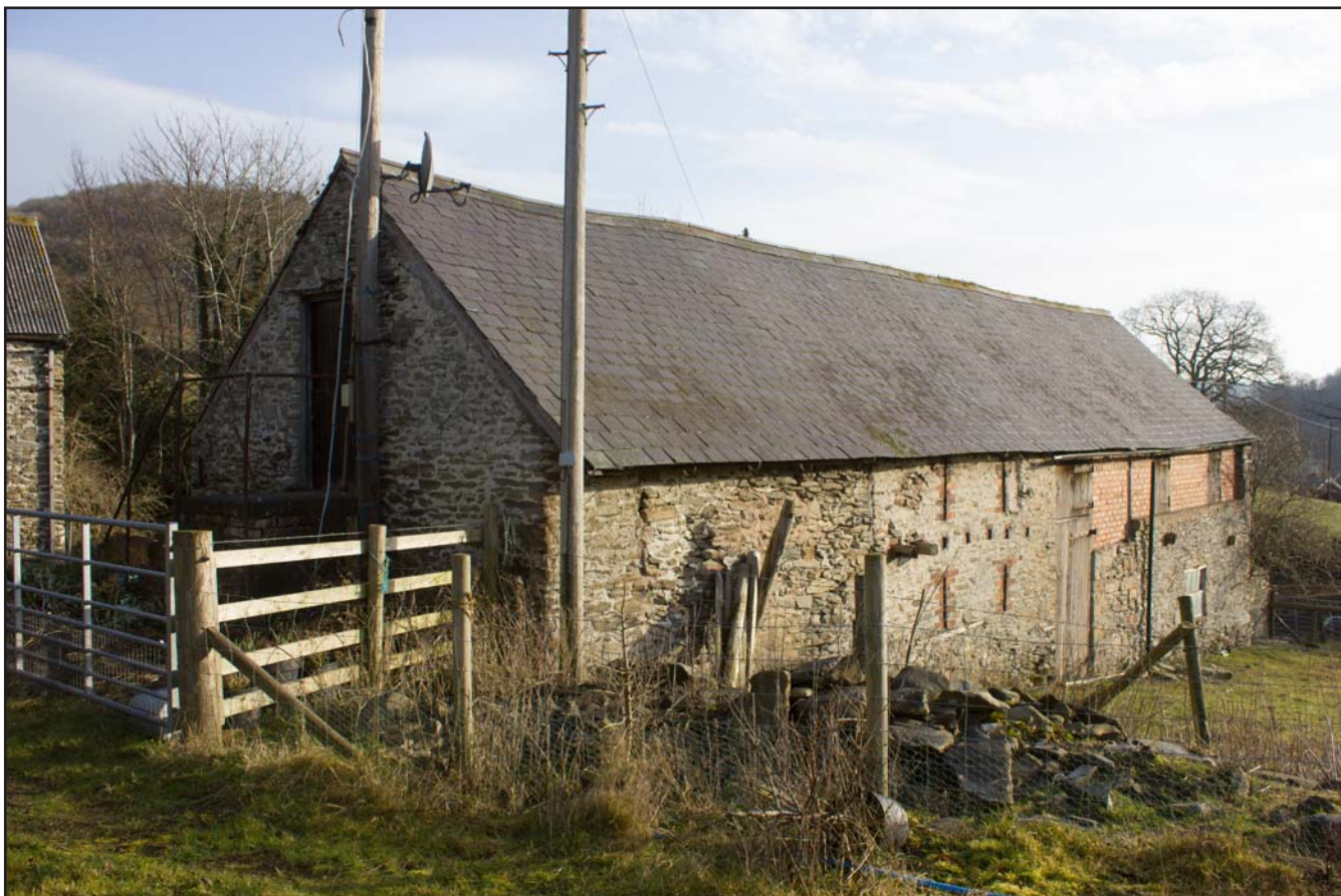
Plate 18: Oblique shot of western and southern elevations of Outbuilding at Tŷ Mawr, Pontfadog, Llangollen, Wrexham - from the southwest - no scale
