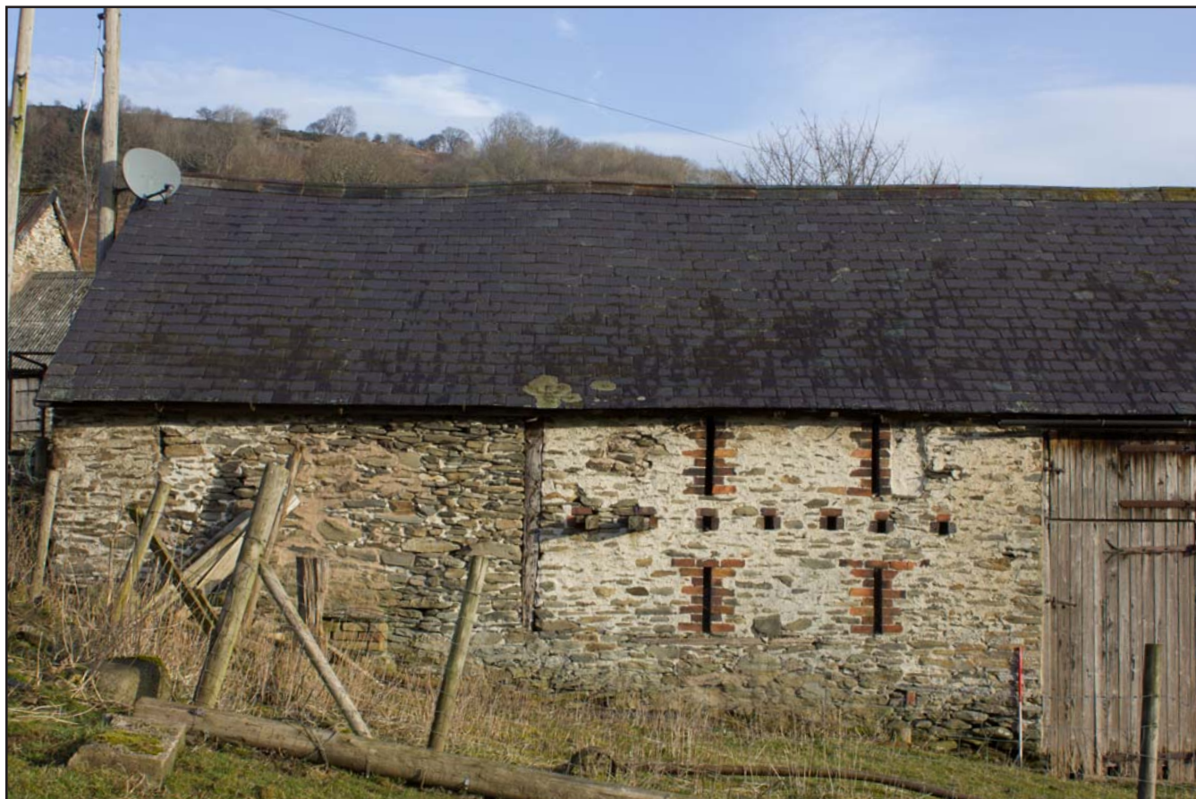
Plate 14: Southern elevation (left) of Outbuilding at Tŷ Mawr, Pontfadog, Llangollen, Wrexham - from the south - 1.00m scale
