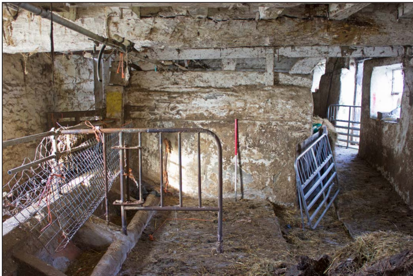
Plate 26: Milking Parlour (east room) within Outbuilding at Tŷ Mawr, Pontfadog, Llangollen, Wrexham - from the east - 1.00m scale
