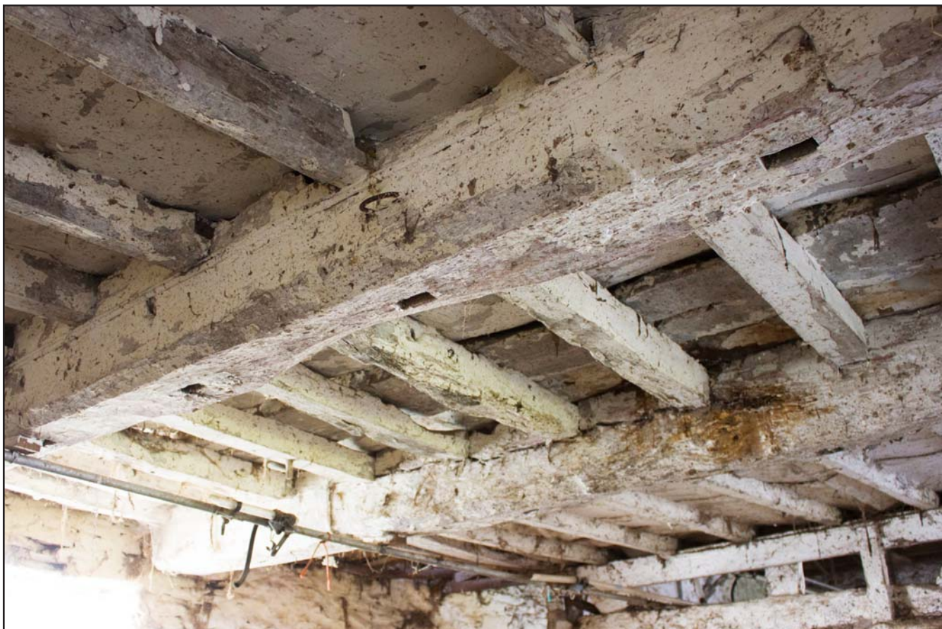
Plate 30: Ceiling & floor joists within eastern milking parlour room within Outbuilding at Tŷ Mawr, Pontfadog, Llangollen, Wrexham - from the southwest - no scale
