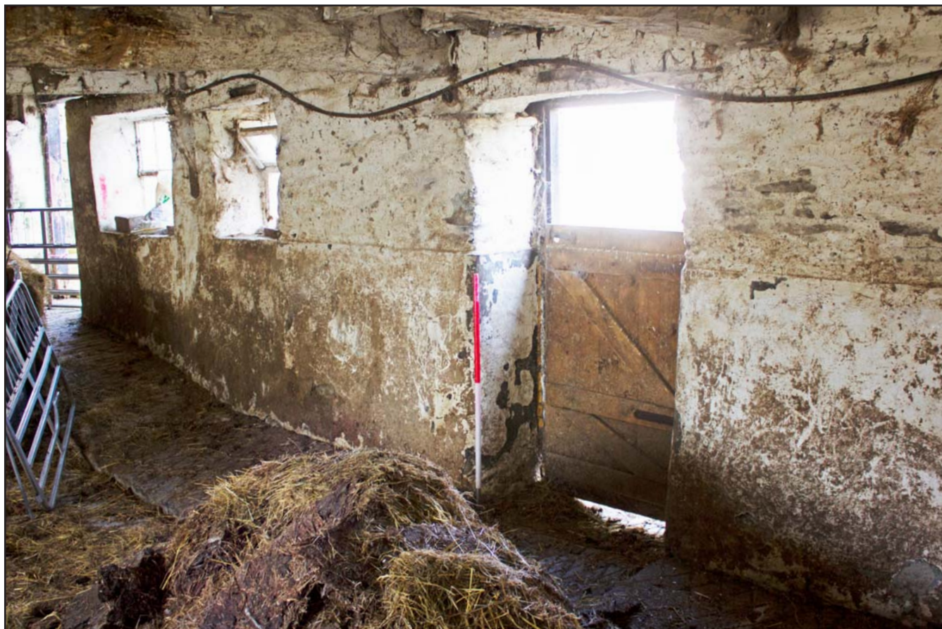
Plate 29: Oblique northern elevation, eastern milking parlour room within Outbuilding at Tŷ Mawr, Pontfadog, Llangollen, Wrexham - from the southeast - 1.00m scale
