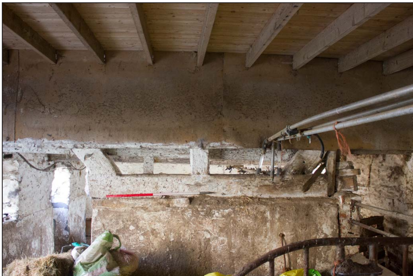
Plate 25: Roof truss ground floor wall support, within Outbuilding at Tŷ Mawr, Pontfadog, Llangollen, Wrexham - from the west - 1.00m scale
