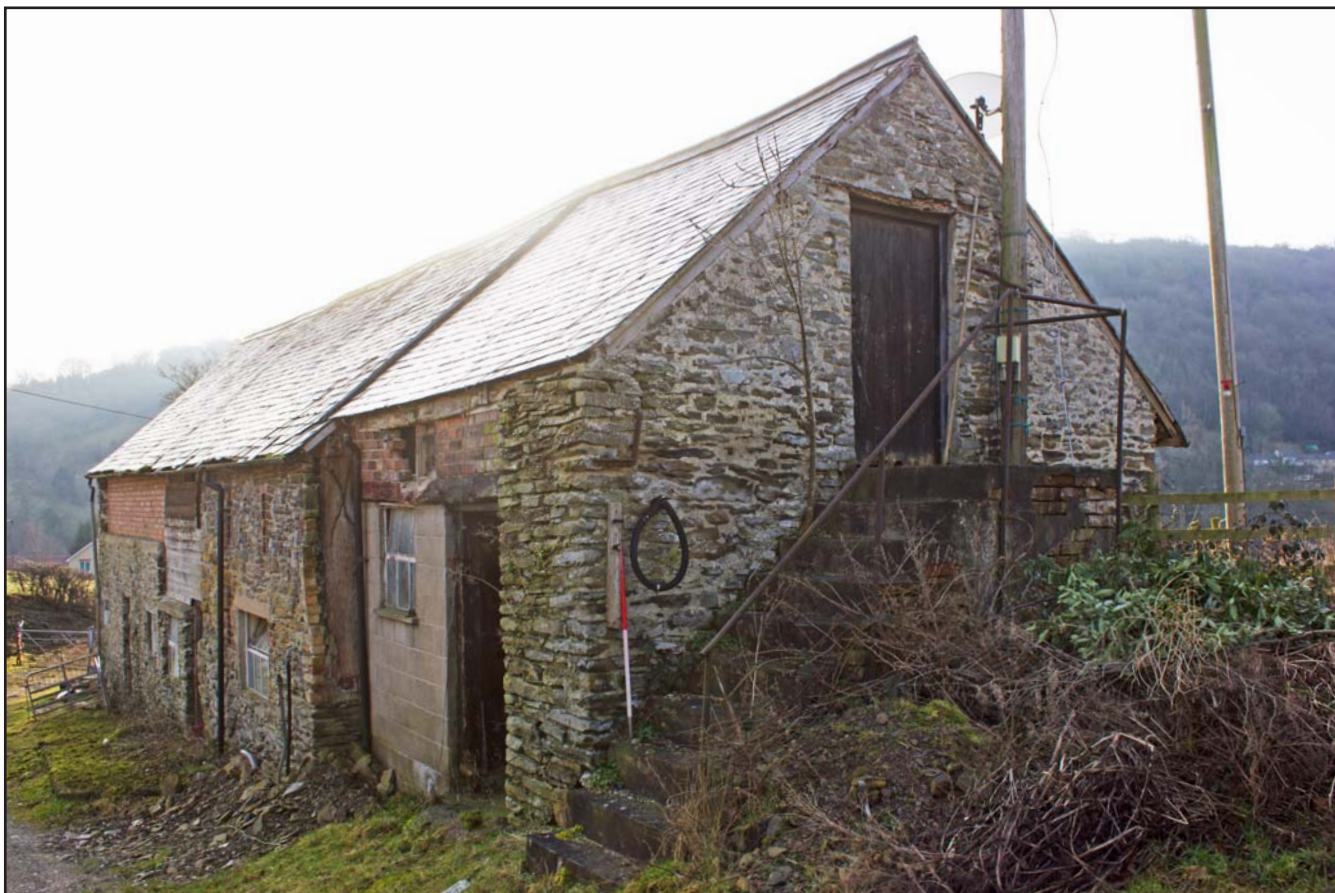
Plate 05: Oblique shot of western and northern elevations of Outbuilding at Tŷ Mawr, Pontfadog, Llangollen, Wrexham - from the northwest - 1.00m scale
