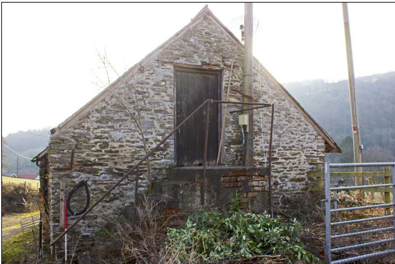
Plate 04: Western gable elevation of Outbuilding at Tŷ Mawr, Pontfadog, Llangollen, Wrexham - from the west - 1.00m scale
