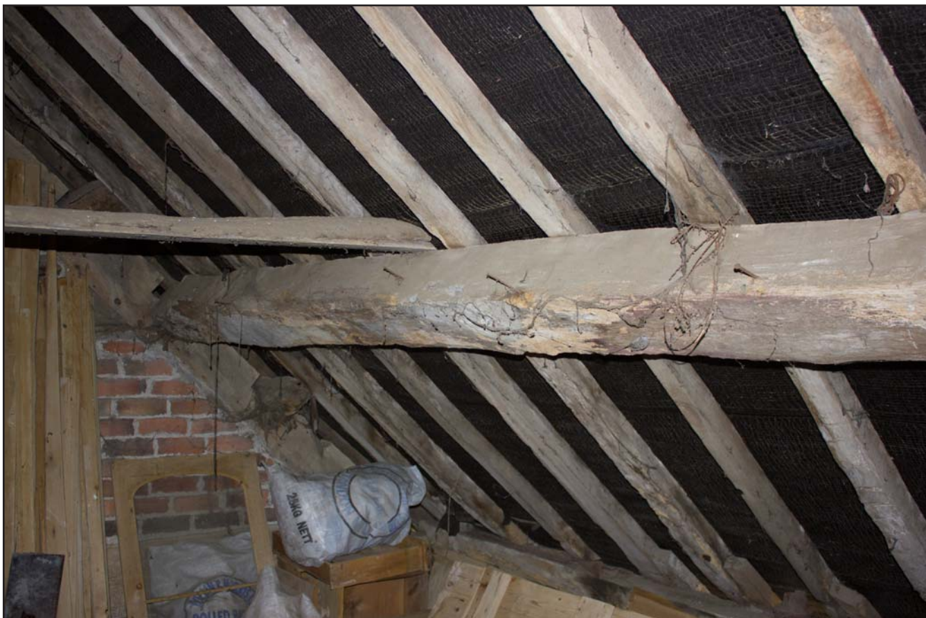
Plate 33: Roof purlin, 1st Floor storage room within Outbuilding at Tŷ Mawr, Pontfadog, Llangollen, Wrexham - from the northwest - no scale
