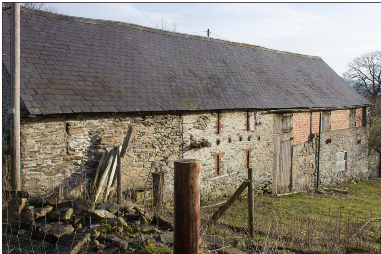
Plate 19: Oblique shot of southern elevation of Outbuilding at Tŷ Mawr, Pontfadog, Llangollen, Wrexham - from the southwest - no scale
