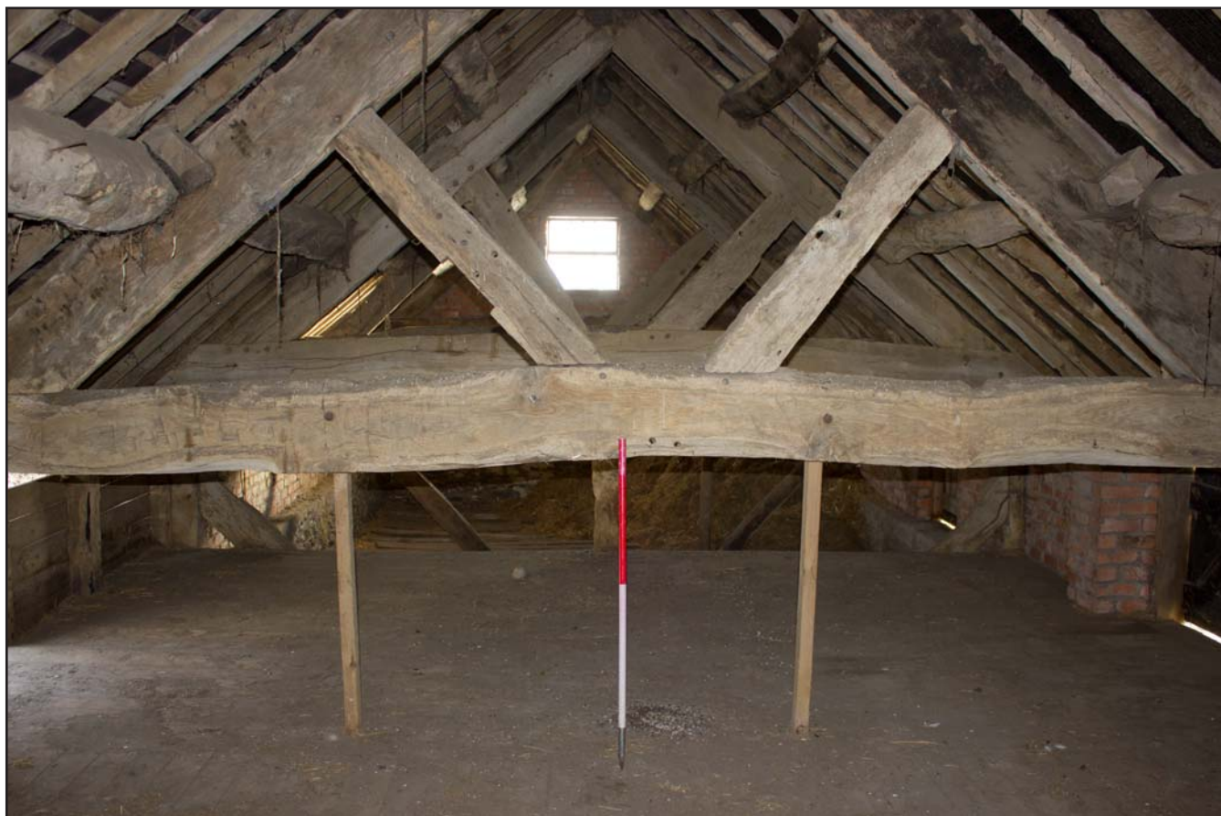
Plate 35: Collar tie beam trusses with raking struts within the Hayloft inside the Outbuilding at Tŷ Mawr, Pontfadog, Llangollen, Wrexham - from the west - 1.00m scale
