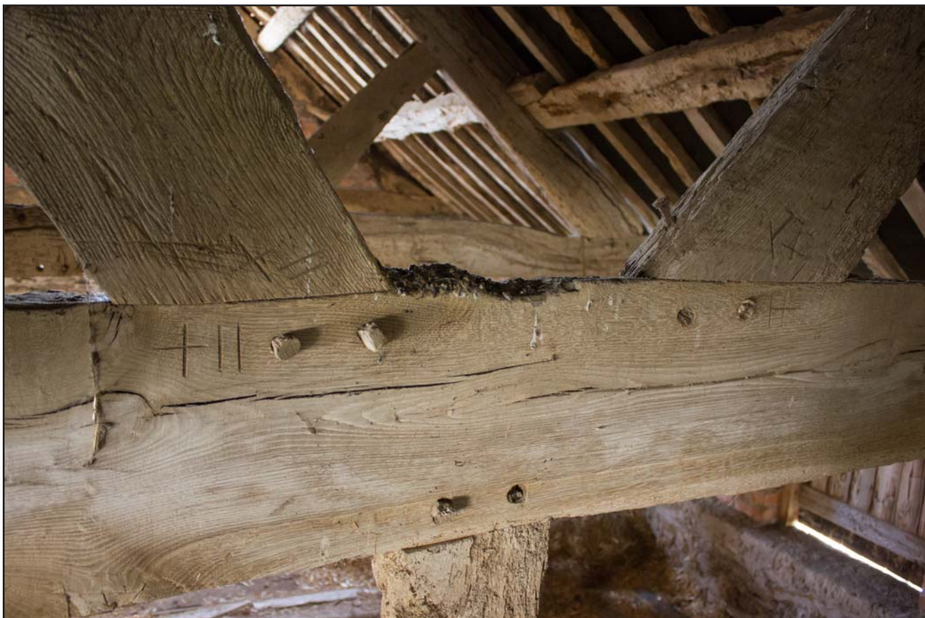
Plate 45: Carpenter's marks and dowel joint reinforcement on trusses in Hayloft Outbuilding at Tŷ Mawr, Pontfadog, Llangollen, Wrexham - from the northwest - no scale
