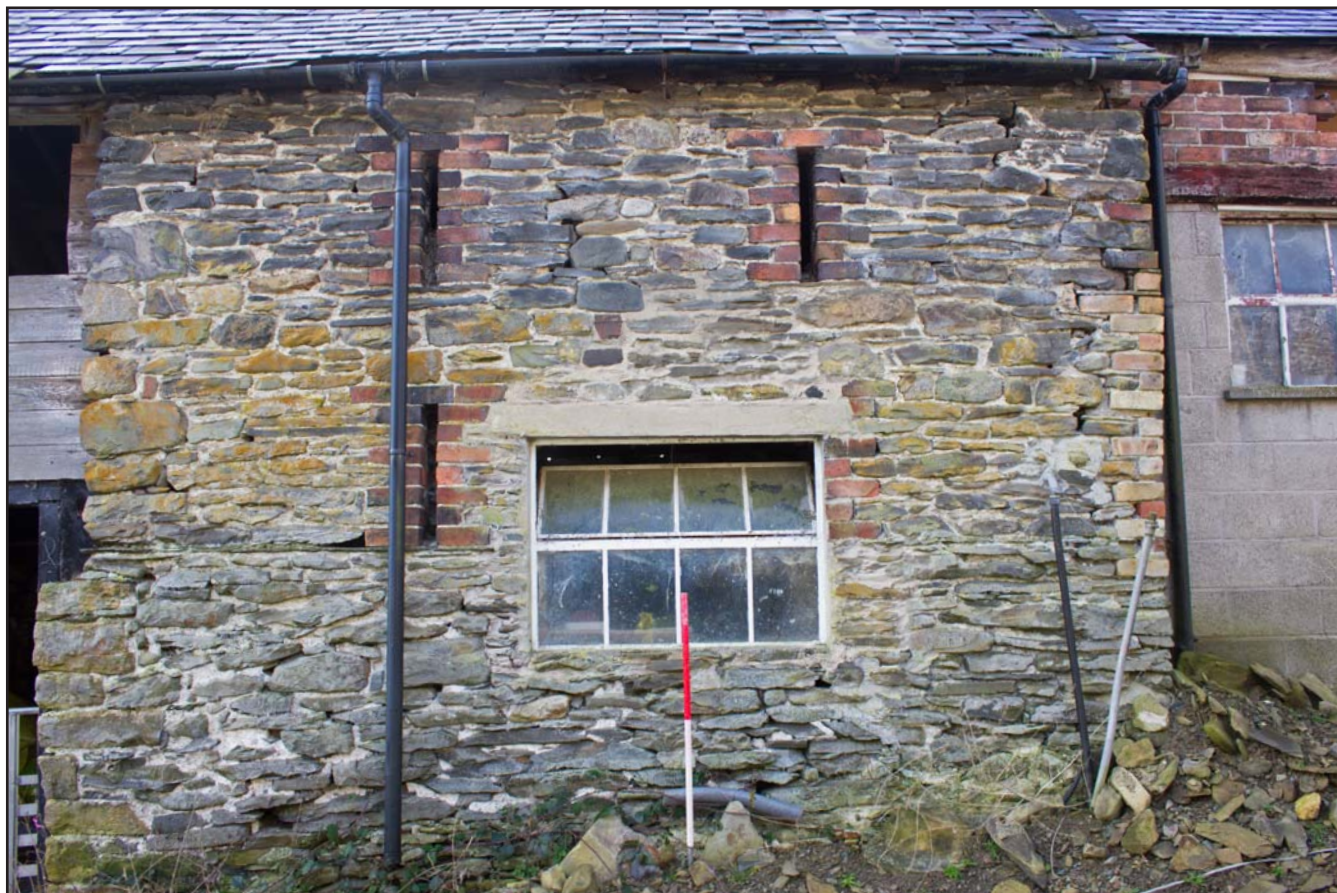
Plate 17: Ventilation embrasure slots in northern elevation of Outbuilding at Tŷ Mawr, Pontfadog, Llangollen, Wrexham - from the north - 1.00m scale
