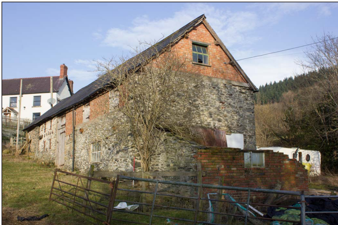
Plate 11: Oblique shot of eastern and southern elevations of Outbuilding at Tŷ Mawr, Pontfadog, Llangollen, Wrexham - from the southeast - 1.00m scale
