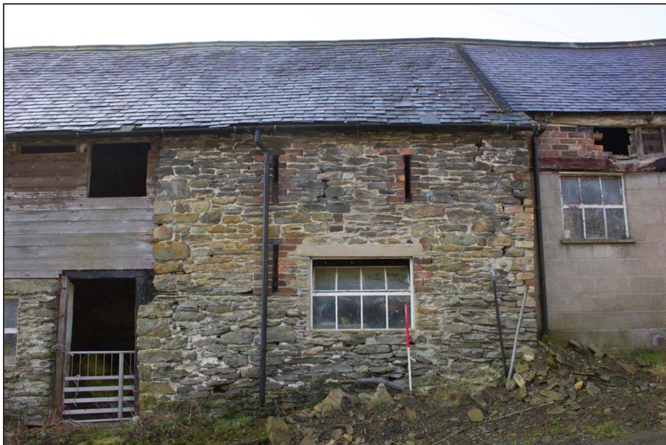
Plate 07: Northern elevation (centre) of Outbuilding at Tŷ Mawr, Pontfadog, Llangollen, Wrexham - from the north - 1.00m scale
