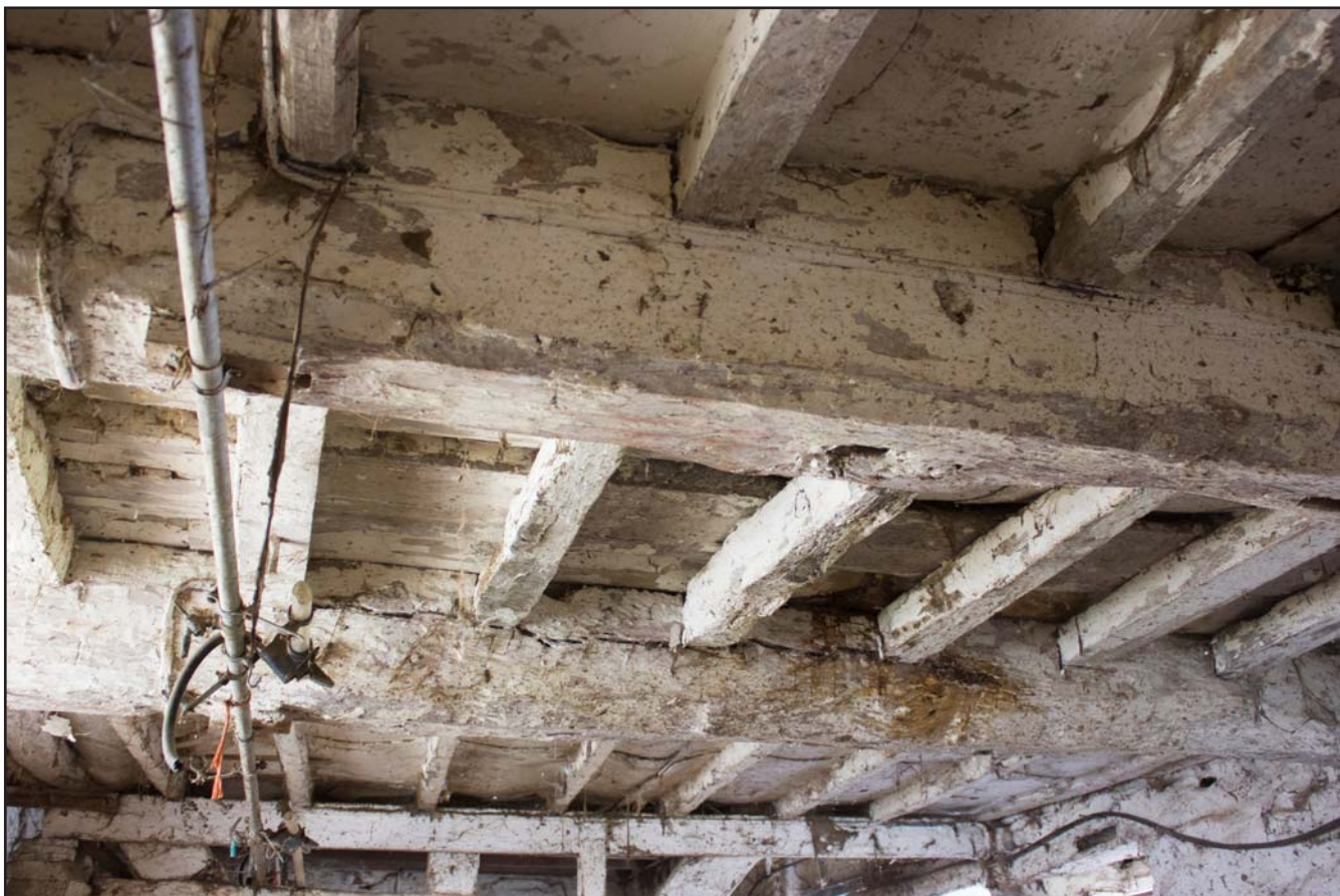
Plate 31: Ceiling & floor joists within eastern milking parlour room within Outbuilding at Tŷ Mawr, Pontfadog, Llangollen, Wrexham - from the southeast - no scale
