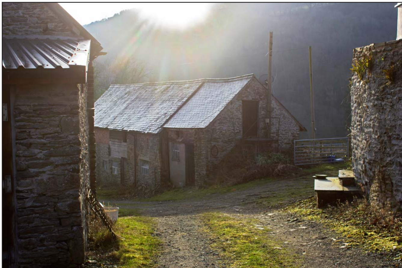
Plate 01: Context Shot of the Outbuilding at Tŷ Mawr, Pontfadog, Llangollen, Wrexham - from the southwest - 1.00m scale
