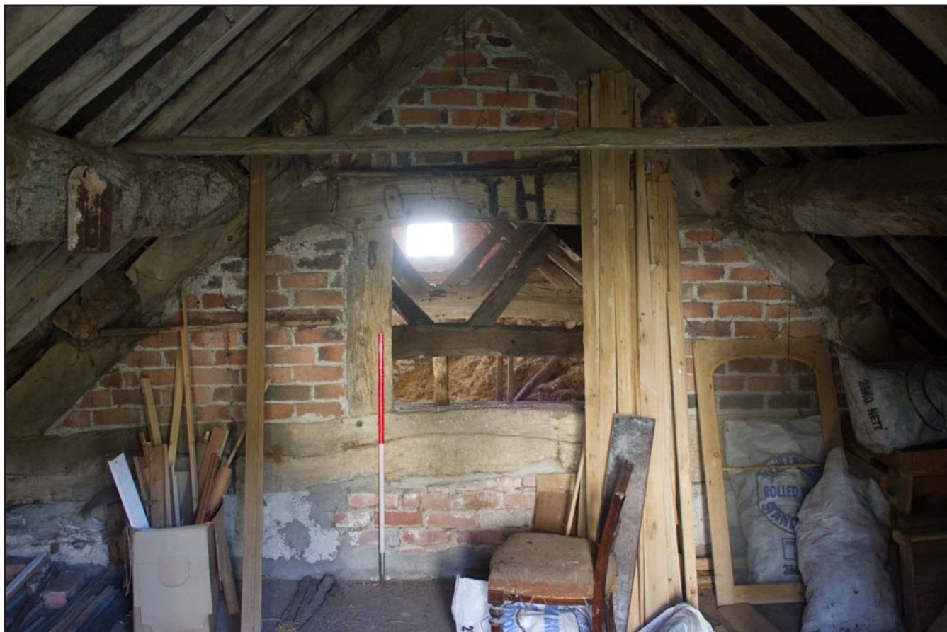
Plate 32: 1st Floor storage room within Outbuilding at Tŷ Mawr, Pontfadog, Llangollen, Wrexham - from the west - 1.00m scale
