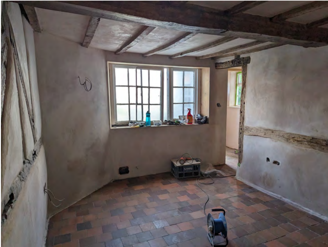
Office - All walls and ceiling lime plastered
