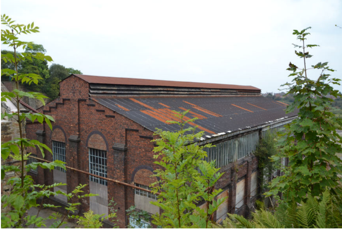
View of the roof from path above
