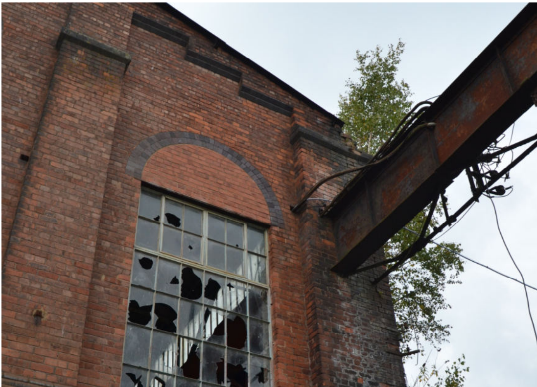
Industrial features will be retained
