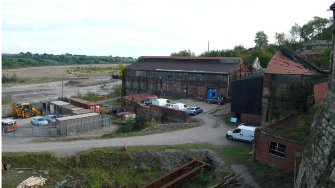
North elevation and existing car park
