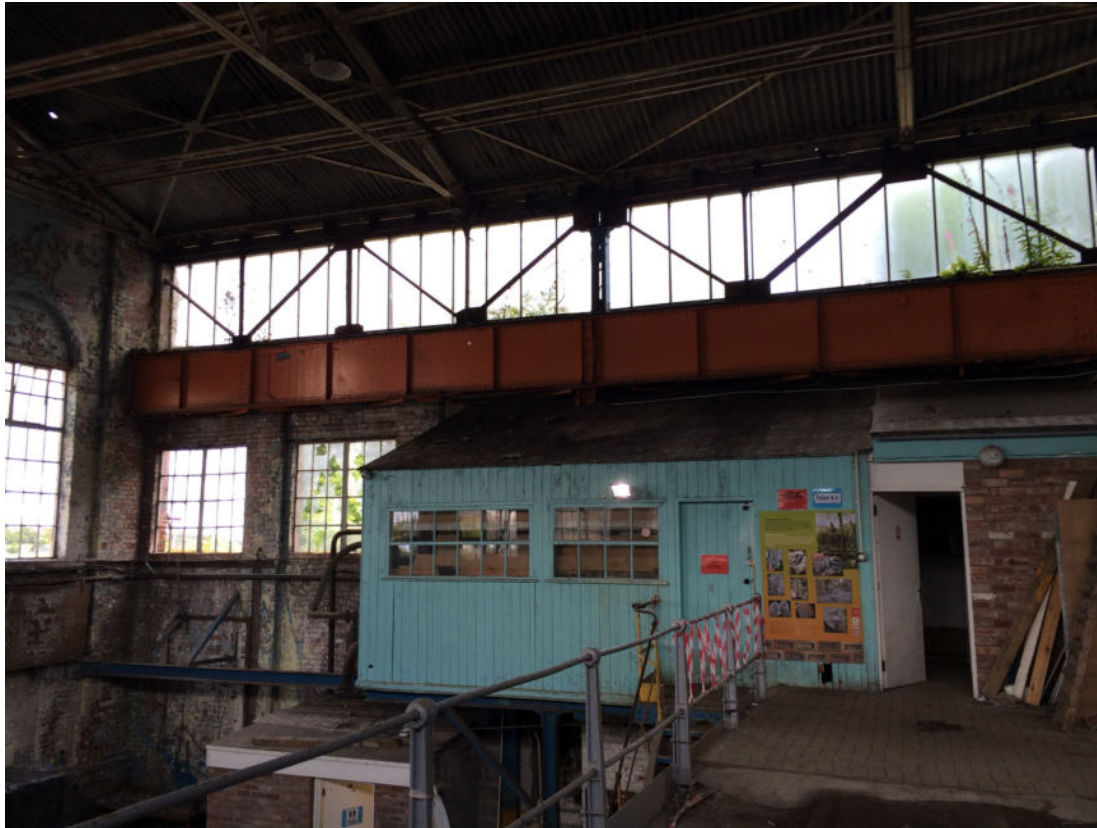
The structure is apparent internally and creates much of the character
