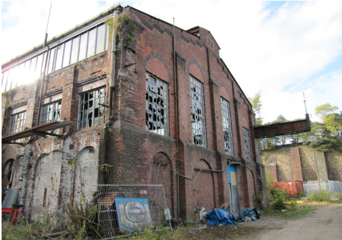
The gable end elevation faces the main road. The existing door opening will become the main visitors entrance.
