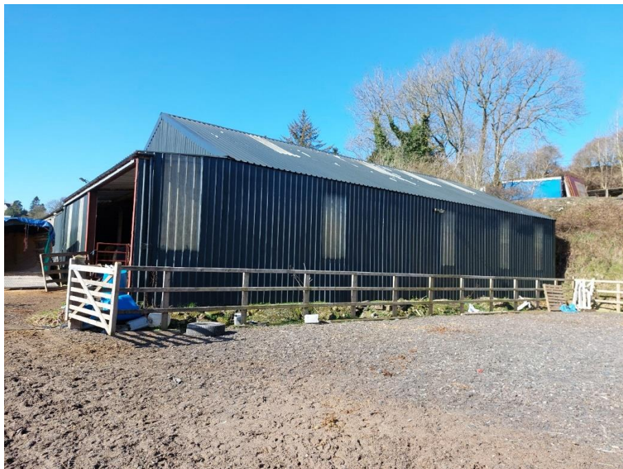
Figure 4.3. External view of the eastern extension
