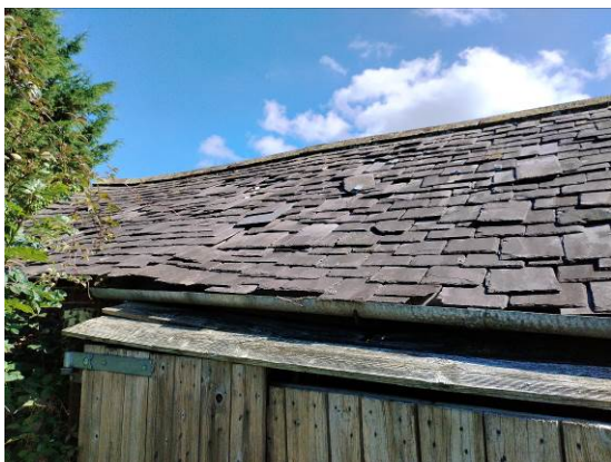
Photo 3 – Typical condition of roof finishes.
