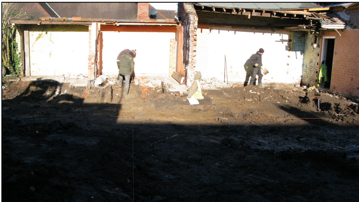
Site prepared for trenching work.
