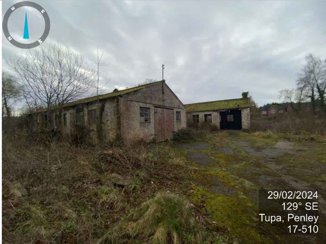
PLATE 1 VIEW OF FORMER HOSPITA BUILDING FACING SOUTH-EAST
