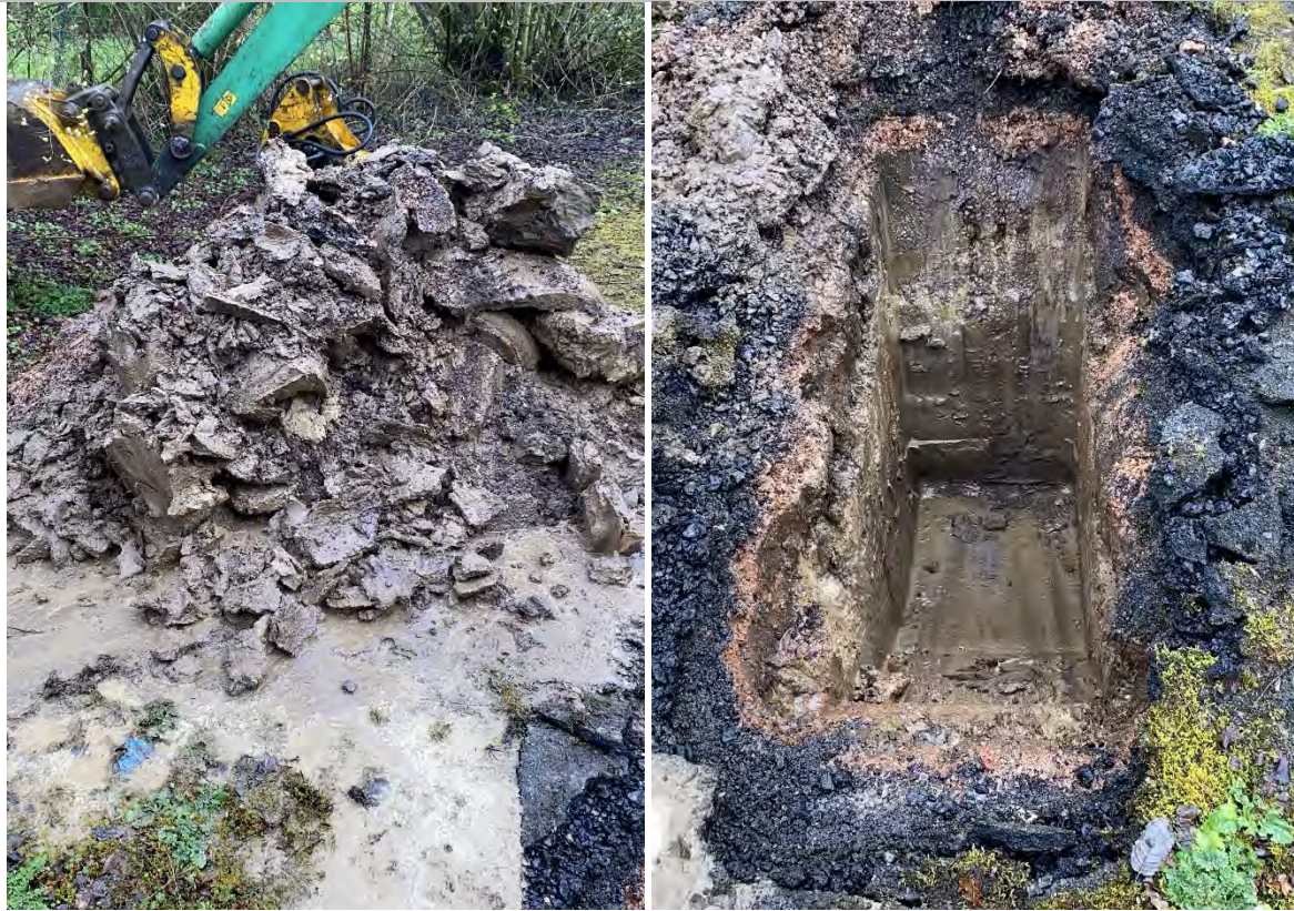
PLATE 5 TRIAL PIT TP101 & ARISINGS
