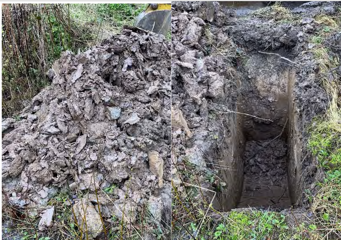
PLATE 6 TRIAL PIT TP104 & ARISINGS
