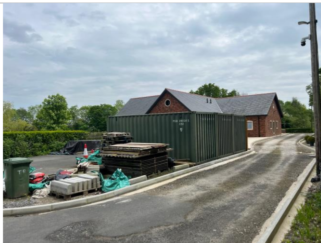
Southern edge of compound fitted with curbs.
