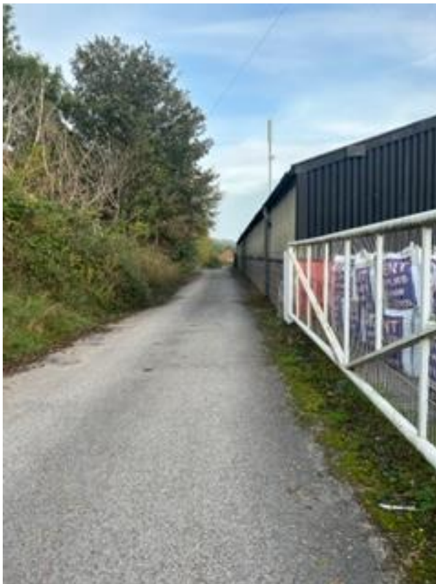
Exterior prior to works
