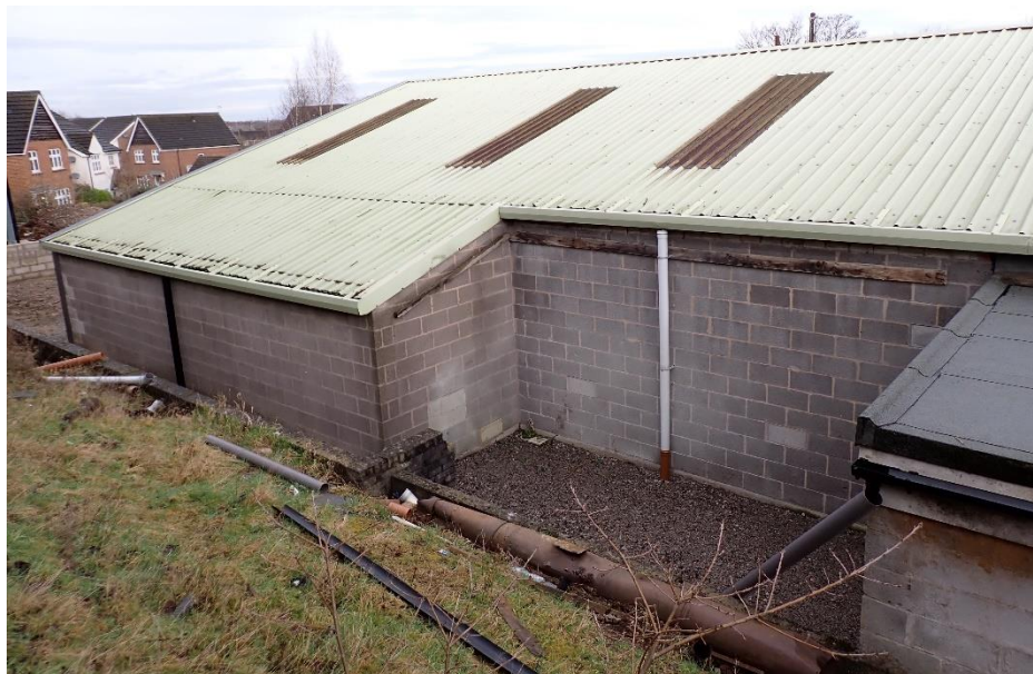
The southwest elevation of the main building towards the northern end ( Target Note 10 ).
