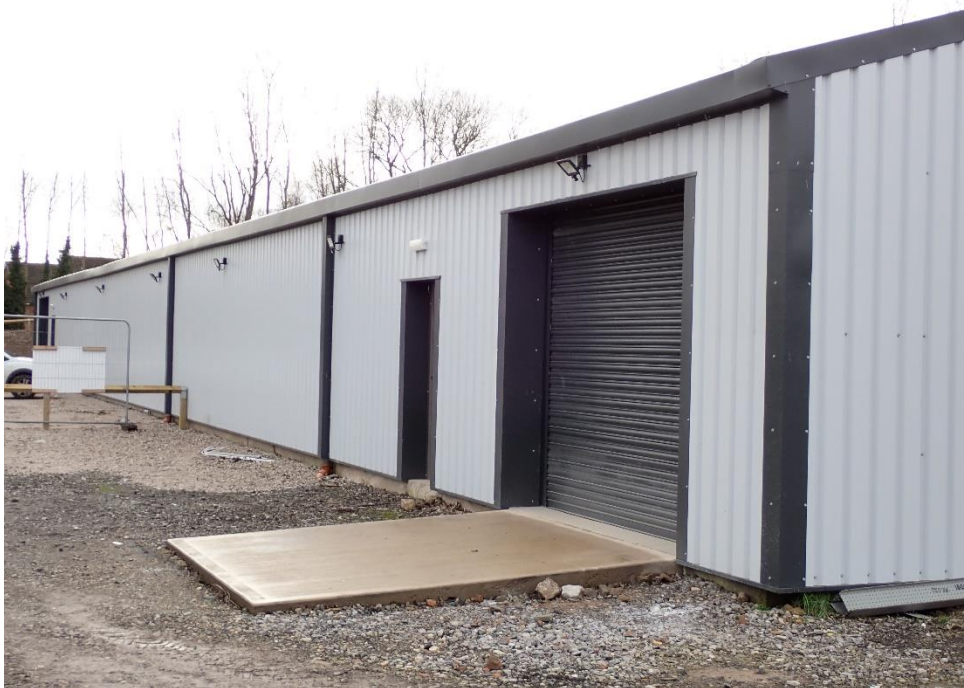
The northeast elevation ( Target Note 10 ).
