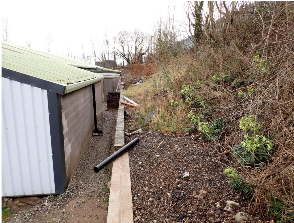
The slope at Target Note 8 viewed from the northwest end.
