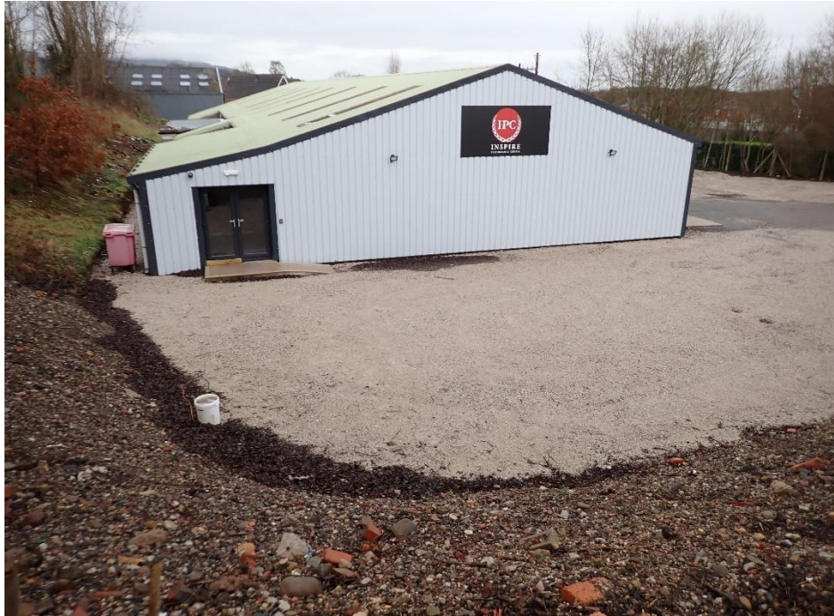
The southeast elevation ( Target Note 10 ).
