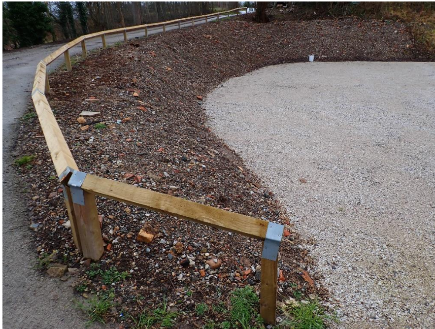
The slope at Target Note 9 .
