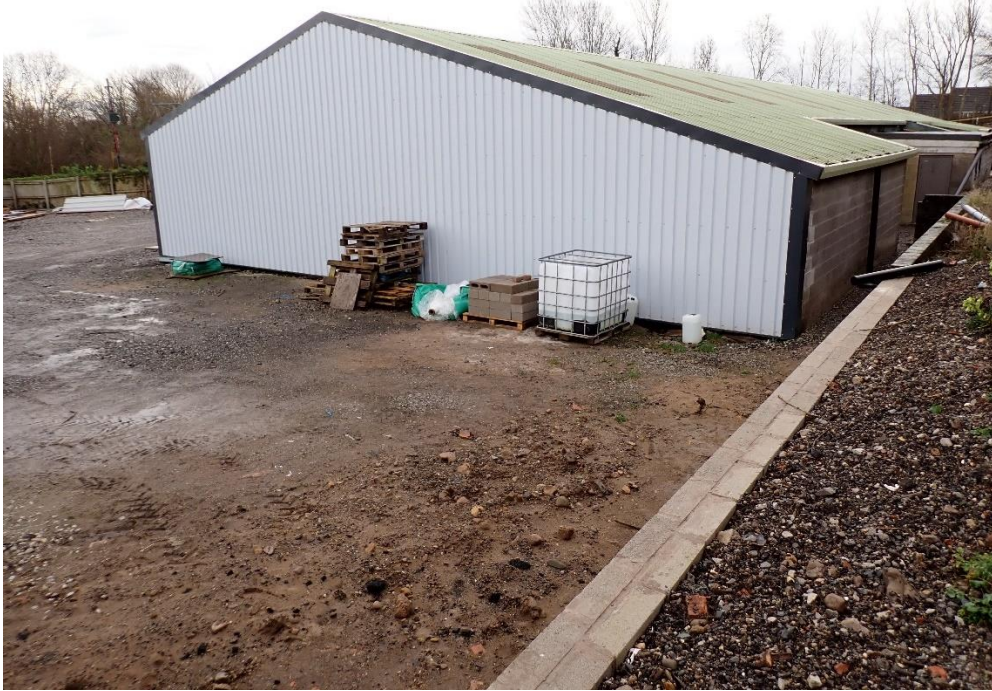
The northwest elevation ( Target Note 10 ).
