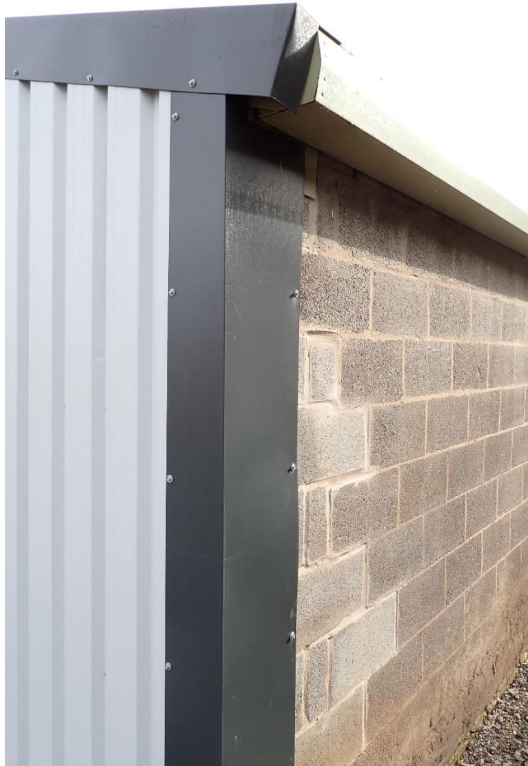
The corner of the building ( Target Note 10 ) between the northwest and southwest elevations.
