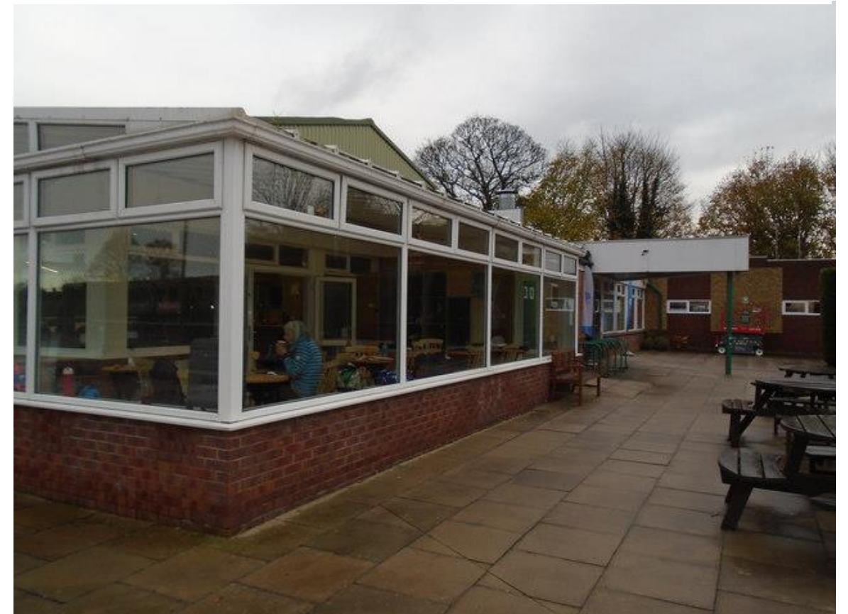
External View of Corner Conservatory Extension
