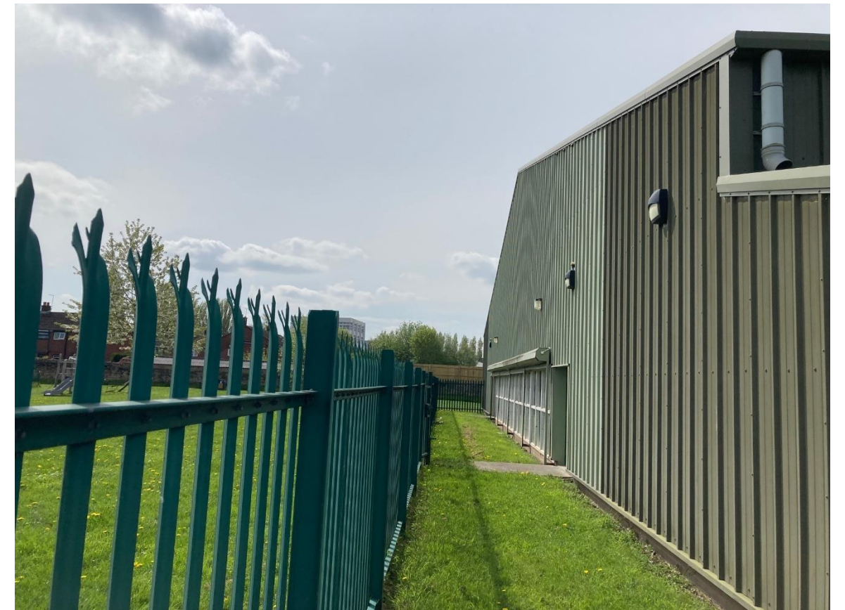
External View of Portal Frame South Gable
