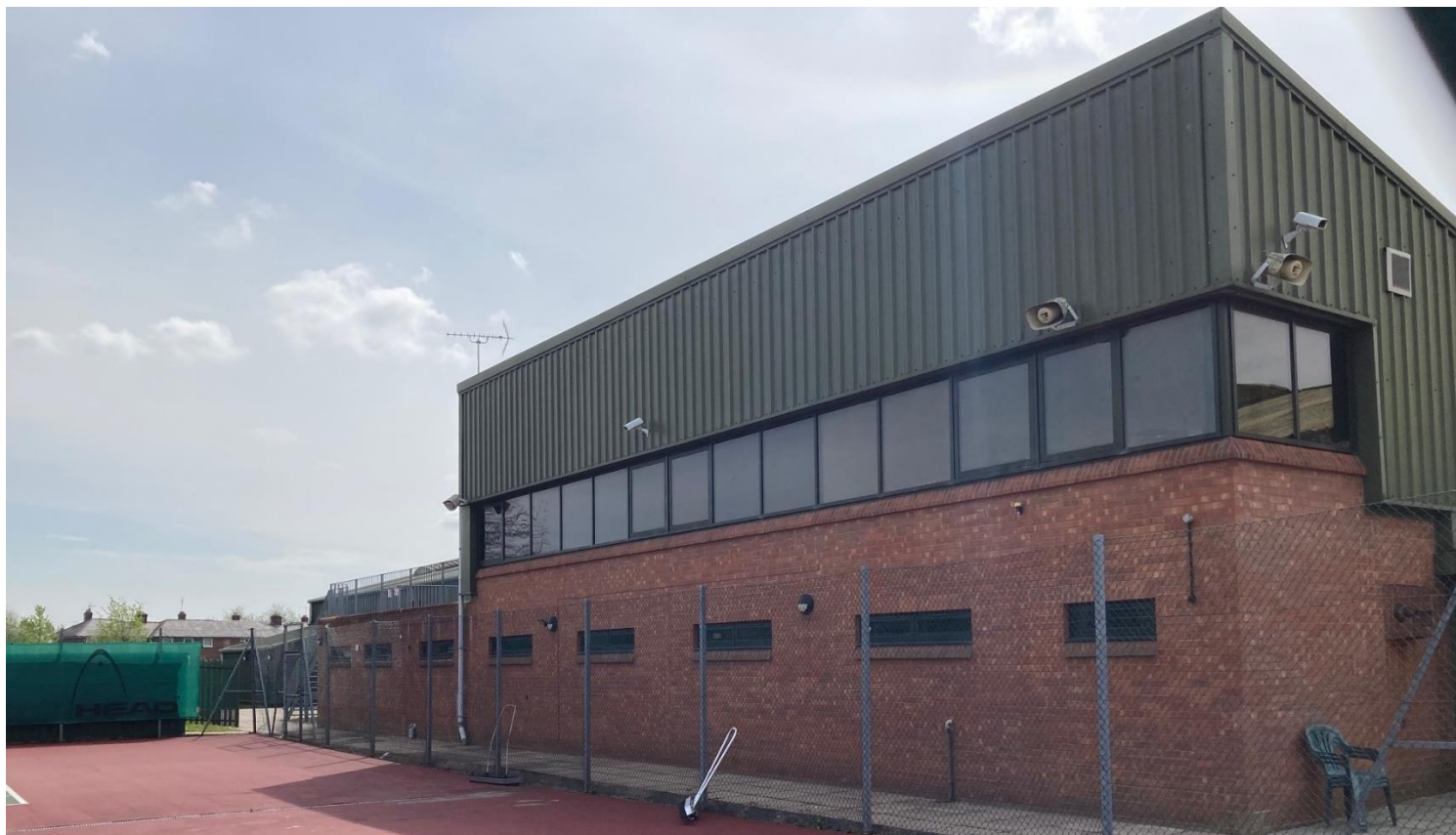
External View of Side Extension
