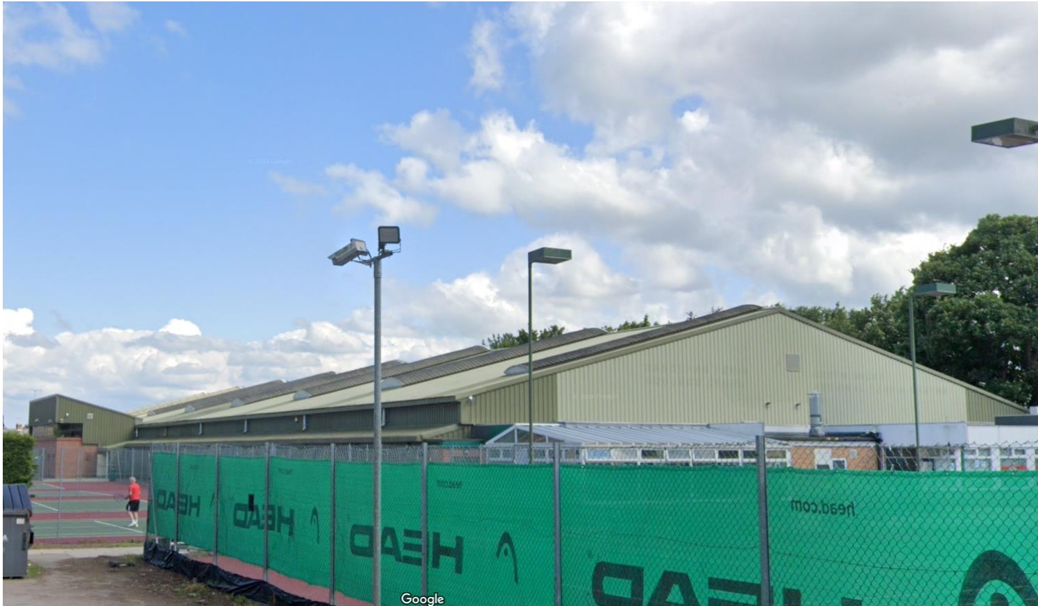
External View of Portal Frame and Side Extension
