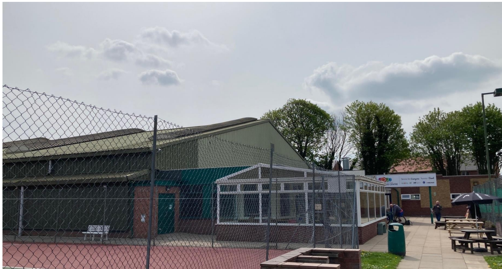
External View of Single Storey Frontage from Outdoor Courts
