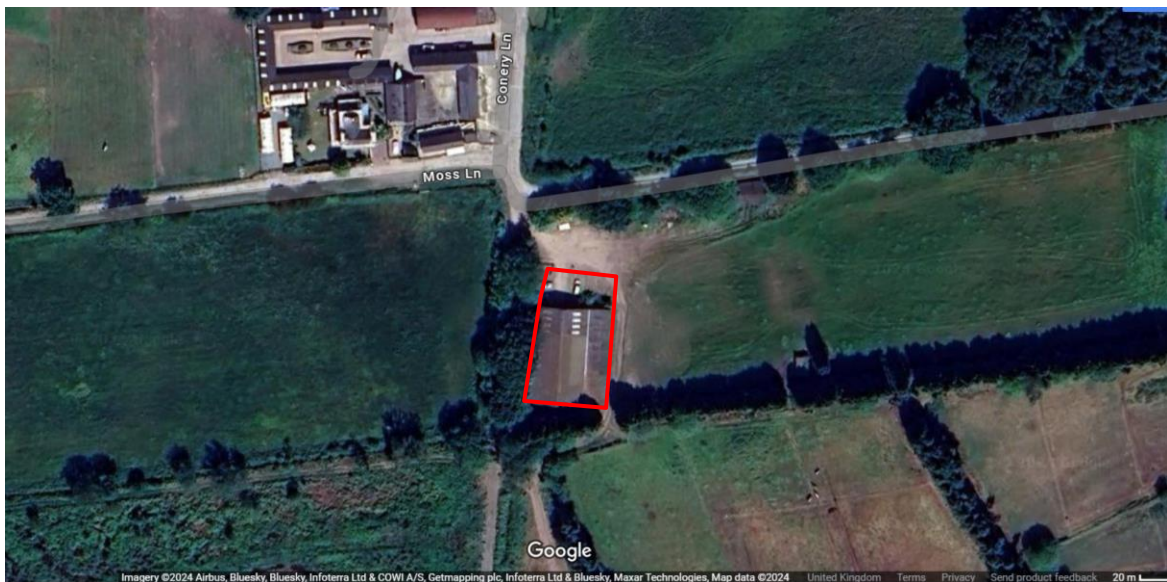
Figure 1. Aerial view of the site (not to scale). Google Maps, 2024.
