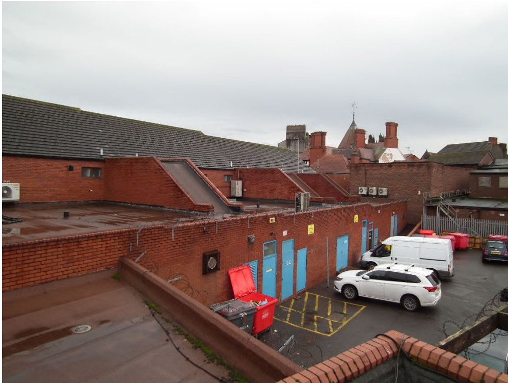
Photo 1 – Flat Roofs and Rear Courtyard
