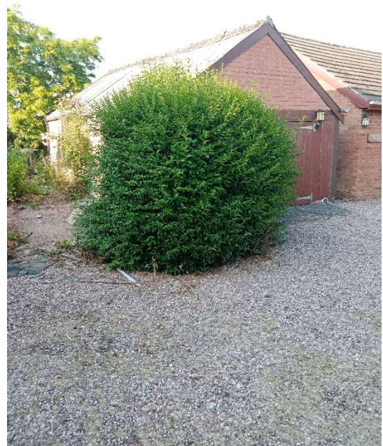
Photo 16: G5 adjacent to the existing garage and workshop building.
