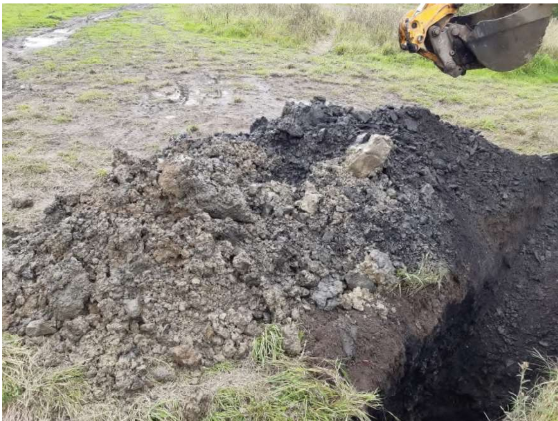
Trial Pit 5 -Spoil
