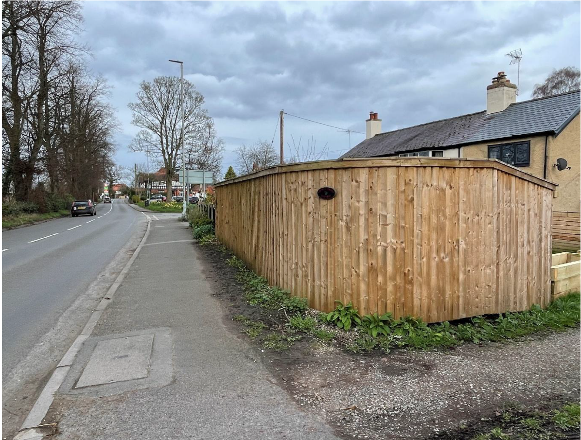
View to the right hand side fencing when leaving the site.
