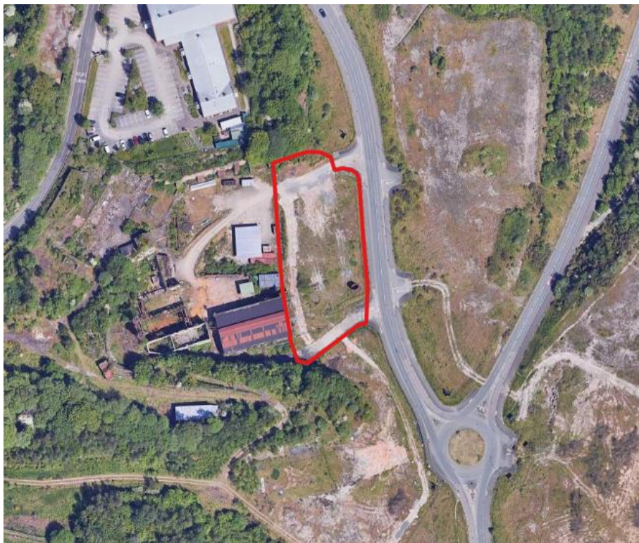
FIGURE 2.1. 'CAR PARK' AT BRYMBO HERITAGE AREA, WITH THE APPROXIMATE SURVEY AREA SHOWN BY THE RED OUTLINE
