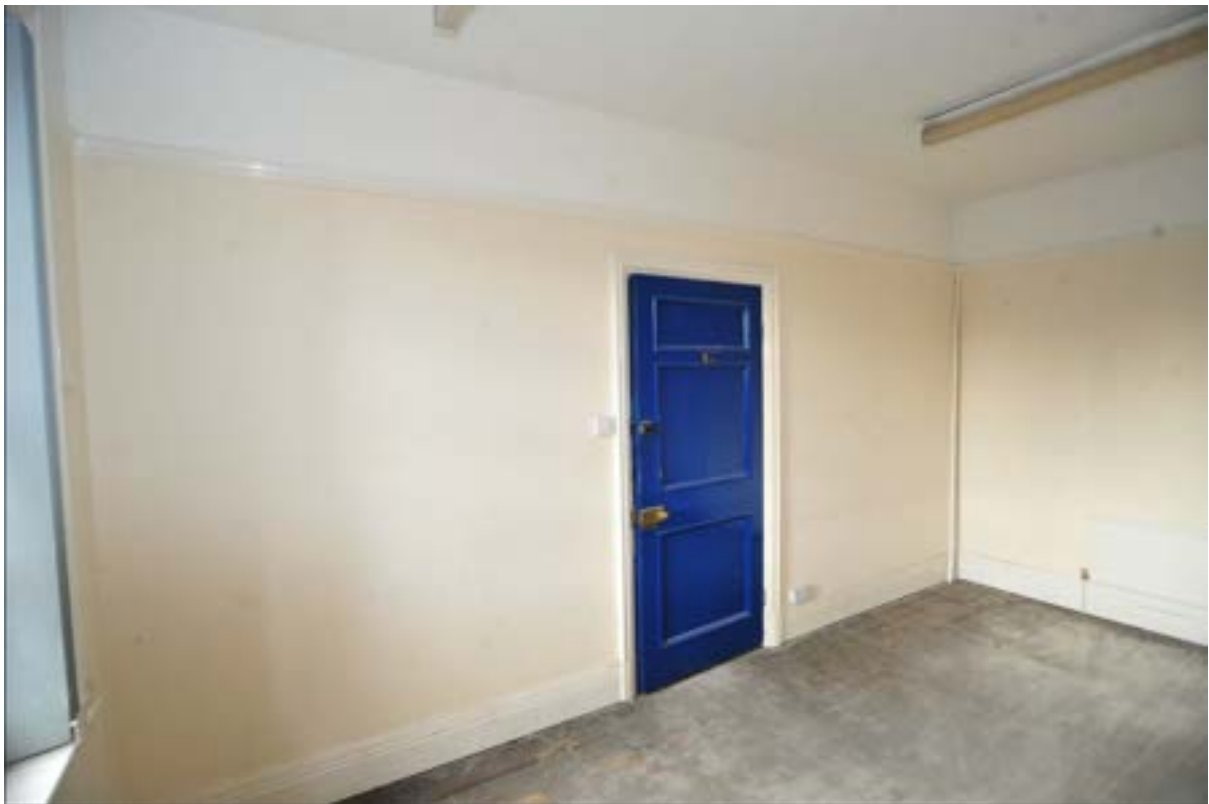
Pl.37: East rear second-floor room looking north-west (1348).
