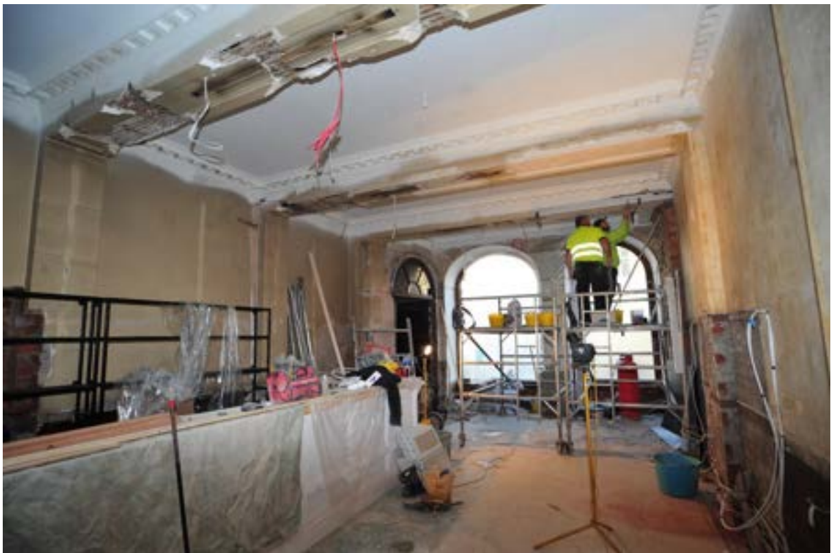
Pl.14: Ground-floor of frontage range, looking north (1375).
