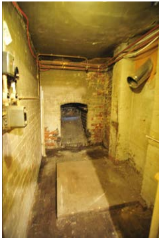
Pl.51: Plant room in basement looking north (1405).
