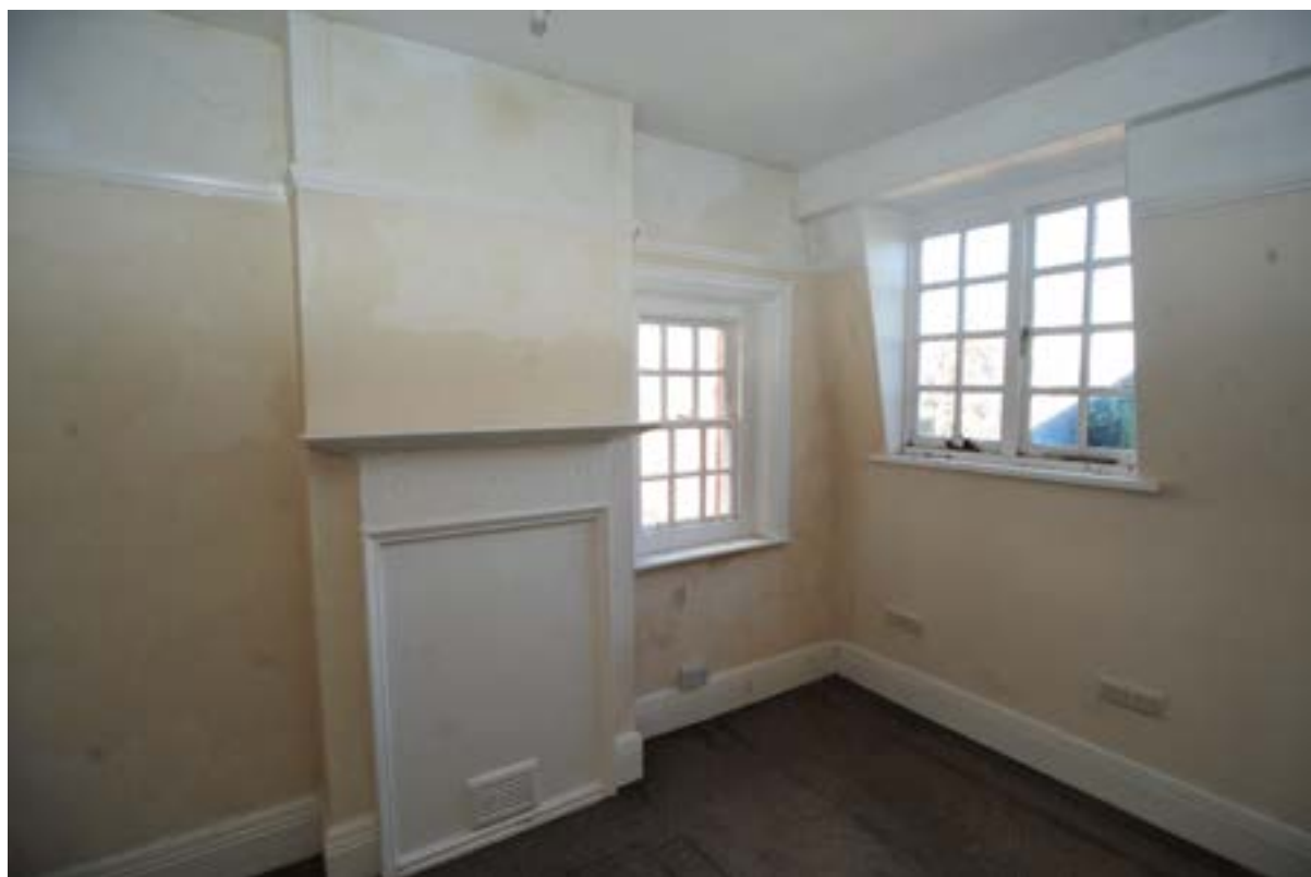
Pl.41: West front third-floor room looking north-west (1332).
