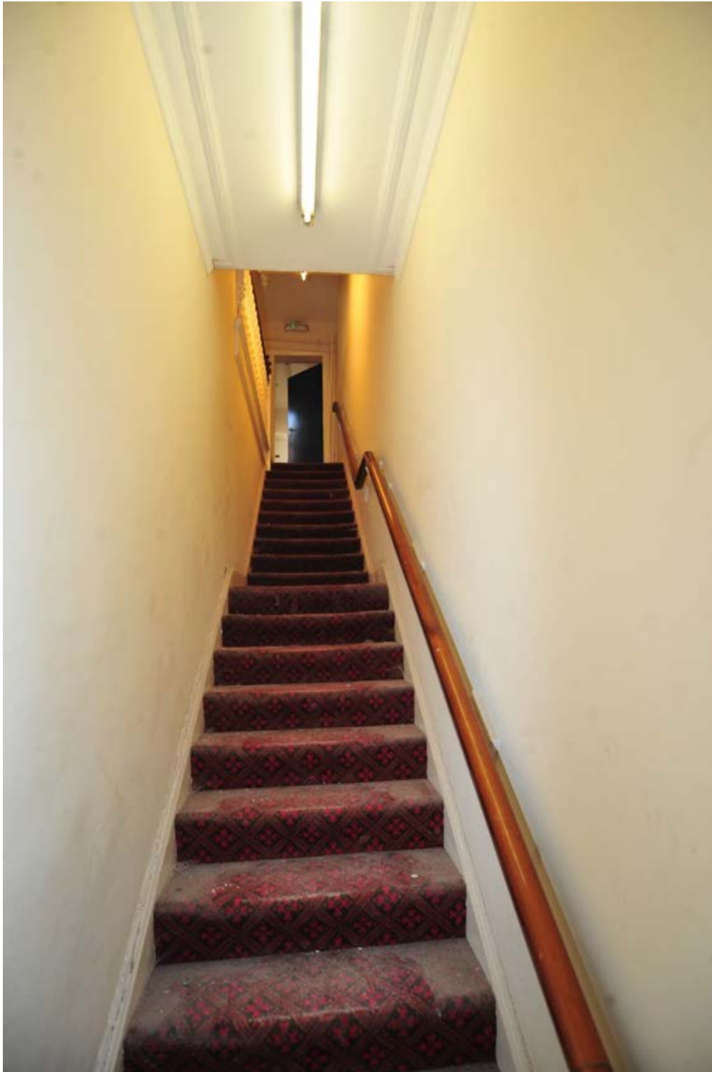
P1.21: Main stairs from lobby (1368).
