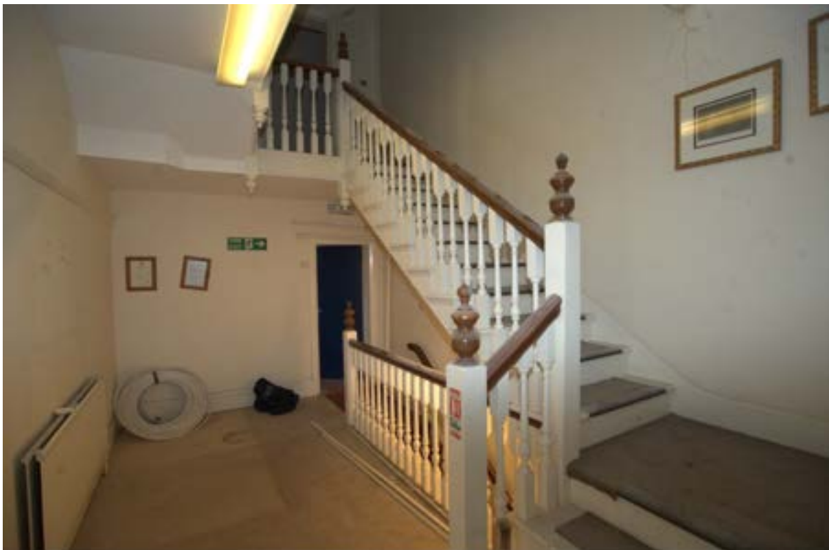
Pl.23: First-floor landing, looking south (1355).
