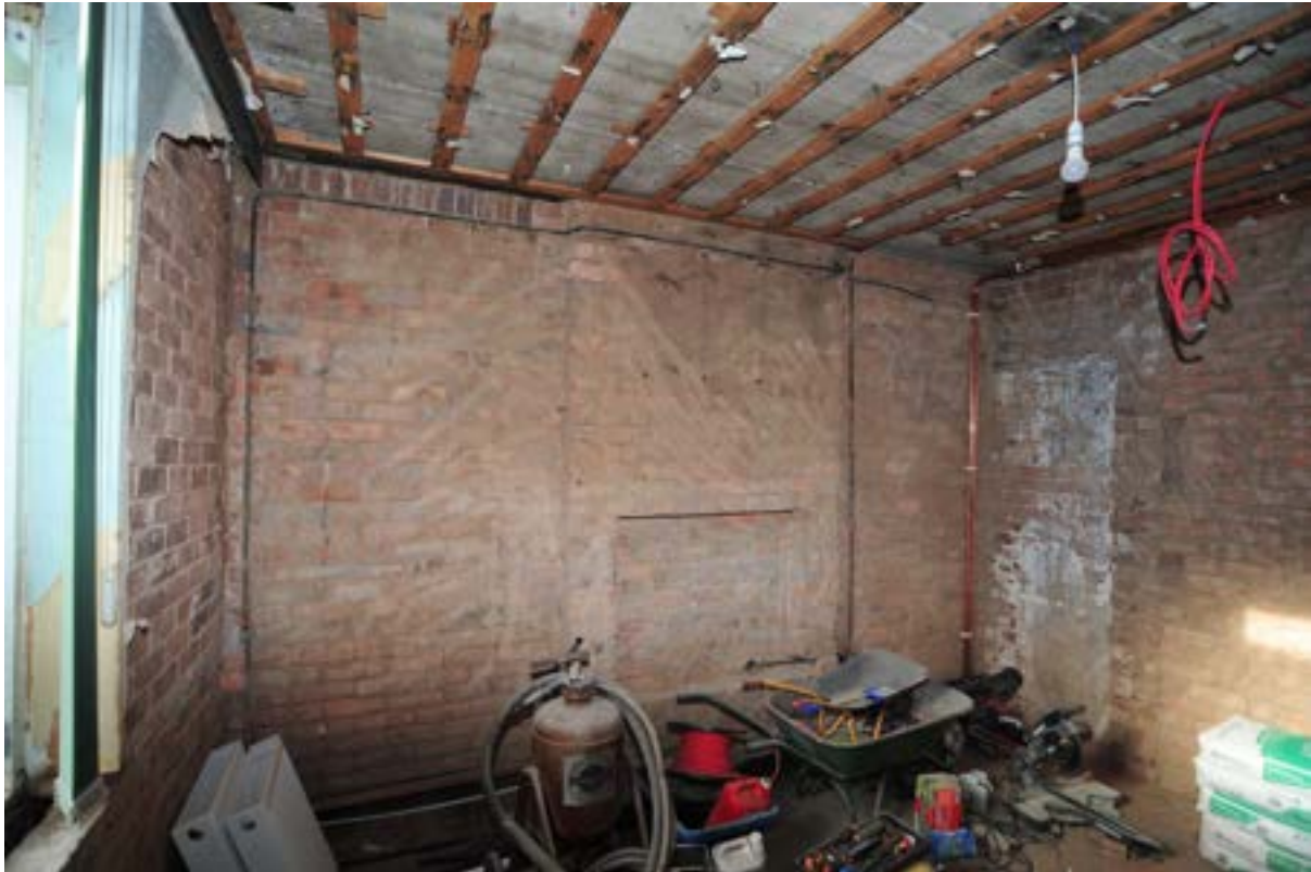
Pl.54: Ground-floor room in original rear wing, looking east (1378).
