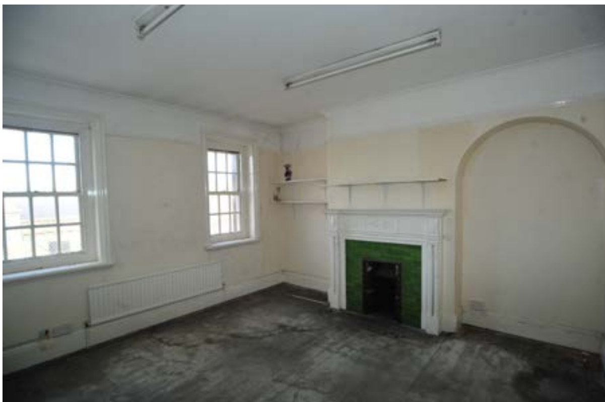
Pl.34: East front second-floor room looking north-east (1344).
