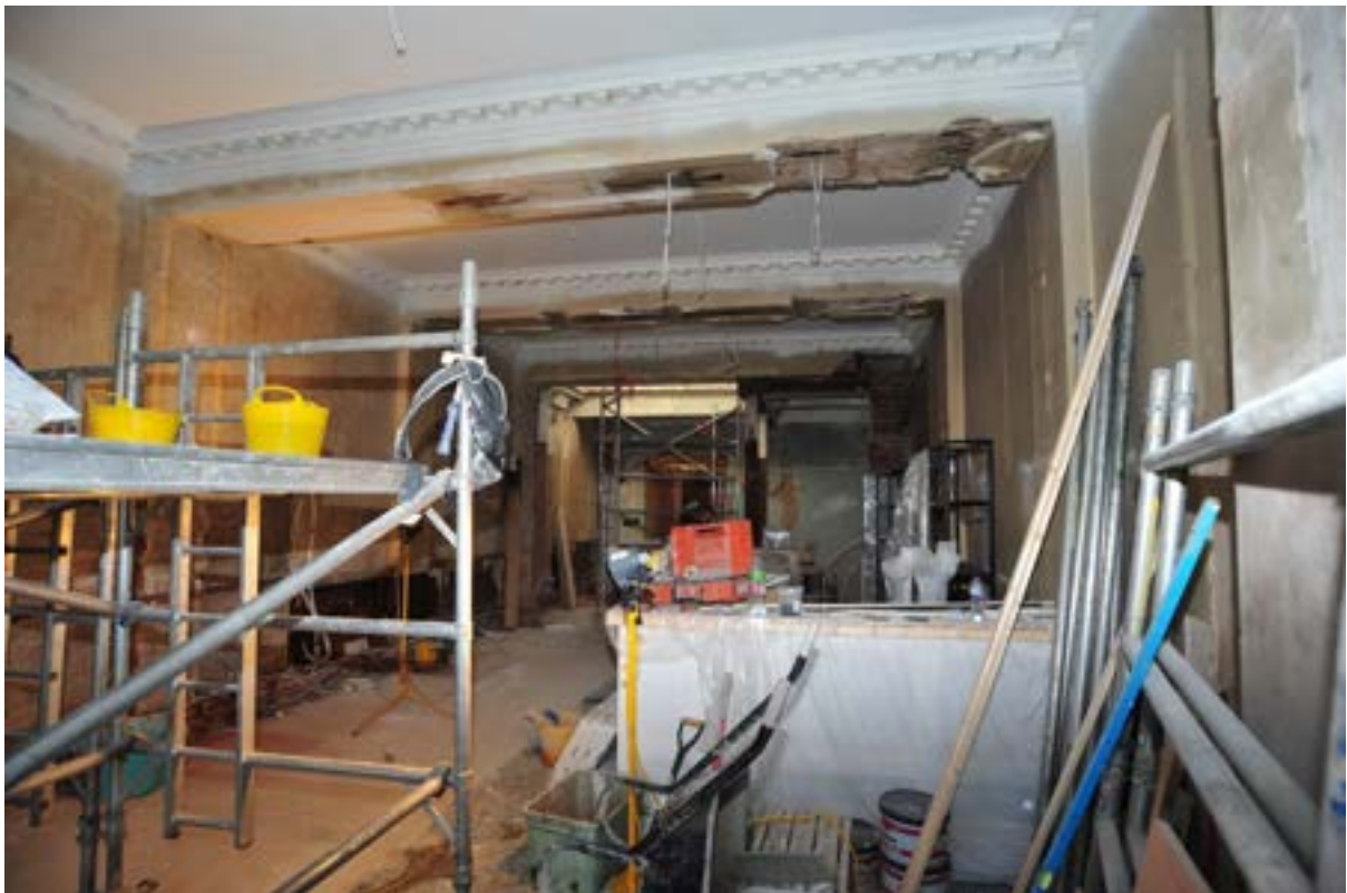
Pl.16: Ground floor looking south (1374).
