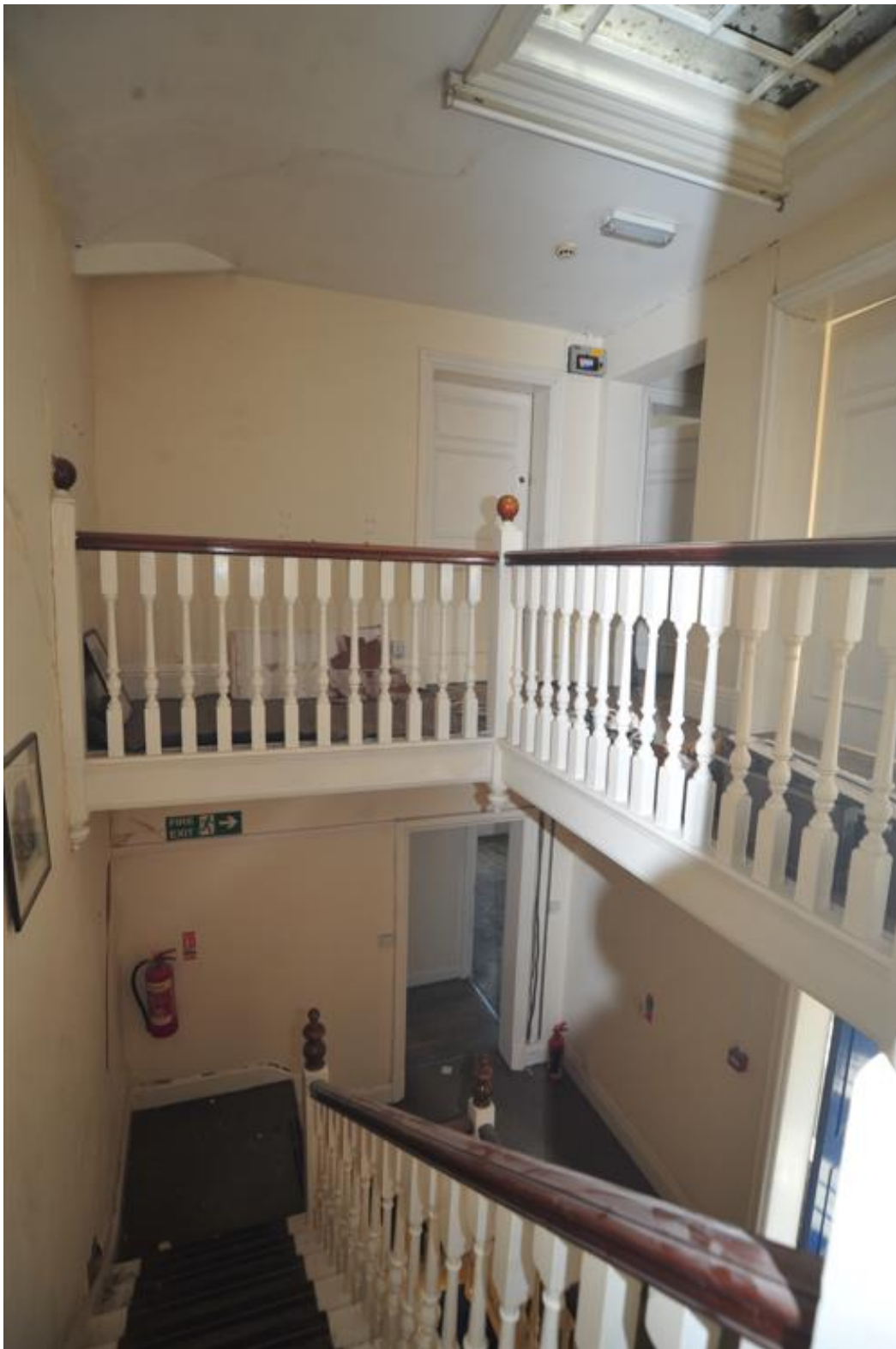
Pl.40: The top of the stairs and the third-floor landing (1339).
