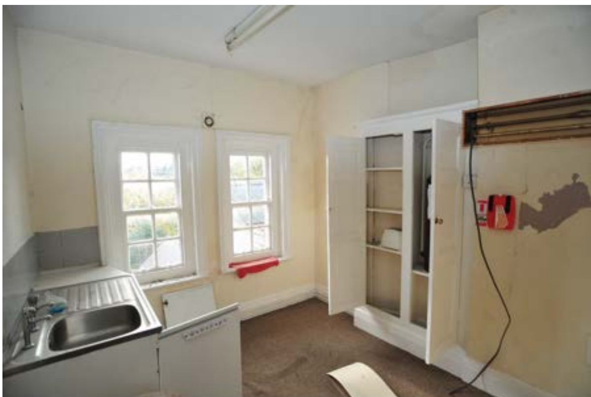
Pl.46: Original third-floor rear wing, looking south (1337).
