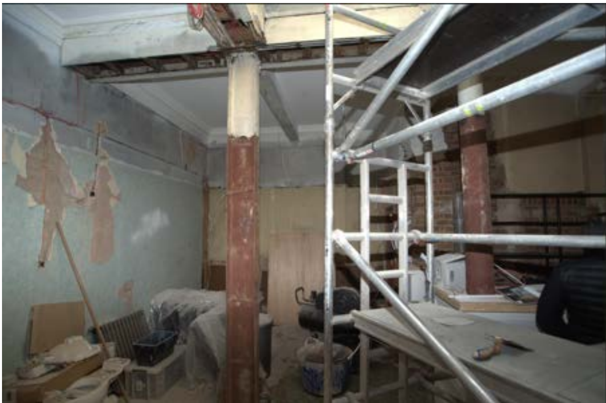
Pl.18: West internal wall of the rear portion of the frontage block (1379).
