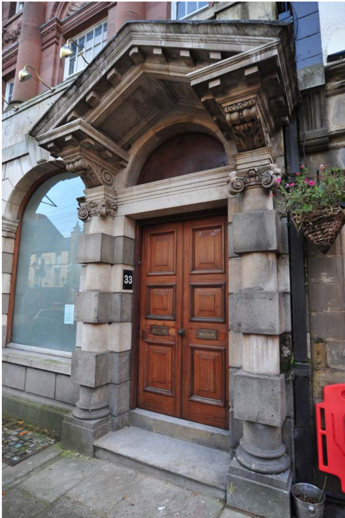
Pl.4: Detail of the main entrance to High Street (1313).
