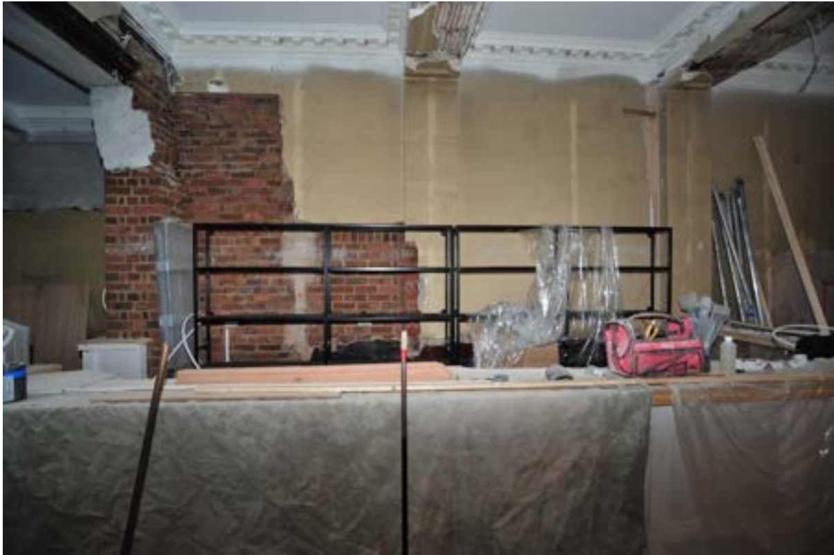
Pl.17: East internal wall of the southern end of the frontage range (1414).
