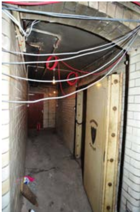
Pl.49: Northern corridor in the basement, looking east (1397).
