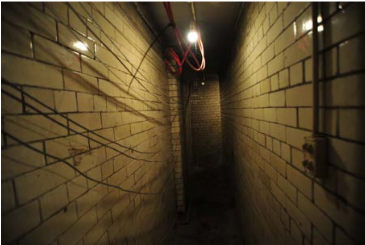
Pl.53: Southern corridor in the basement, looking west (1410).
