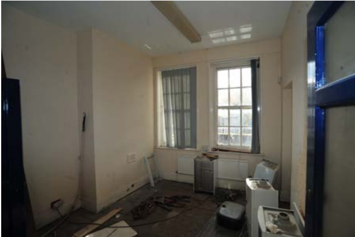
Pl.28: East rear first-floor room looking south (1361).
