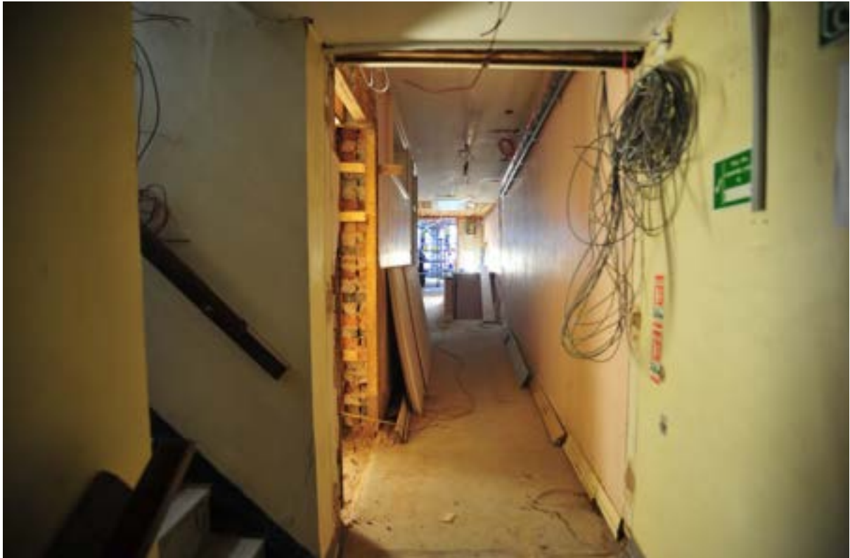
Pl.56: Rear corridor on the ground-floor looking north (1384).
