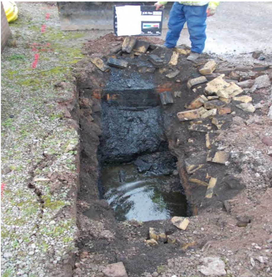
Plate 10: TP1 South of Garage (29-11-2013)
