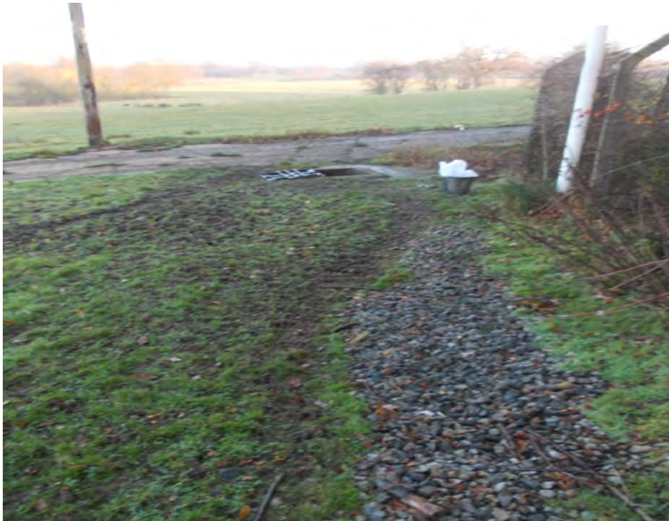
Plate 4: French Drain (SS11-07-1) NW Boundary – Looking North (10-12-2014).
